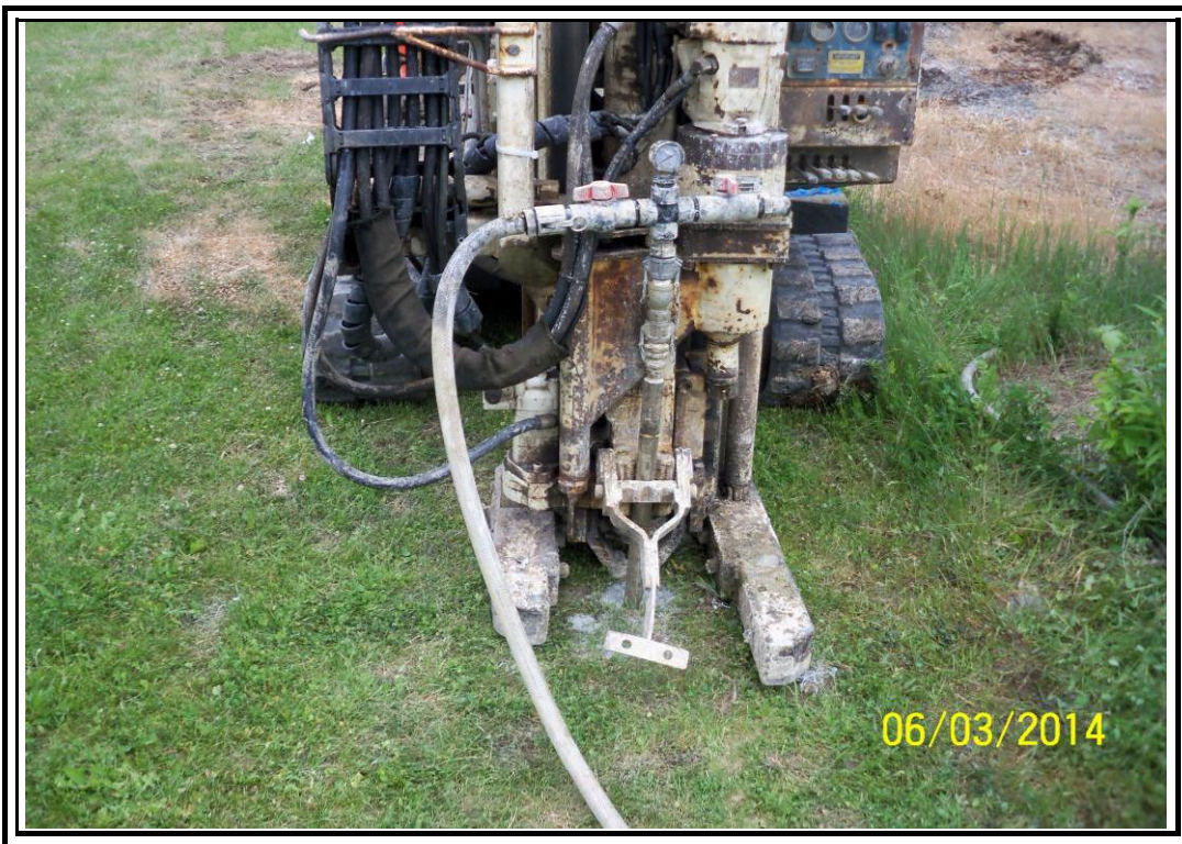
Photo 2 – View of typical PersulfOx™ injection setup, near the SUMP
