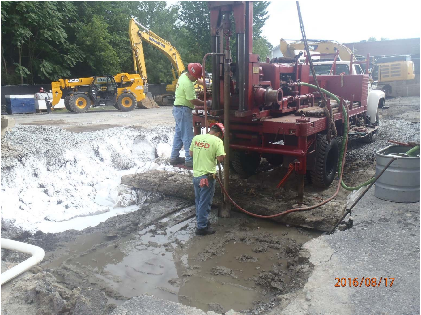
Start of ISS coring in pilot cell.
