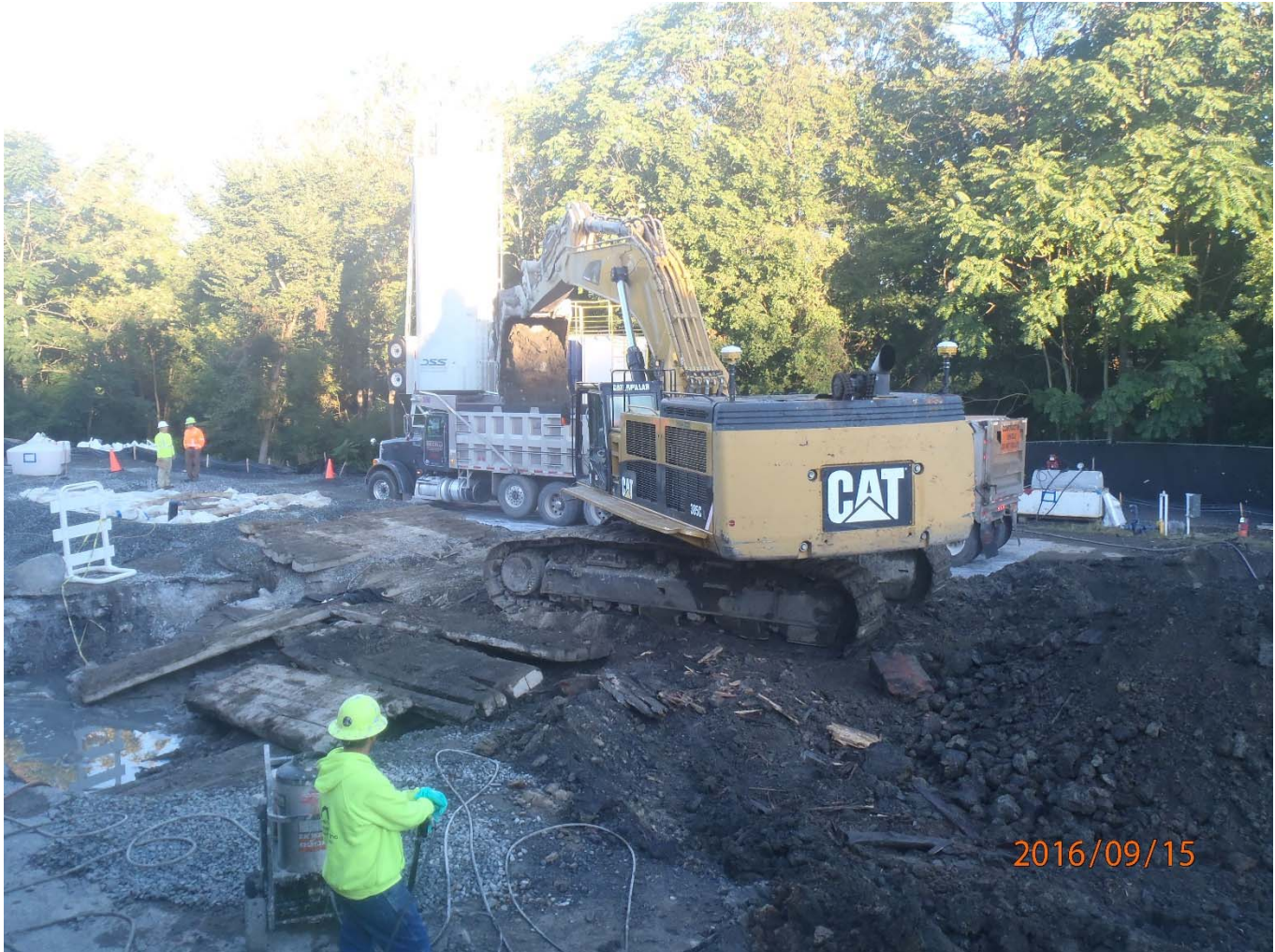
Loading out pre-cut soils.
