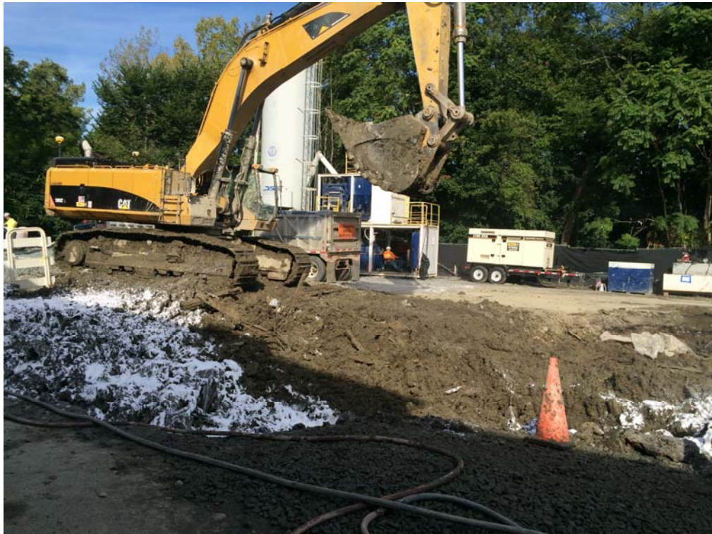
Photo 1: Loading soils into truck for off-site disposal
