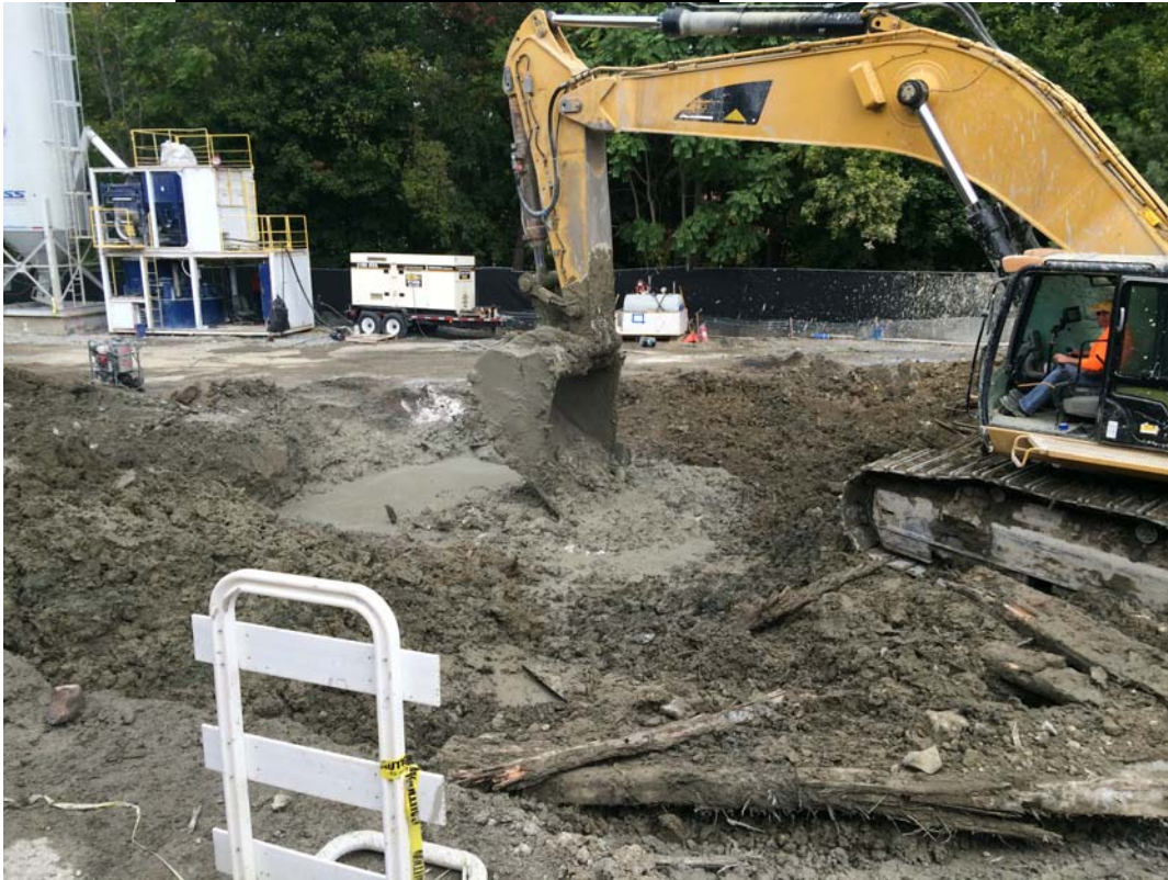
Mixing ISS swell with CKD for offsite disposal
