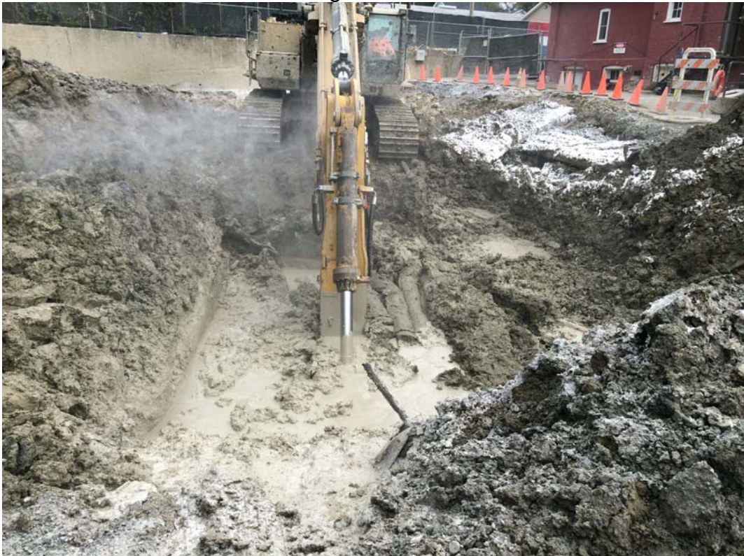
ISS Mixing on Cell 2K
