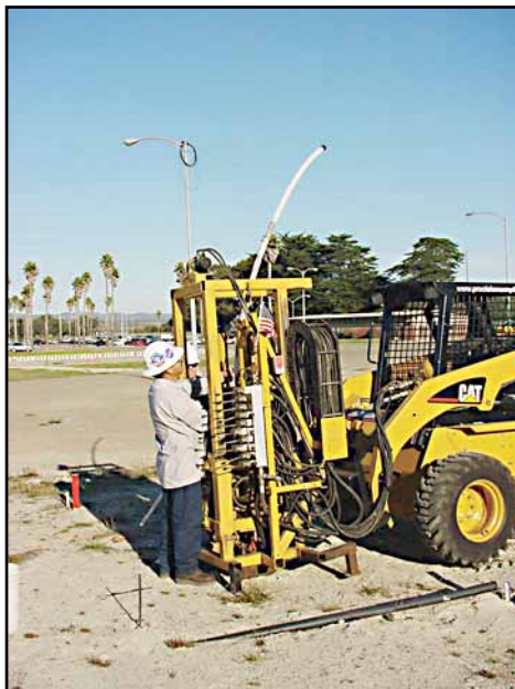
CMT System Being Installed Beside Direct Push Rig
