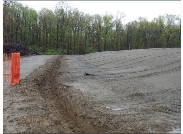
Photo No. 44: View of excavated anchor trench for top liner at Containment Cell
