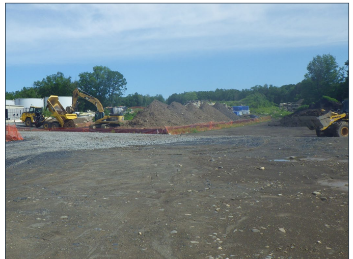
Photo No. 30: View of soil stabilization at relocated batch treatment area at north end of Eastern Fill Area
