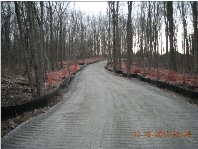
Photo No. 9: View of constructed temporary construction road
