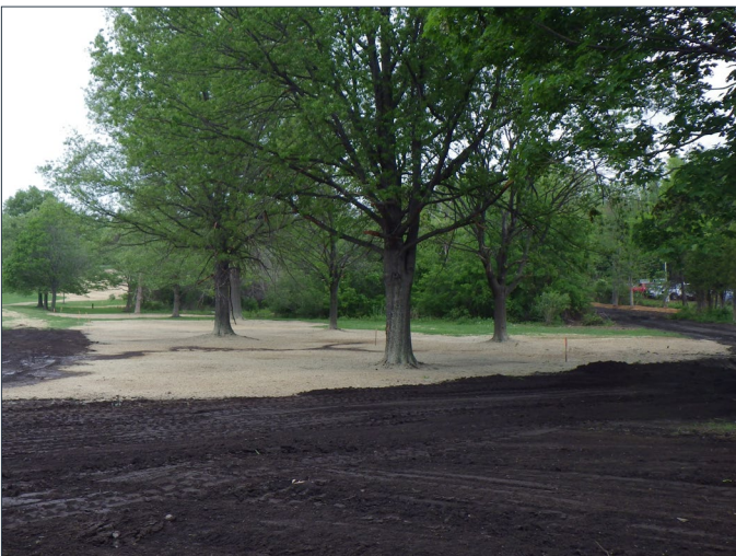
Photo No. 29: View of topsoil placement on excavated surface of Front Lawn Area
