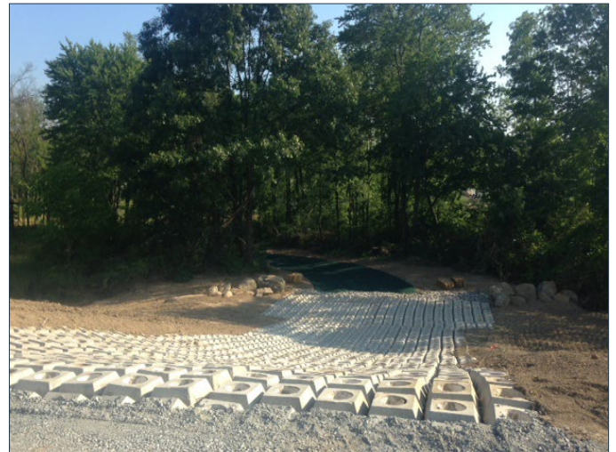
Photo No. 48: View of installed concrete block and vegetated swale spillway from Containment Cell
