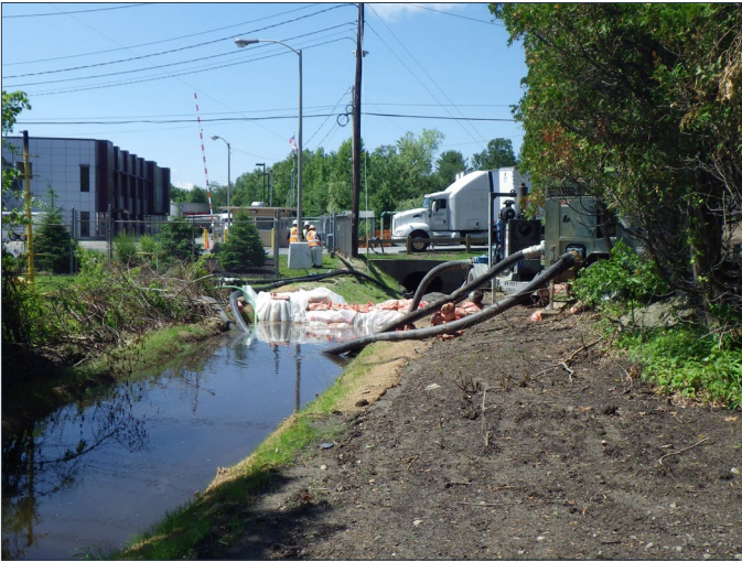
Photo No. 31: View of surface water bypass system for Western Stream south of facility driveway (Area 16B)
