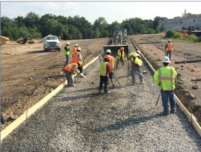
Photo No. 23: View of grading and installation of concrete road in Eastern Fill Area
