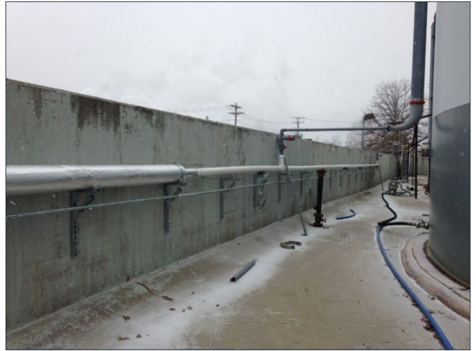
Photo No. 55: View of installation of permanent leachate conveyance piping at tanks
