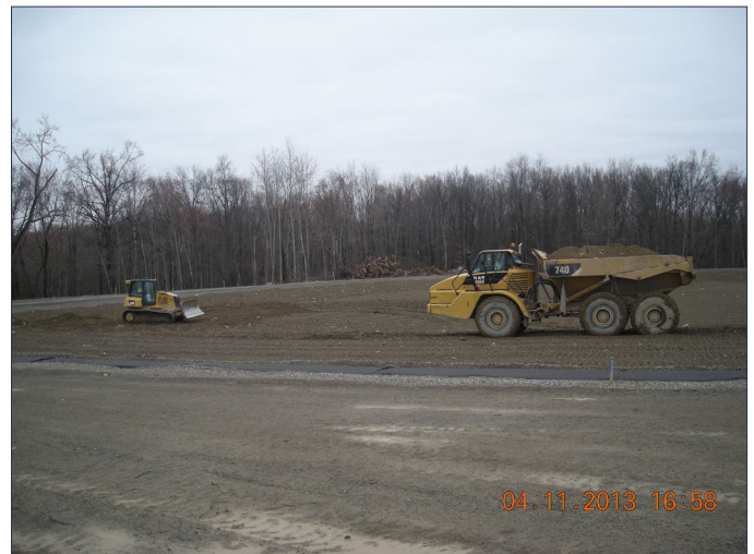
Photo No. 12: View of placement of stabilized soil in Containment Cell
