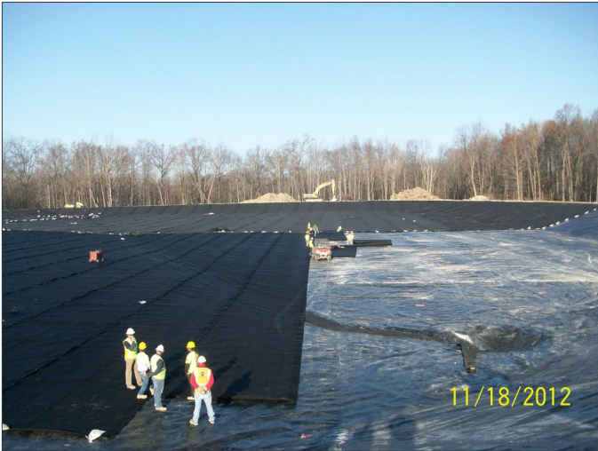
Photo No. 7: View of installation of composite drainage layer for bottom liner of Containment Cell
