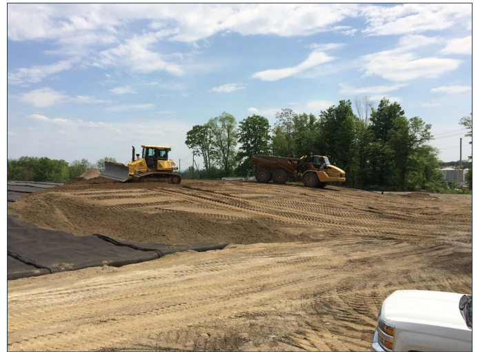
Photo No. 46: View of placement of protective cover soil on Containment Cell cap permanent section
