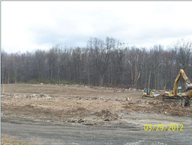
Photo No. 1: View of clearing and grading of Containment Cell footprint
