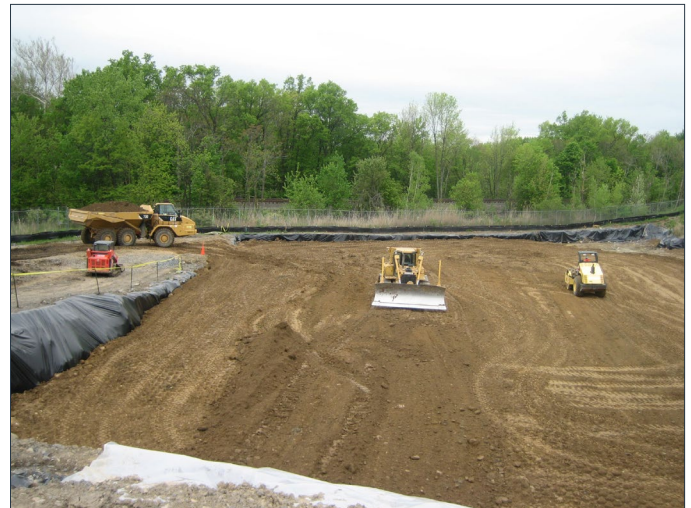
Photo No. 4: View of backfilling of water-filled excavation in Eastern Fill Area
