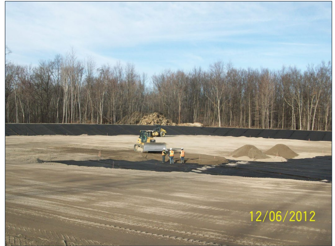
Photo No. 8: View of placement of protective soil layer on bottom liner of Containment Cell
