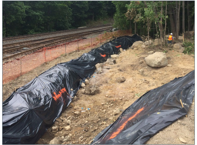
Photo No. 14: View of placement of demarcation liner in excavated Area 20
