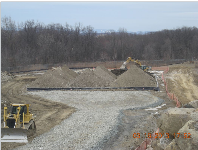
Photo No. 11: View of soil stabilization in batch treatment area
