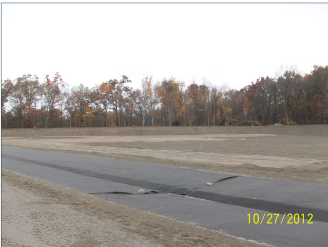
Photo No. 5: View of installation of bedding layer and groundwater underdrain for Containment Cell
