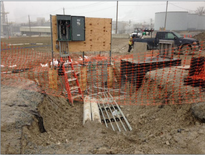
Photo No. 54: View of installation of permanent leachate conveyance system plumbing and electrical components at vault
