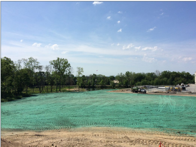
Photo No. 47: View of hydroseeded surface of Eastern Fill Area surface drainage area south of Containment Cell
