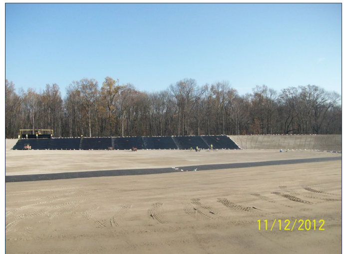
Photo No. 6: View of installation of HDPE geomembrane for bottom liner of Containment Cell
