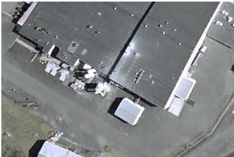
Aerial Photo, April 2001, showing equipment and structures in the building addition area.
