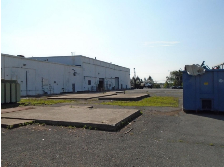
View facing southeast across the building addition area, with the drill rig working at boring B1.
