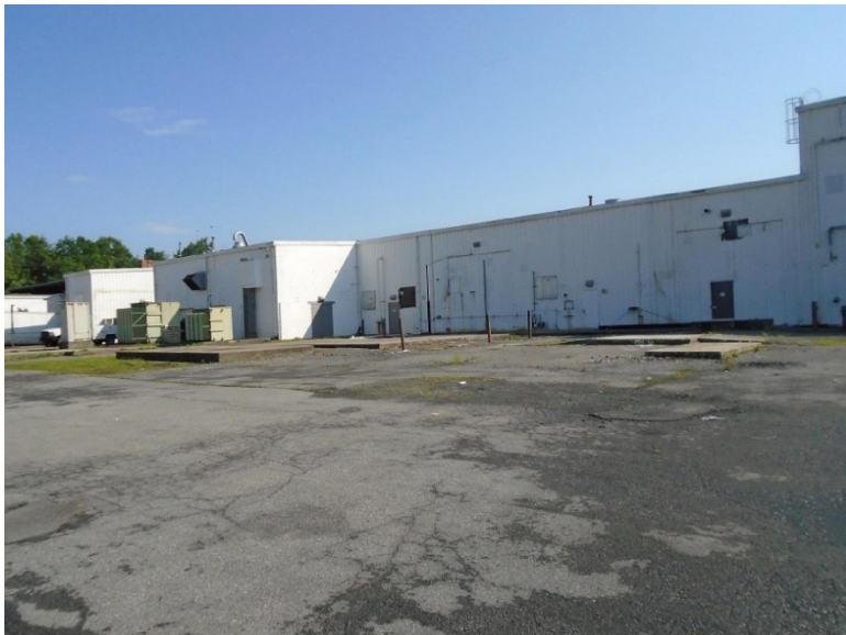
View facing northeast across the middle and rear of the building addition area.
