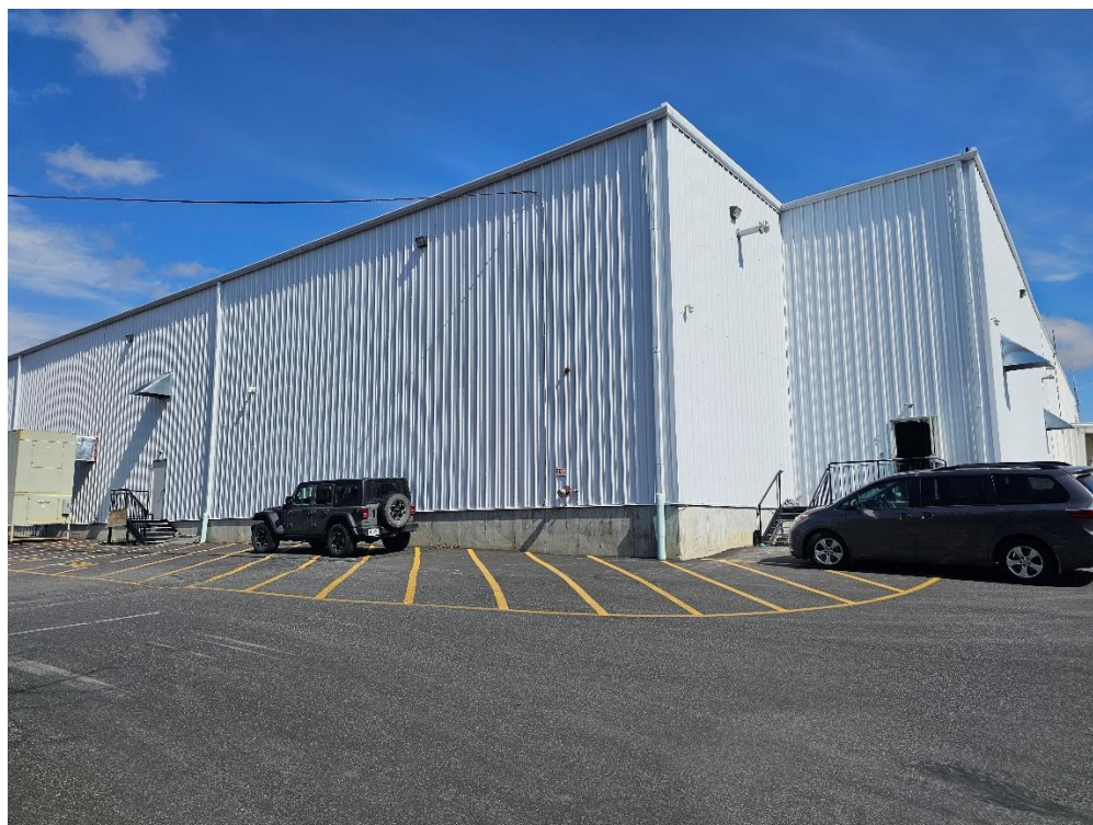
Photo No. D-2 – Addition facing east, note raised foundation. (03/20/2025)
