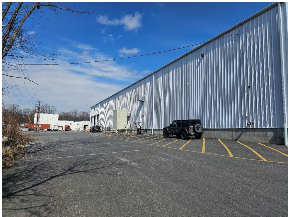
Photo No. D-1 – Addition facing northeast. (03/20/2025)
