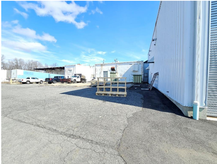
Photo No. D-3 – Northernmost wall of addition, facing east. (03/20/2025)
