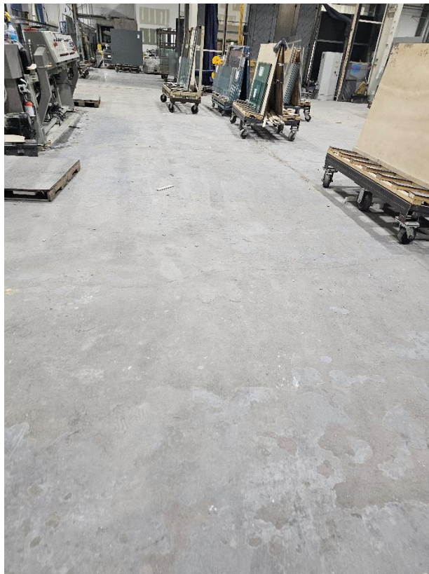
Photo No. D-4 – Slab in addition area, good condition. (03/20/2025)
