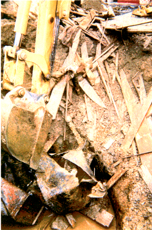
Excavation of Holding Tank. Note amount of wood and cloth contained within tank's interior.
