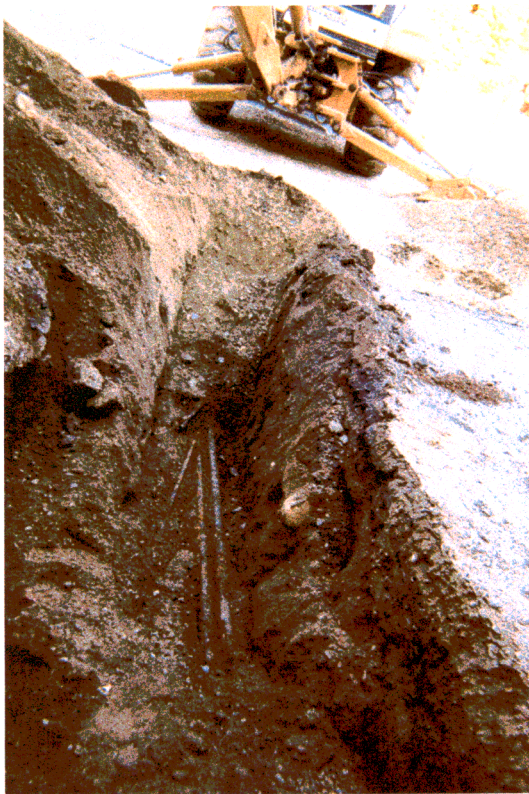
Excavation of piping from Holding Tank to building foundation. Pipes were not connected to anything within the building and were not observed to penetrate foundation walls.
