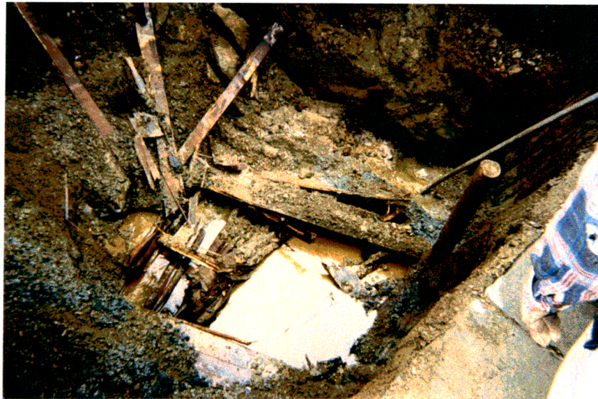
Excavation of Cylindrical Object (Holding Tank). Note wood from tank's interior and vertical pipe in right hand portion of Photograph
