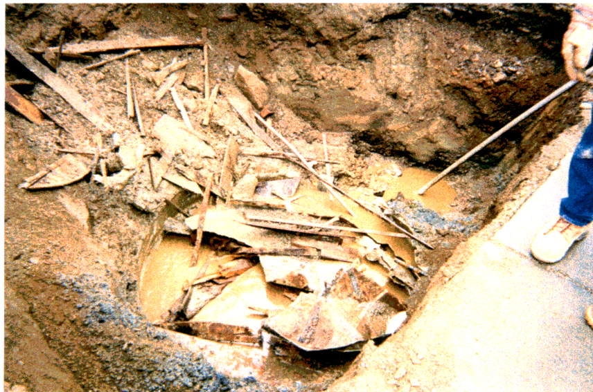
Excavation of Cylindrical Object (Holding Tank). Note wood from tank's interior. Tank contents pumped out and transported off-site for disposal (Bill-of-Lading appendix B)
