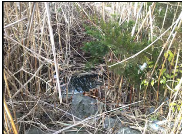
EXISTING CONDITIONS AT OUTFALL 010 NOT TO SCALE
