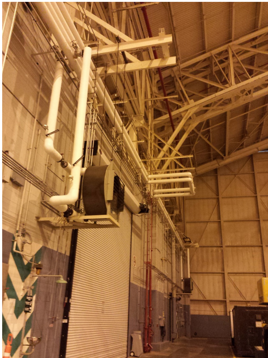
Photo 9: AFFF generators were formerly installed on the high beams in Hangar 100.
