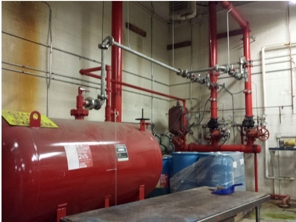
Photo 8: Boiler Room at Hangar 100, which currently is equipped with a HEF bladder tank (formerly equipped with AFFF bladder tanks).
