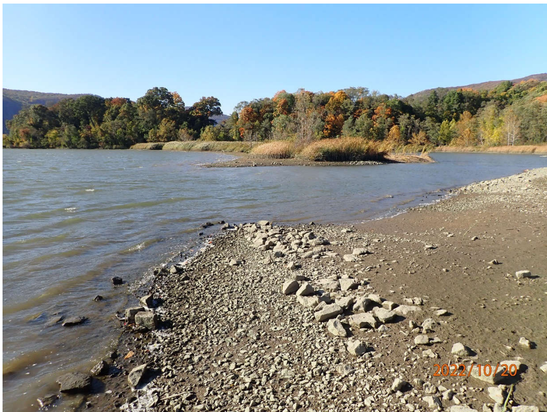
Photo 14 – photo location D5 – Looking west.
