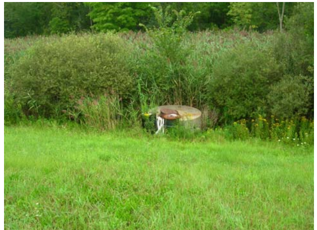
The Leachate Sump on the east side of the landfill
