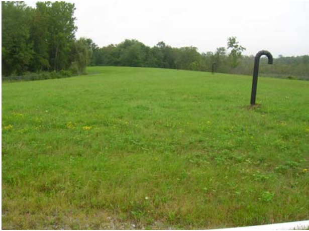
Looking north along the top of the landfill from the gravel roadway
