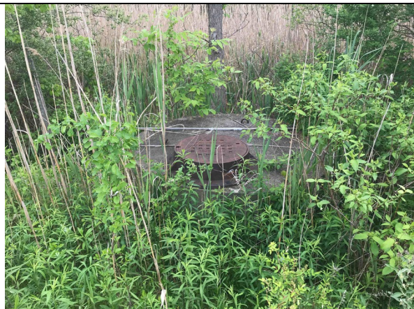
Photo 2: View of the Leachate Collection System Sump Manhole
