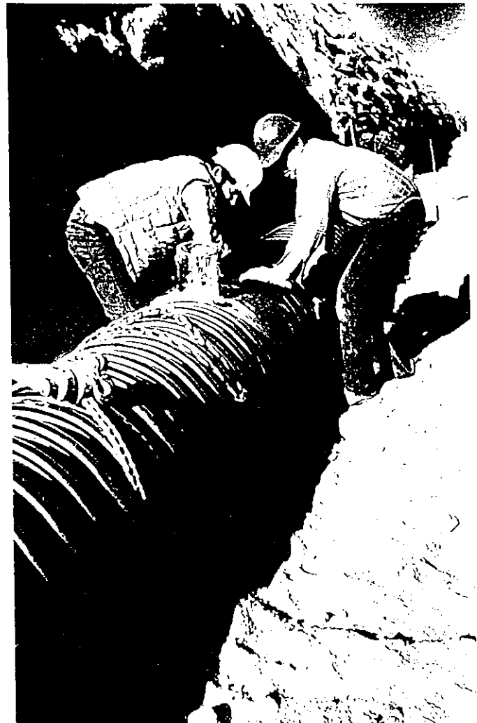
Assembling a Spirolite® joint
