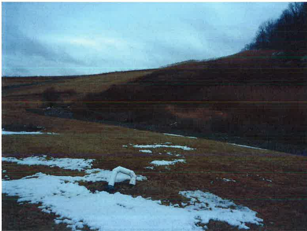
Photograph 8: Down vent near the eastern bend of the Landfill.
