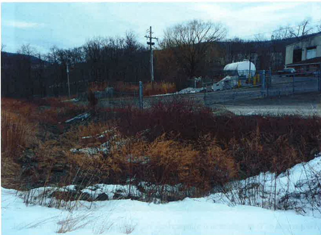
Photograph 2: Overgrown drainage on the most eastern border of Landfill and directly northwest of Baler Building.
