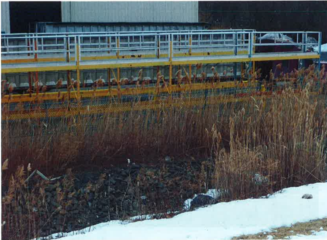
Photograph 1: Overgrown drainage across from Baler Building.
