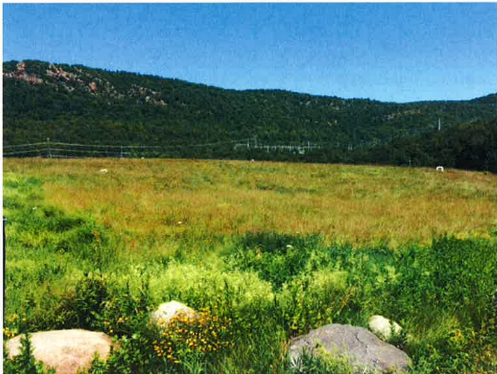
Photograph 4: Landfill cover has suitable vegetation and no evidence of erosion was observed (southeast to northwest).
