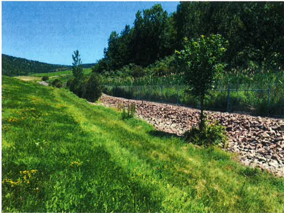
Photograph 13: Occasional saplings and slightly overgrown vegetation present in the drainage channel on the southeastern portion of the Landfill (southwest to northeast).
