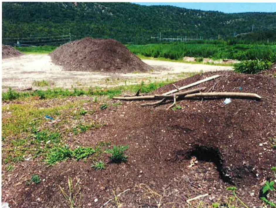
Photograph 16: Six (6) inch diameter inactive vector burrow located east of the compost windrows on the northeastern portion of the Landfill (southeast to northwest).
