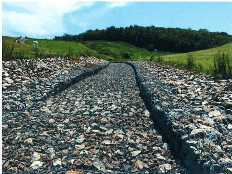
Photograph 10: Center drainage channel is in good condition located on the central portion of the Landfill (northwest to southeast).
