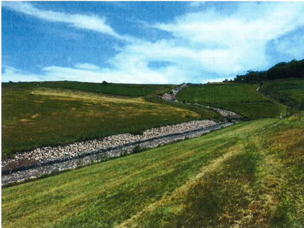
Photograph 11: View of central drainage structures with no signs of erosion (west to east).
