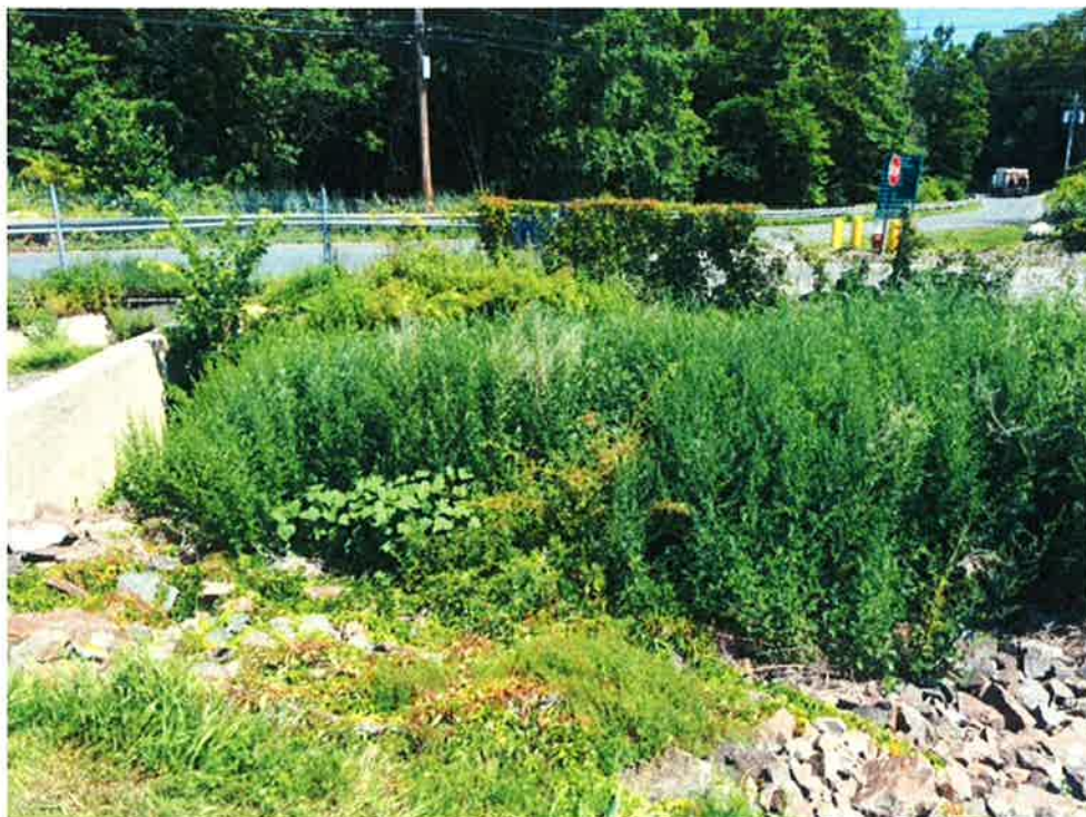
Photograph 8: Overgrown vegetation present within the drainage swale on the northernmost edge of the Landfill (south to north).
