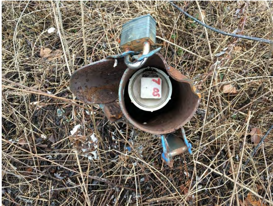
Photograph 23: Top view of damaged monitoring well 7-OS.
