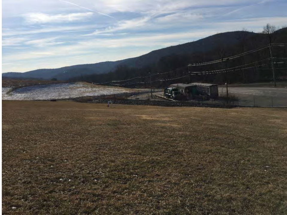
Photograph 9: View of scalehouse along the western portion of the Landfill (east to west).
