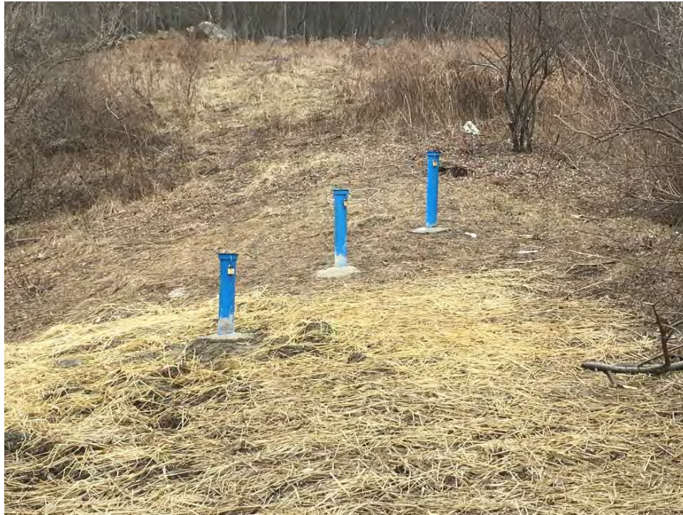
Photograph 1: View of newly installed upgradient monitoring well cluster – UP-OS, UP-I, and UP-R (northwest to southeast).
