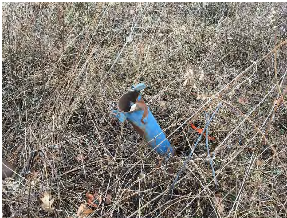
Photograph 22: Monitoring well 7-OS is damaged approximately three (3) feet below the top of the outer steel protective casing (southwest to northeast).
