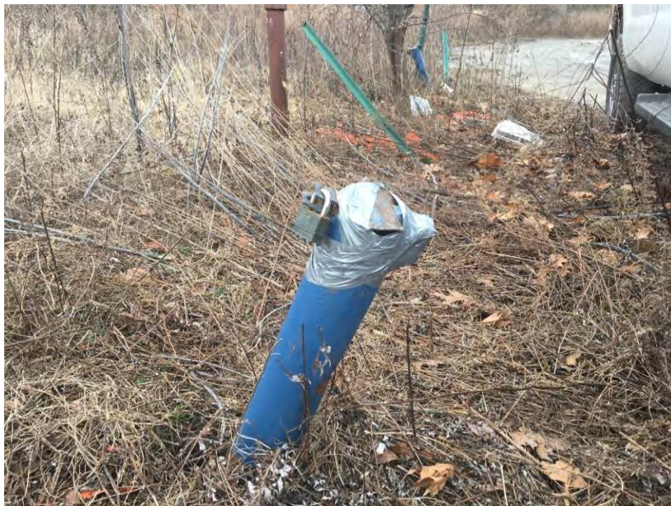
Photograph 24: Monitoring well 7-OS was wrapped with duct tape to temporarily keep the internal portion of the monitoring well secure (north to south).
