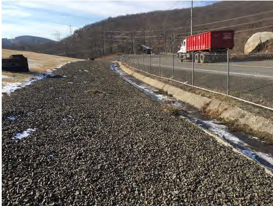
Photograph 7: Perimeter drainage ditch along the northern portion of the Landfill is in good condition and operating as designed (east to west).
