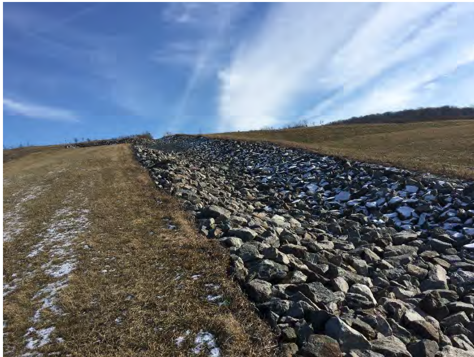
Photograph 8: Drainage structure Downchute 3 is in good condition and operating as designed (northwest to southeast).
