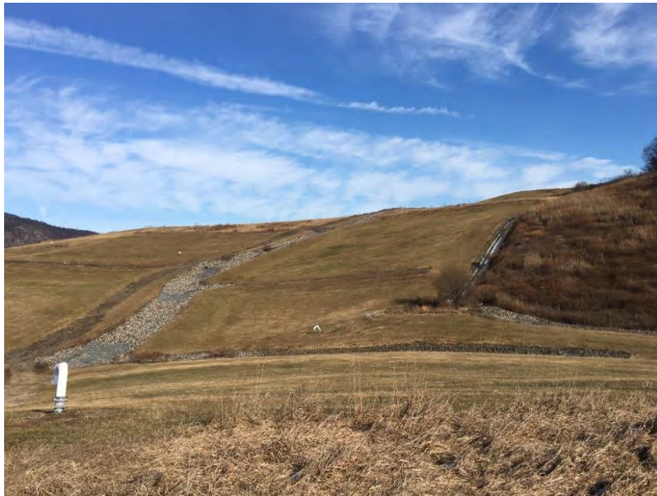
Photograph 14: View of southern portion of Landfill (southwest to northeast).
