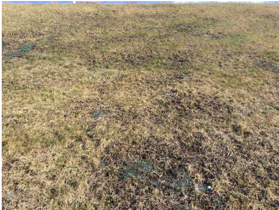
Photograph 10: Lightly vegetated Landfill cover was observed along southwestern sideslope of the Landfill (west to east).
