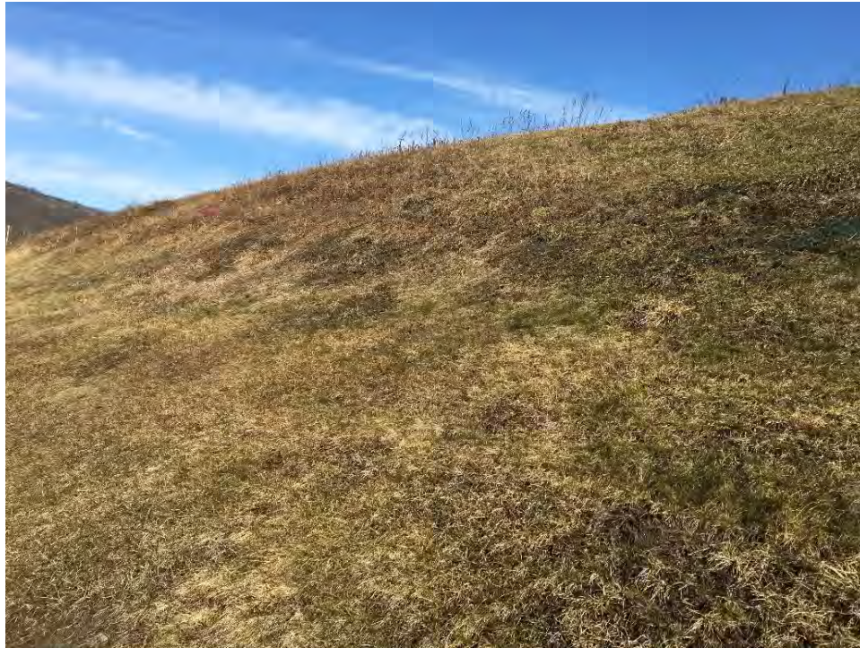
Photograph 11: Another view of the minor stressed vegetation due to erosion observed along the southwestern side slope of the Landfill (south to north).
