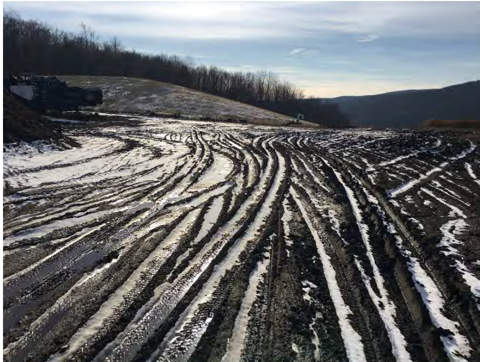
Photograph 19: Ruts observed on the access road to the compost piles. Landfill cover is not compromised (northeast to southwest).
