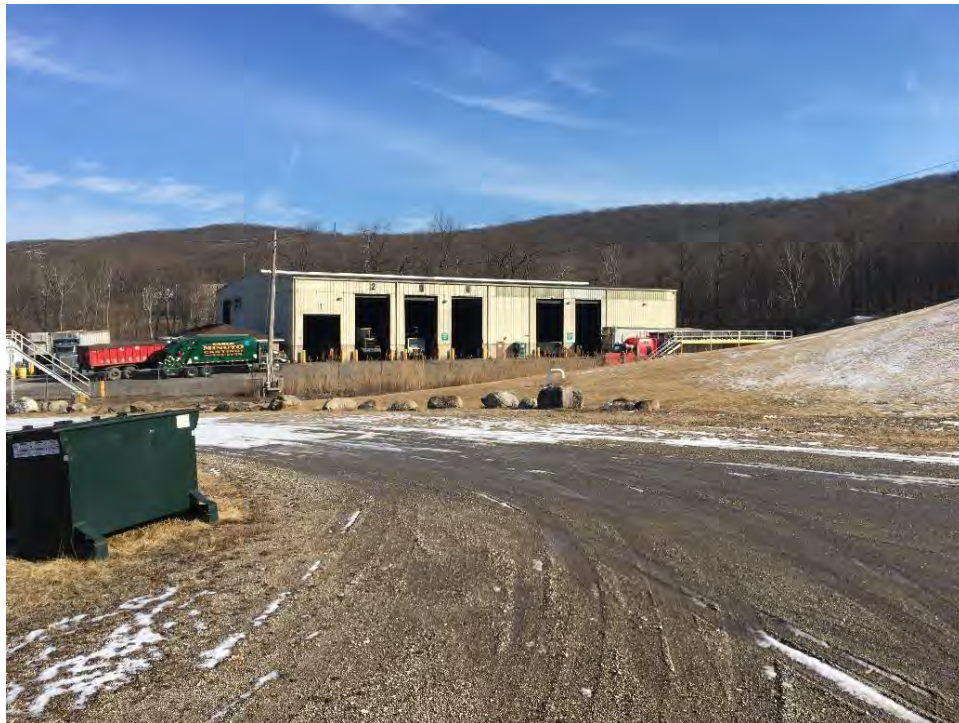
Photograph 2: View of the Baler Building from Landfill west of upper Landfill gate (west to east).
