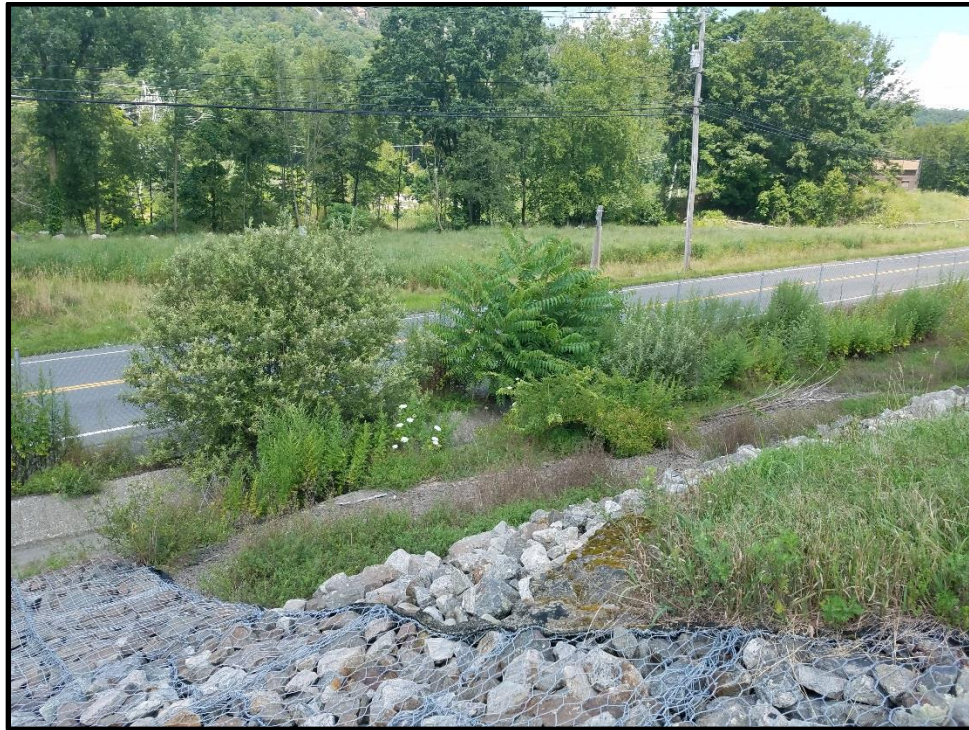
Photograph 1714: View of northwestern perimeter of the Landfill, looking north.
