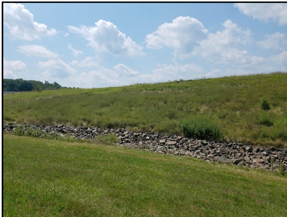
Photograph 2017: View of northern portion of Landfill, looking west-southwest
