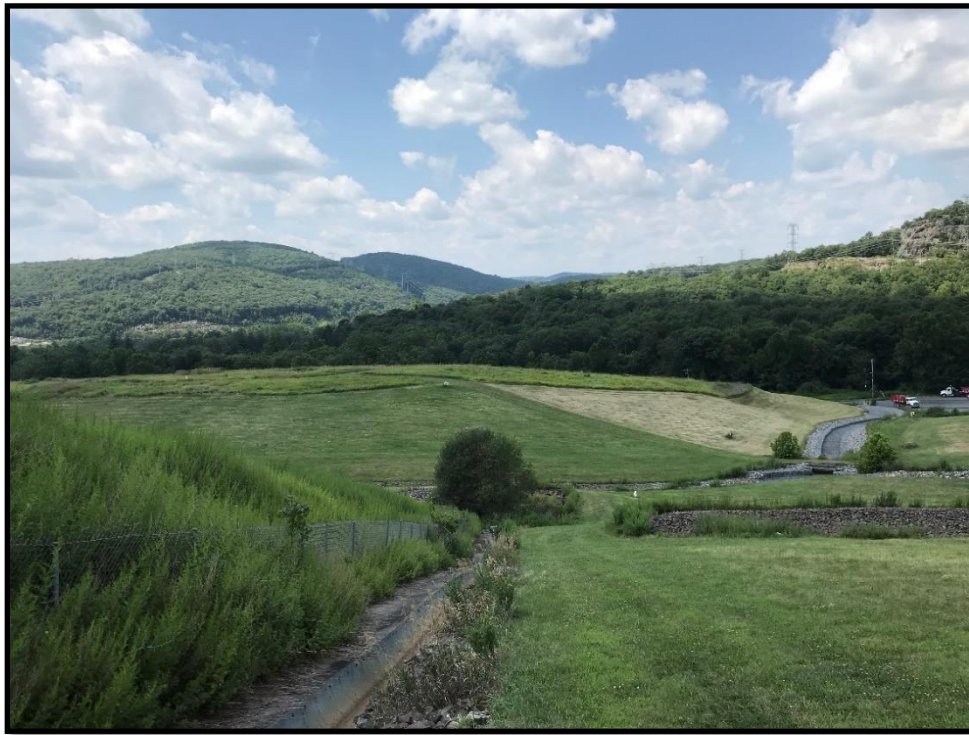
Photograph 7: View of central portion of Landfill cover and drainage system, looking west.
