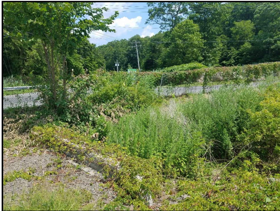
Photograph 1815: View of northernmost portion of the Landfill with vegetation grown in the drainage channel, looking northeast.
