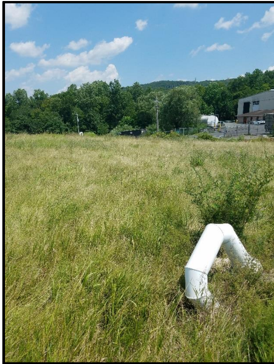
Photograph 2118: View of northern portion of Landfill with bent gas vent and baler building, looking northeast.
