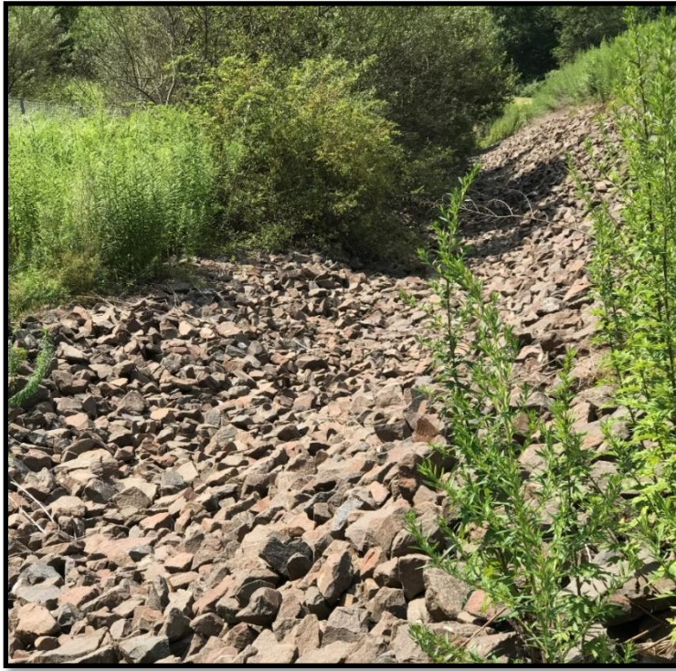
Photograph 1: View of Drainage Channel 2 along northeastern border of the Landfill facing southeast.
