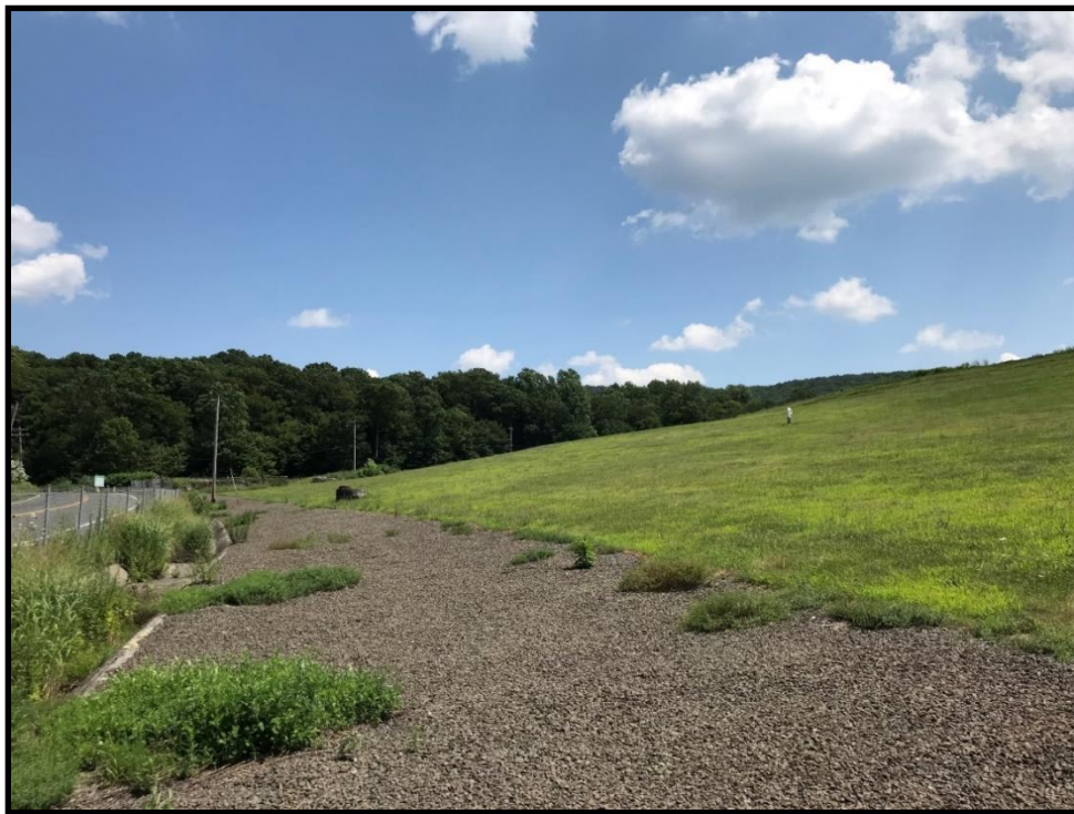
Photograph 1613: View of northwestern perimeter of the Landfill, looking east-northeast.
