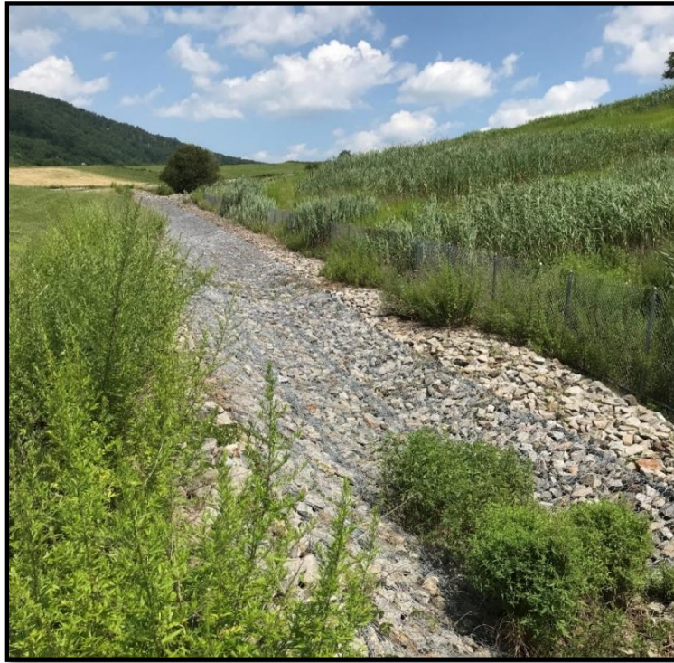
Photograph 7: View of southeastern Landfill drainage channel with vegetation growth, looking north.
