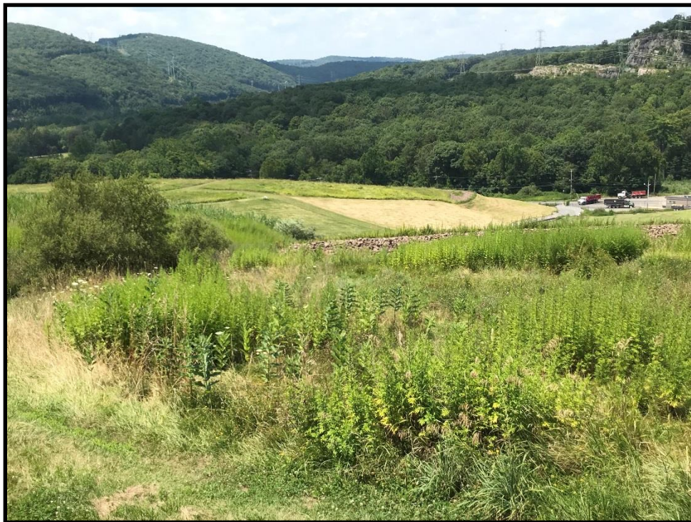
Photograph 6: View of southern border of the Landfill, looking west.
