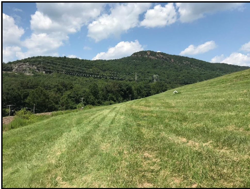
Photograph 10: View of southwestern portion of the Landfill, looking north.
