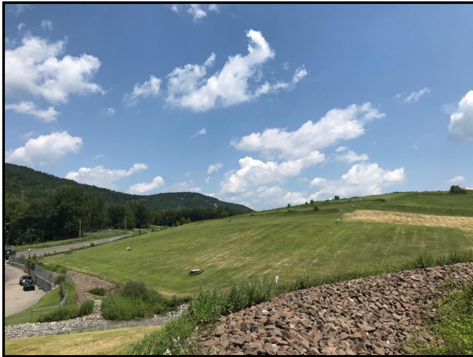
Photograph 14: View of central portion of the Landfill, looking northeast.
