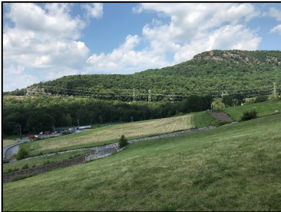
Photograph 8: View of southwestern portion of the Landfill cover and drainage system, looking northwest.
