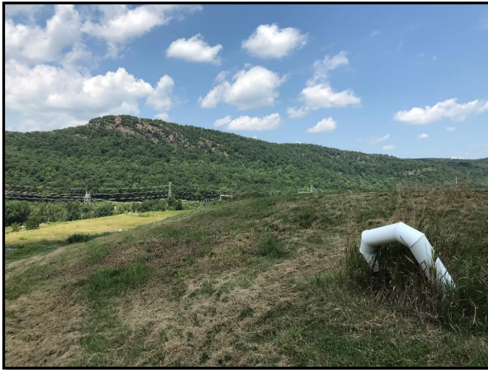
Photograph 5: View angled gas vent with overgrown vegetation along southeastern face of the Landfill, looking northwest.
