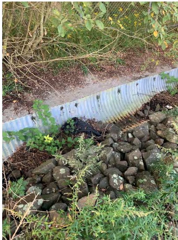
Photograph 1612: View of debris build-up in drainage swale along the mideastern perimeter of the Landfill, looking southeast.
