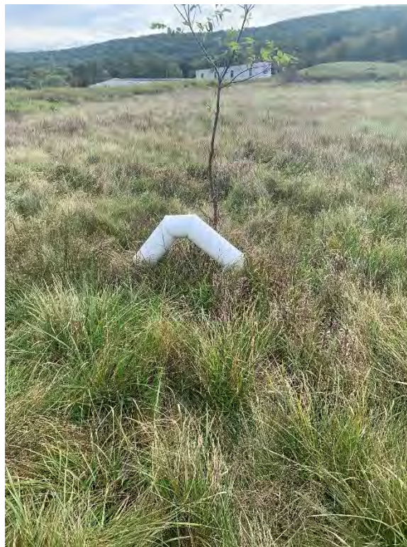
Photograph 3: View of leaning gas vent in the north central portion of the Landfill, looking southeast.
