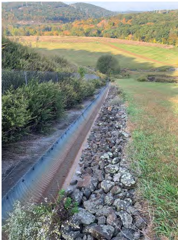
Photograph 14: View of well-maintained drainage chute along the mideastern perimeter of the Landfill, looking west-southwest.
