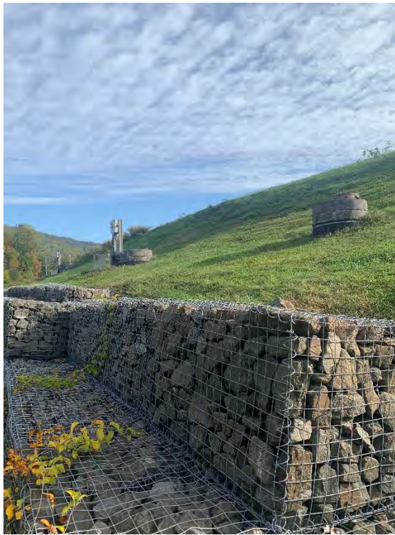
Photograph 1915: View of well-maintained gabion retaining walls along the southwestern perimeter of the Landfill, looking north.
