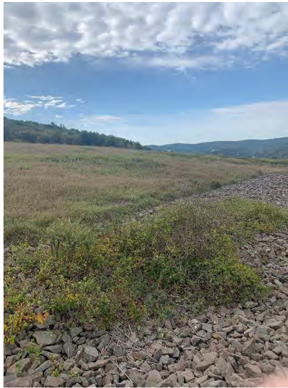
Photograph 2: View of well-established cover system and minor overgrown vegetation in drainage feature in the northern portion of the Landfill, looking southwest.
