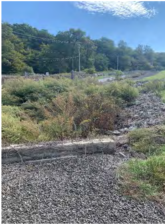
Photograph 1: View of slightly overgrown vegetation in the drainage channel along the northern perimeter of the Landfill, looking east-southeast.
