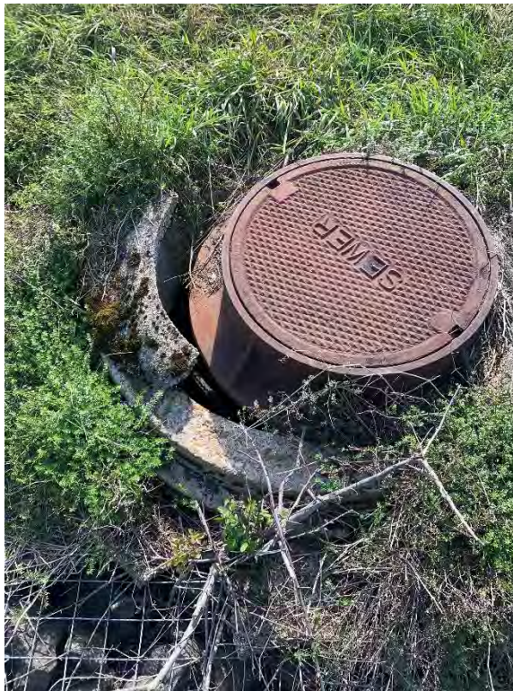
Photograph 1: View of damaged upper portion of the concrete drainage vault (MH E-6) near the northern perimeter of the Landfill, looking southeast.
