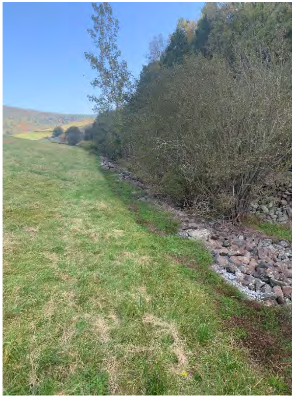
Photograph 2117: View of overgrown vegetation in drainage swale along the southeastern perimeter of the Landfill, looking north-northeast.
