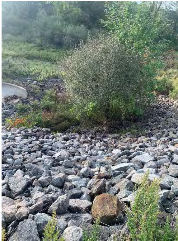
Photograph 10: View of overgrown vegetation in drainage feature along mideastern perimeter of the Landfill, looking east-northeast.
