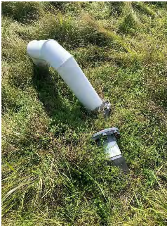
Photograph 8: View of damaged gas vent near the mideastern perimeter of the Landfill, looking southwest.
