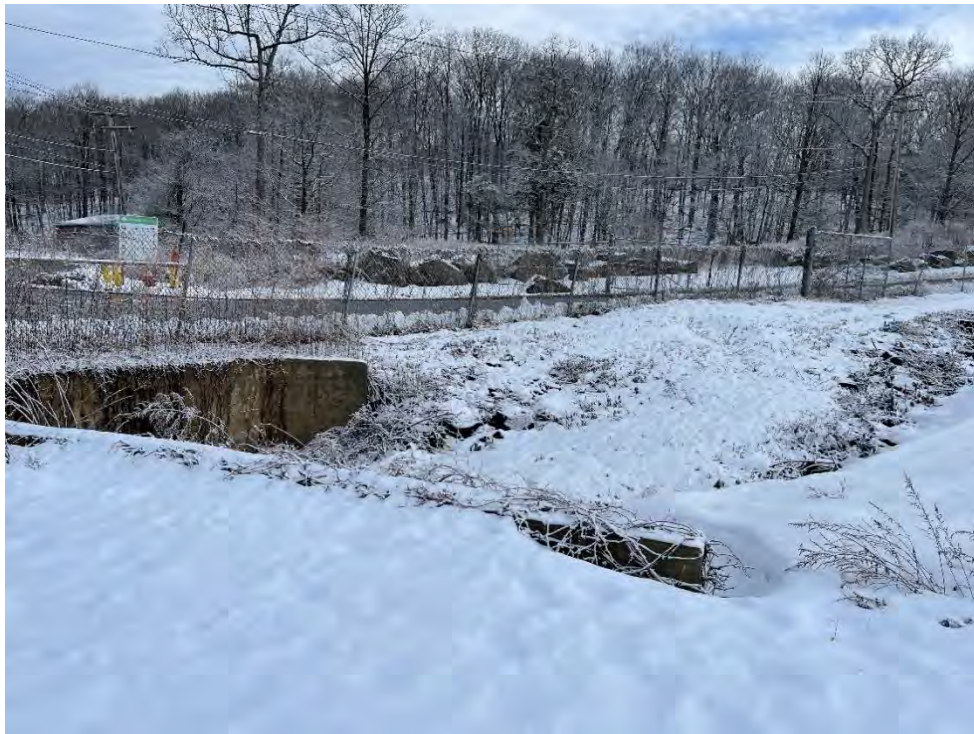
Photograph 1: View of drainage channel along the northern perimeter of the Landfill, looking east-southeast.
