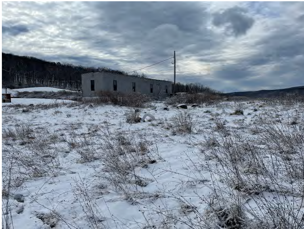
Photograph 5: View of leaning gas vent to the north of the firearms training building, looking south.
