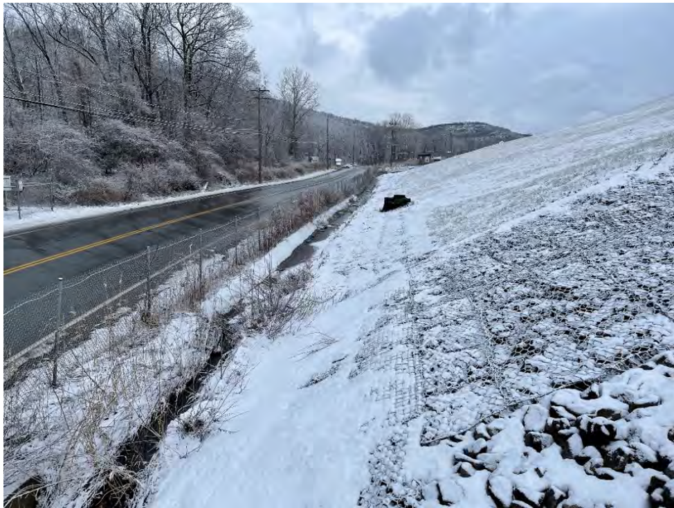
Photograph 11: View of drainage ditch along the southwestern perimeter of the Landfill, looking north-northeast.
