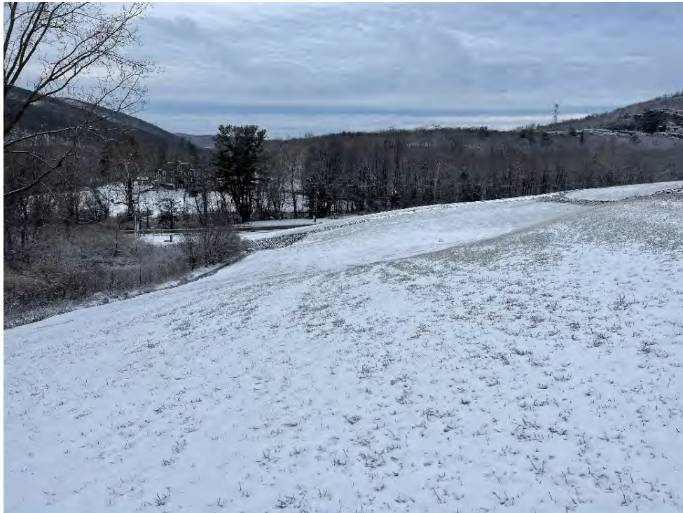
Photograph 22: View of well-maintained cover system along the southern perimeter of the Landfill, looking west-northwest.
