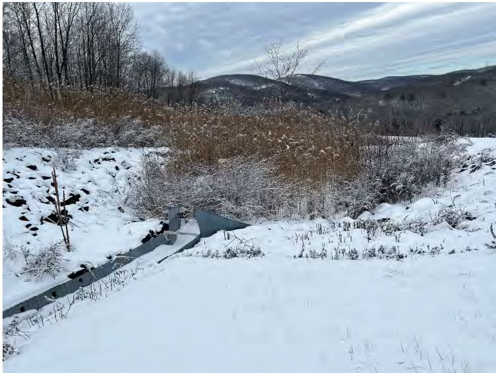
Photograph 13: View of slightly overgrown vegetation in drainage feature along the mid-eastern perimeter of the Landfill, looking west.
