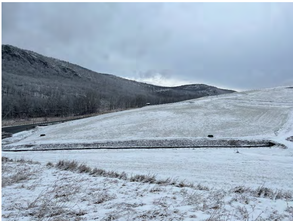
Photograph 12: View of well-maintained cover system in the central portion of the Landfill, looking northeast.
