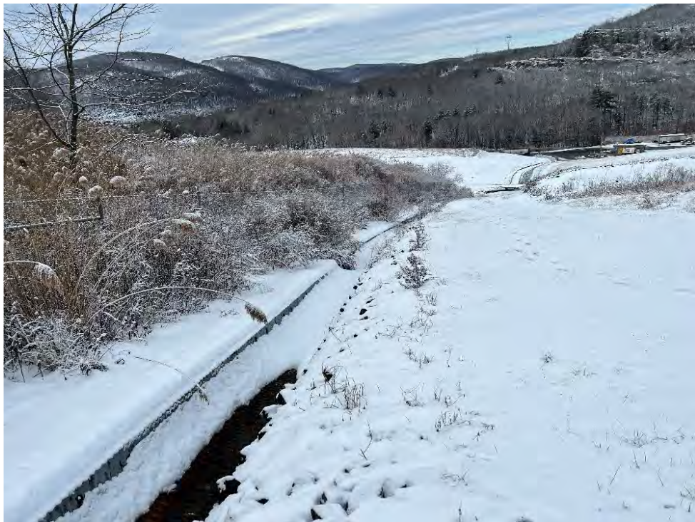
Photograph 14: View of well-maintained drainage chute along the mid-eastern perimeter of the Landfill, looking west.
