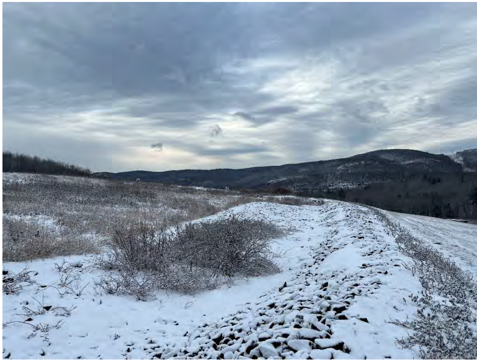
Photograph 3: View of well-established cover system and minor overgrown vegetation in drainage feature in the northern portion of the Landfill, looking southwest.
