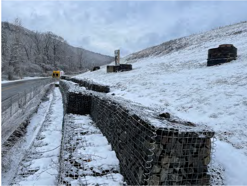
Photograph 17: View of well-maintained gabion retaining walls along the southwestern perimeter of the Landfill, looking north.
