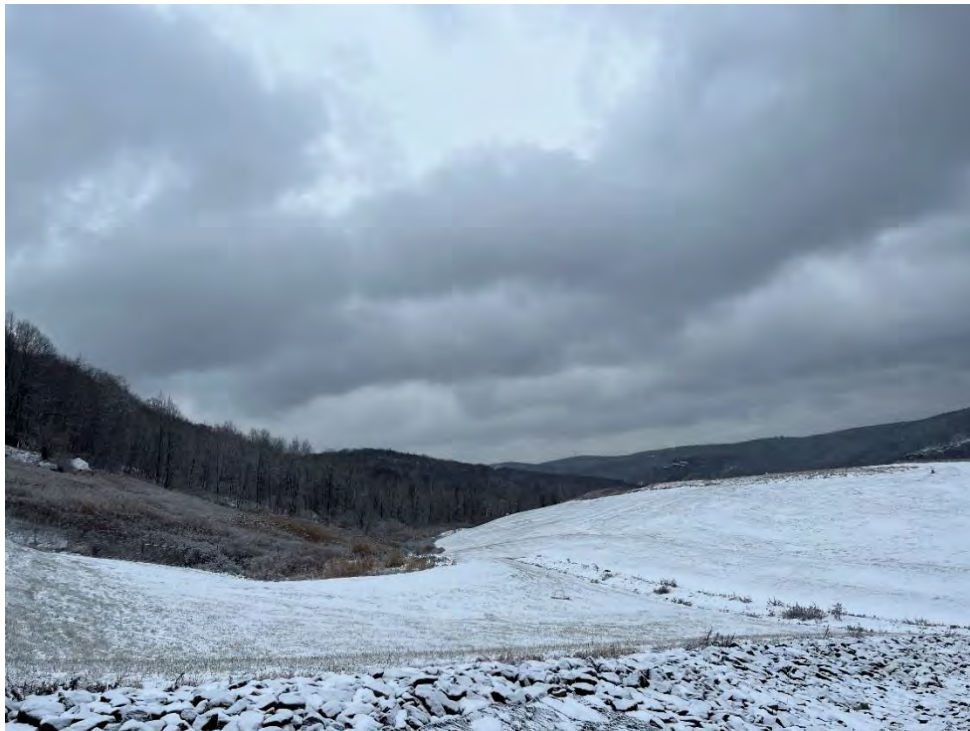
Photograph 10: View of well-maintained cover system along the southeastern perimeter of the Landfill, looking southwest.
