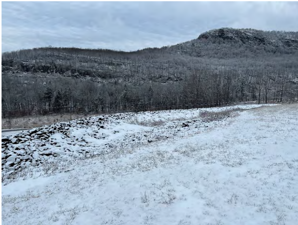
Photograph 7: View of drainage feature in east-central portion of the Landfill, looking northwest.
