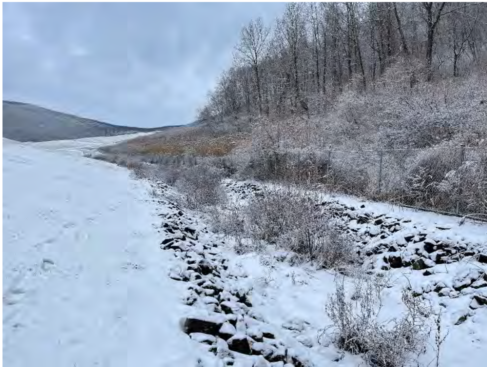
Photograph 19: View of slightly overgrown vegetation in drainage swale along the southeastern perimeter of the Landfill, looking north-northeast.
