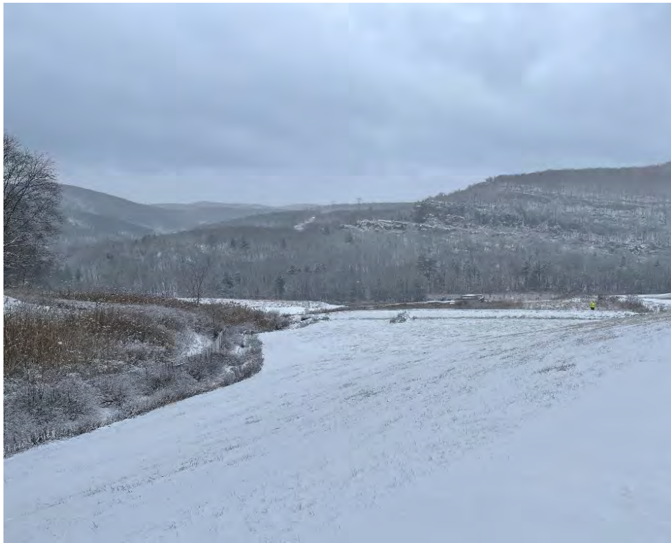
Photograph 15: View of well-maintained cover system along the mideastern perimeter of the Landfill, looking west.
