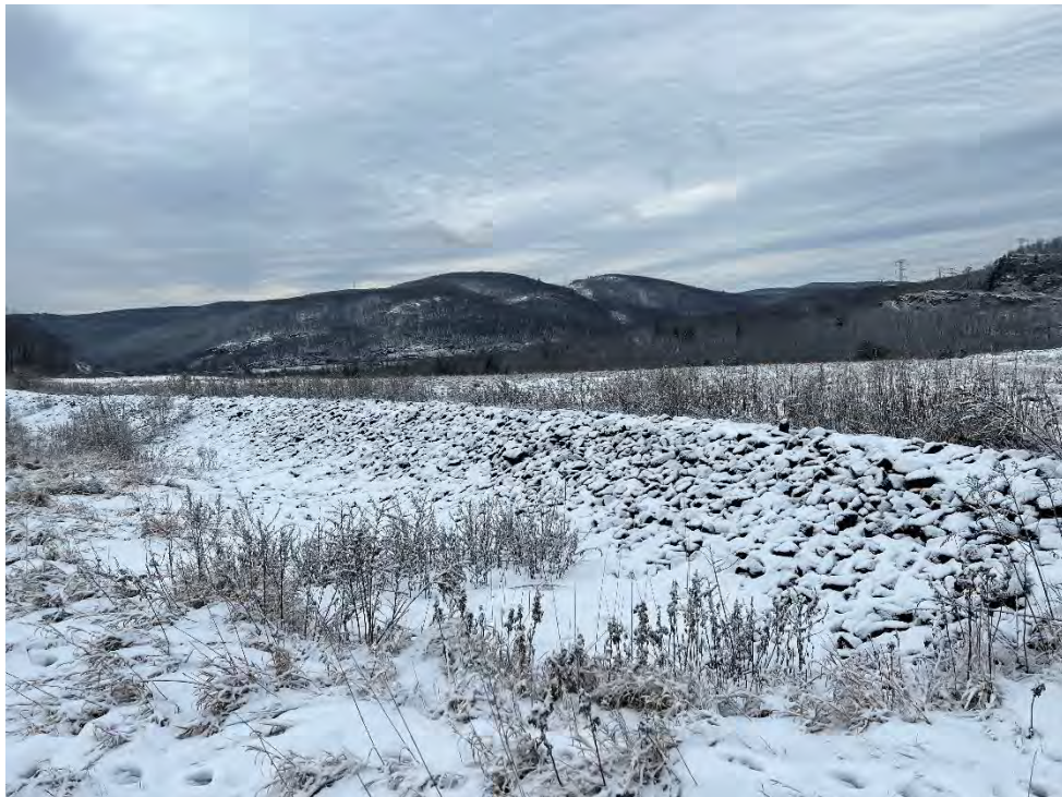
Photograph 8: View of slightly overgrown vegetation in drainage feature in west-central portion of the Landfill, looking southwest.
