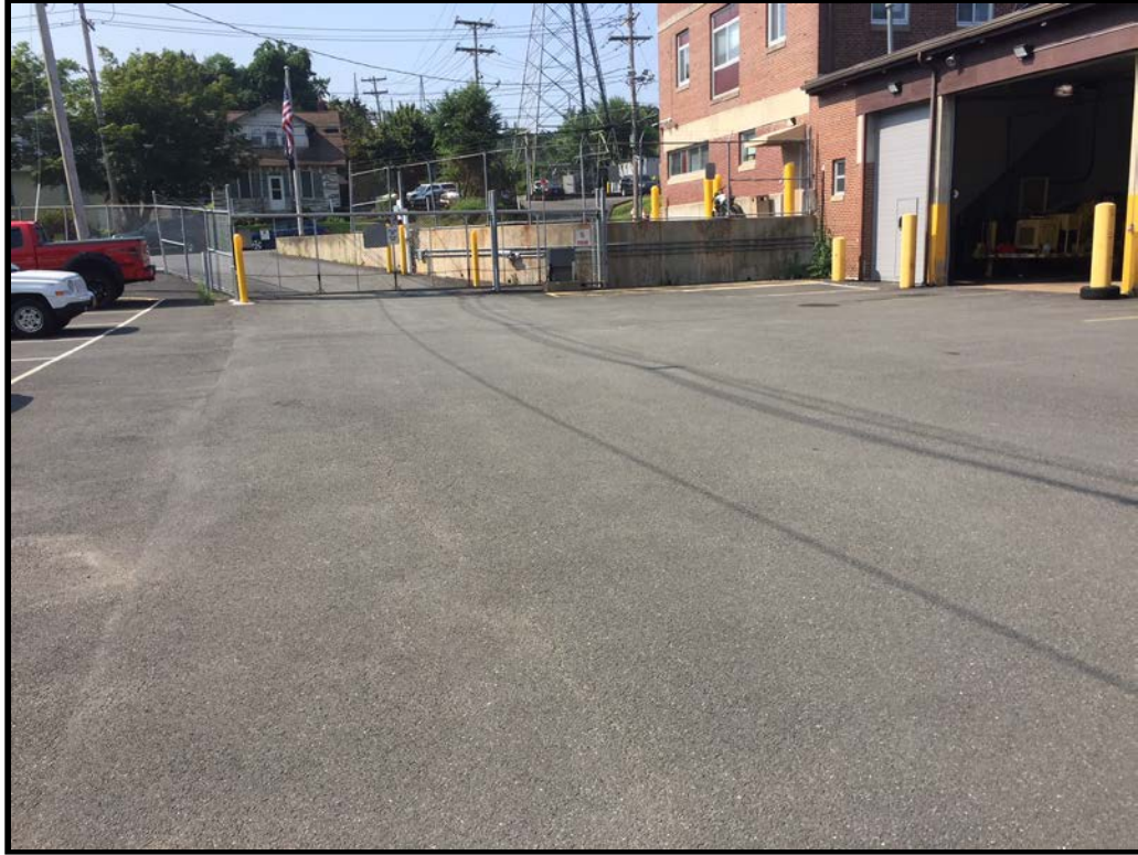
PHOTOGRAPH 1 New Pavement –Looking South, East of NYOC Building
