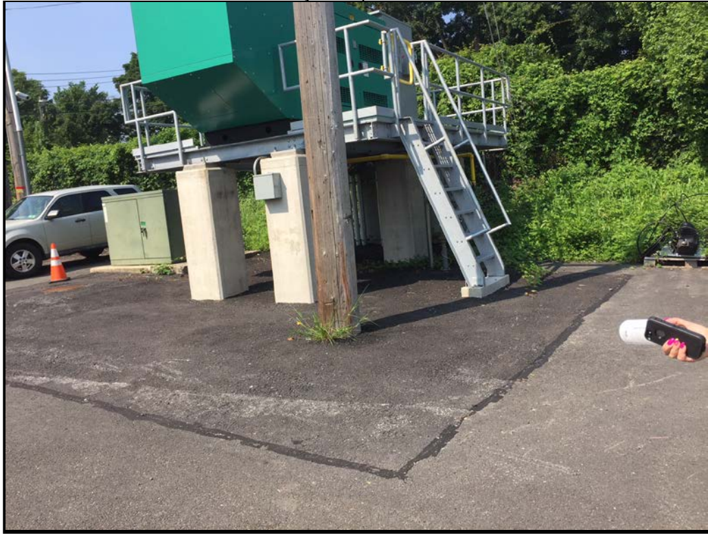
PHOTOGRAPH 7 New Emergency Generator Pavement Patch – Southwest side of Building
