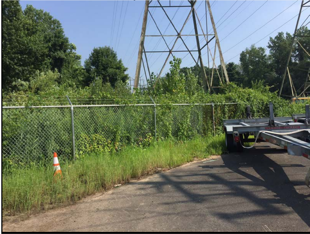
PHOTOGRAPH 5 New Fence Installed Along North Western Fence Line
