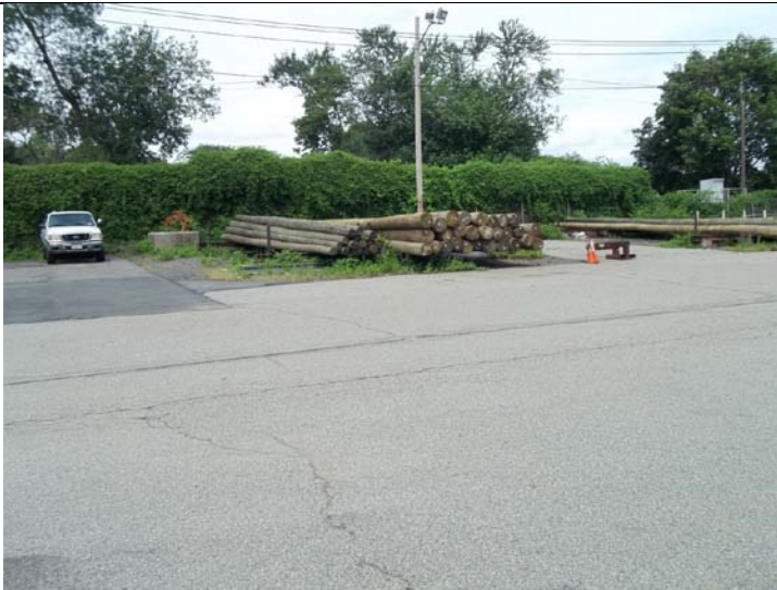
Area beneath the pole racks is not capped
