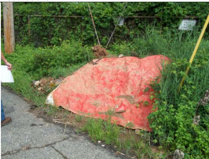
Tarp covered pile of dirt and construction debris
