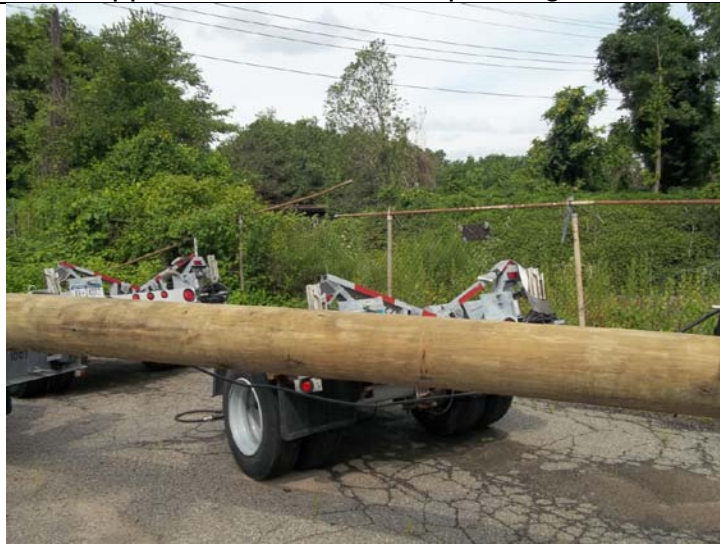
Top railing is broken
