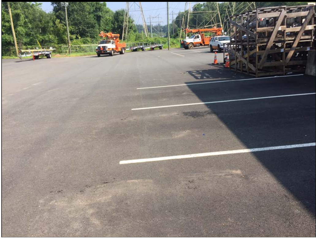
PHOTOGRAPH 3 New Pavement – West of Building Looking North
