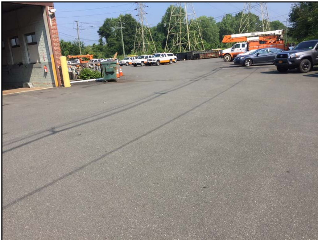
PHOTOGRAPH 2 New Pavement –Looking North, East of NYOC Building
