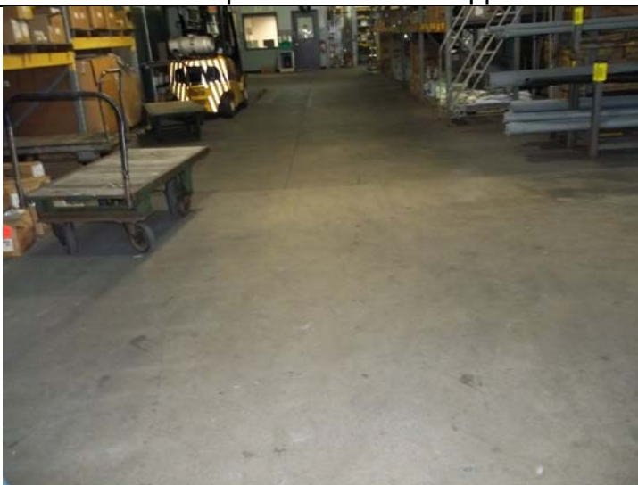
Floor slabs within the building appear to be intact
