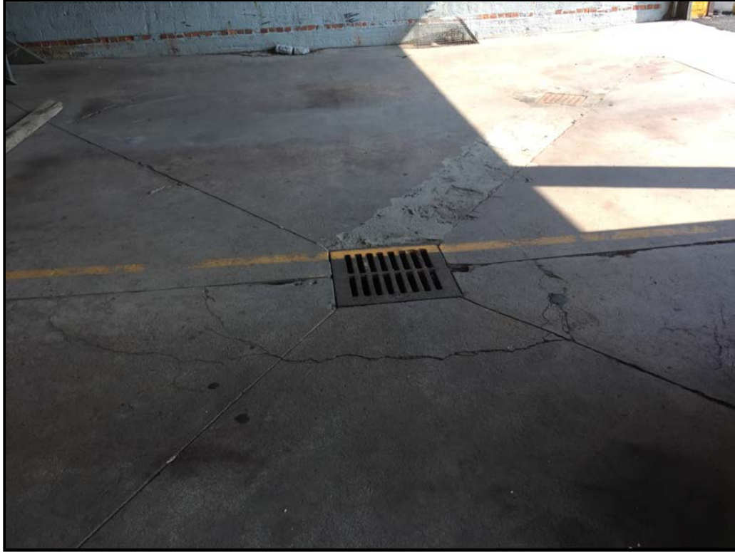
PHOTOGRAPH 9 Cracks in Concrete Floor of Garage on East Side of Building
