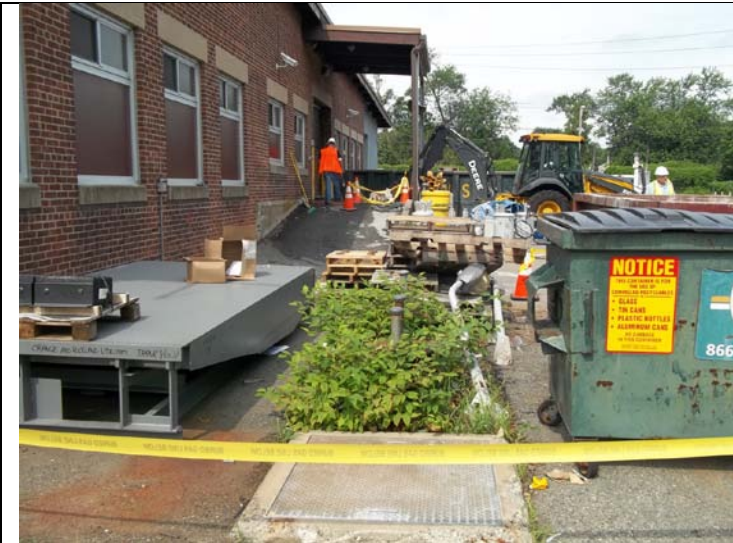
Replacing loading dock platform, soil not impacted
