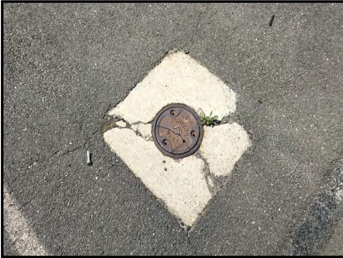
PHOTOGRAPH 15 MW-10S – Crack in concrete pad and cover
