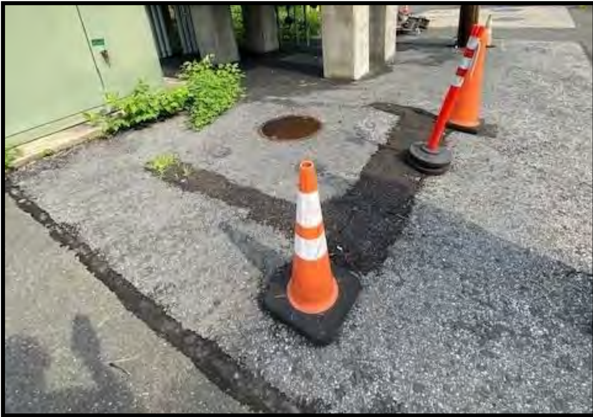
PHOTOGRAPH 15 Fixed Depression/Crack in Pavement Patch for Emergency Generator
