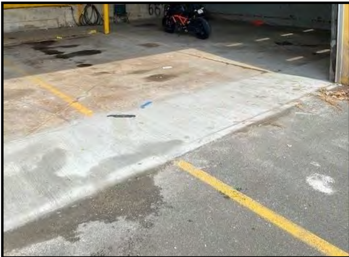
PHOTOGRAPH 16 Cracks in Concrete Floor Fixed of Garage on East Side of Building
