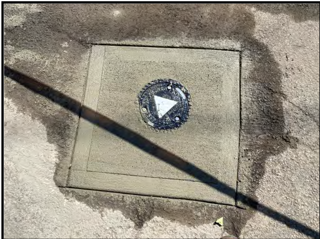
PHOTOGRAPH 16 MW-5B Repaired Road box
