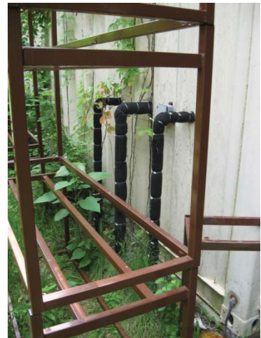
Inlet Groundwater Entering Trailer
