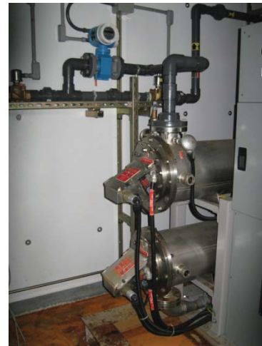
UV/Oxidation Chambers
