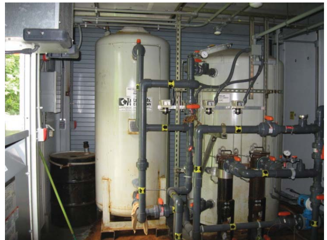
Aqueous Phase GAC and H2O2 Destruct Units
