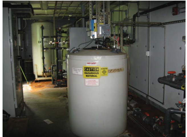
Hydrogen Peroxide Storage Tank
