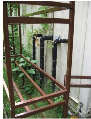
Inlet Groundwater Entering Trailer
