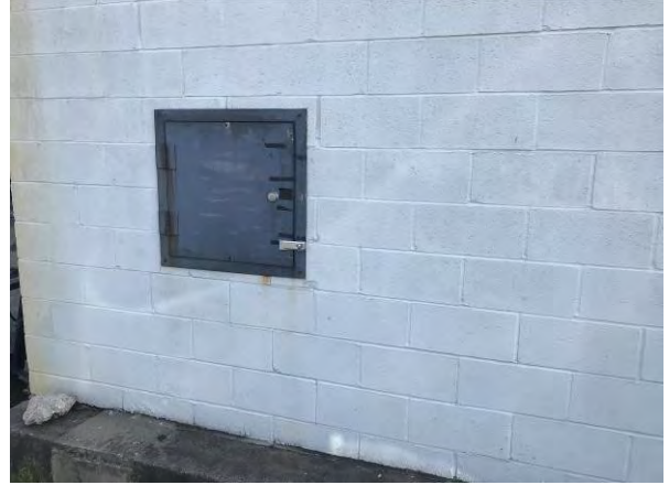
Photo 2: The hatch that allows access to the telecom system was secure.
