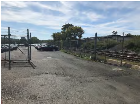
Photo 5: Northern gate to the parking lot used by the automotive warehouse. Secured when not in use.
