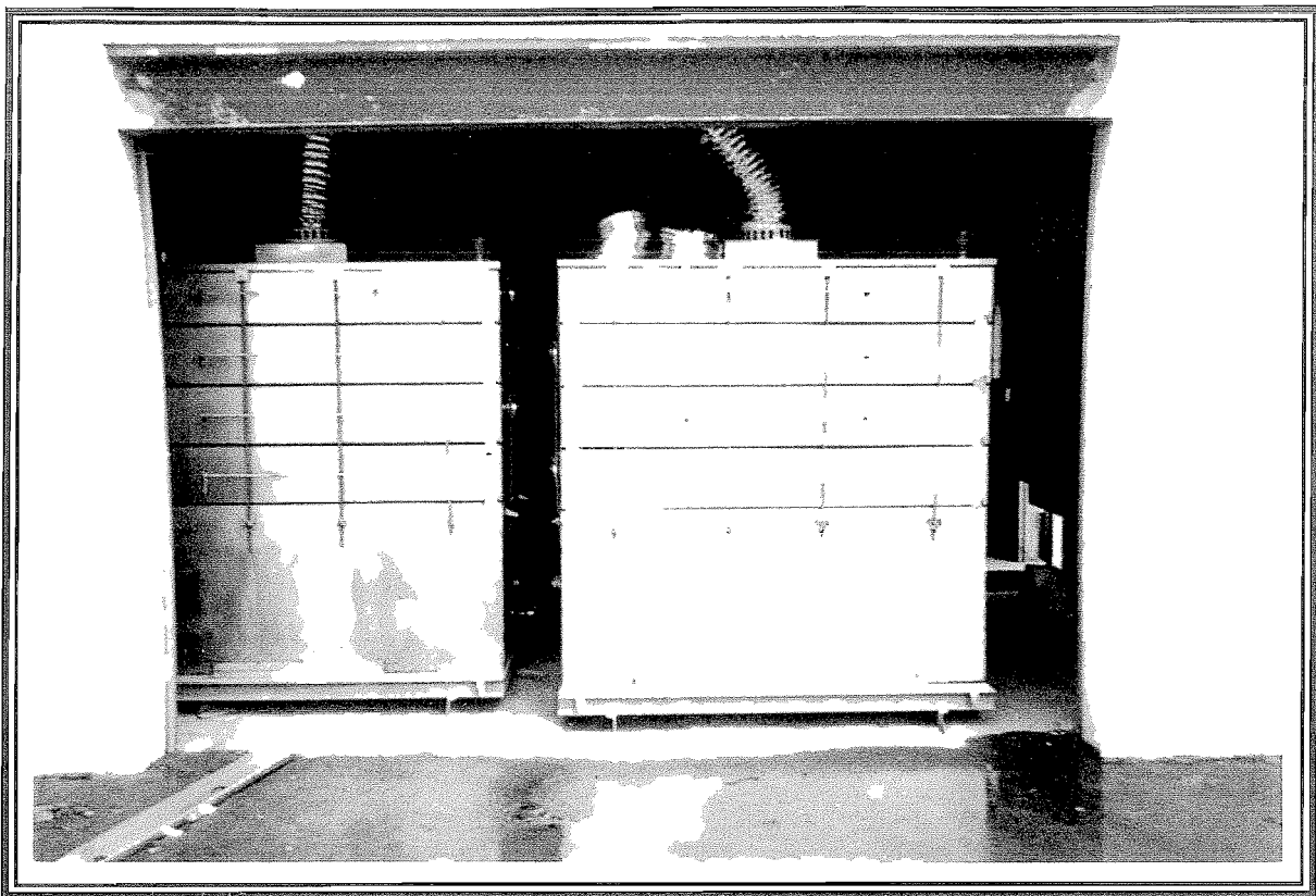
Photo # 1 – Photograph, with the garage door up, of the air stripper towers inside the treatment building.
