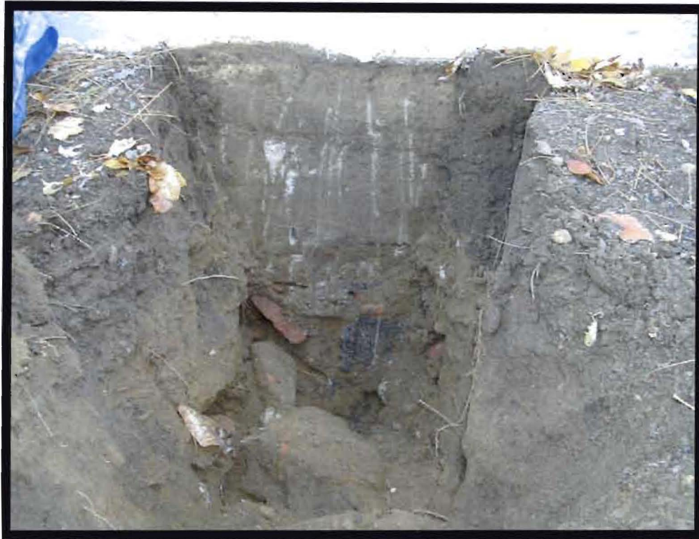
Test Pit GT-TP3, Located At Driveway End Of The Building. Note Rubble And Fill Under The Formed Walls; No Apparent Or Existing Footer At This Location.
