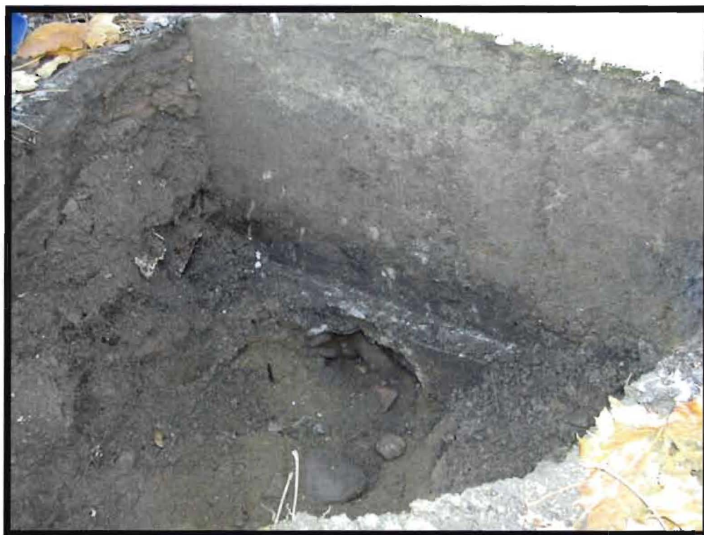
Test Pit GT-TP2, Located At Midpoint Of Building. Note The Small Footing Underneath The Formed Wall.
