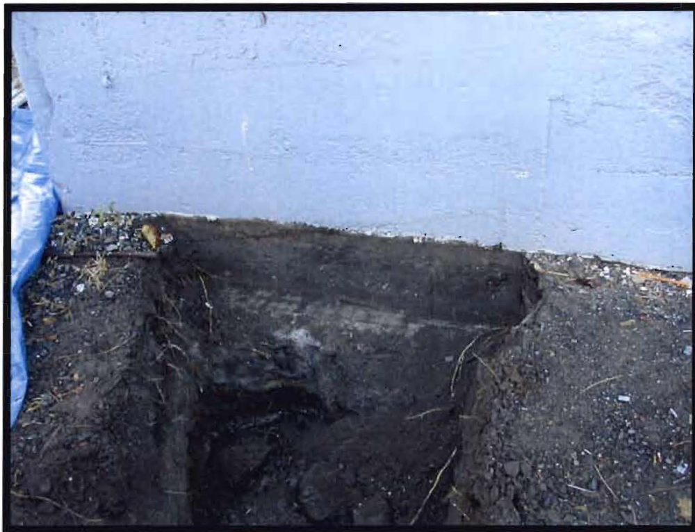
Test Pit GT-TP1, Located At Alley-end Of The Building. Note The Small (4-inch Wide) Ledge Of Overpour From The Forms. Fill Material Is Present Under The "footer".
