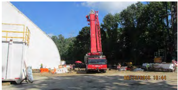
08 15 16 Overall Site and Crane Work
