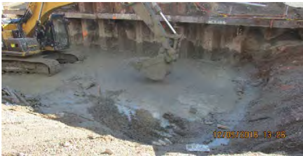
12 05 16 site and bucket mixing
