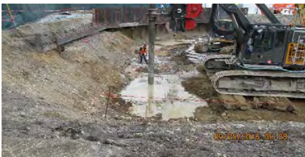
09 29 16 ISS pilot and soil sampling
