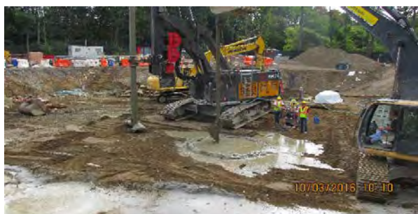
10 03 16 Area D ISS and TFS 5 backfill
