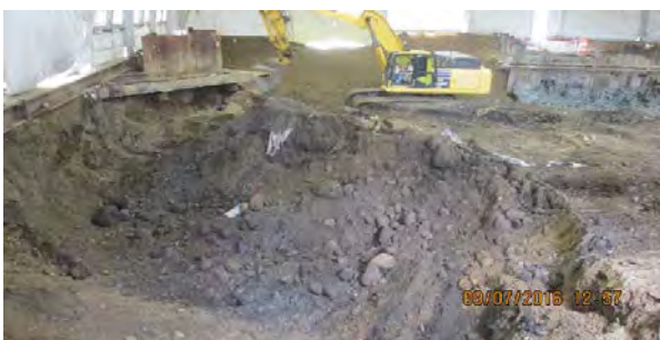
09 07 16 Del Mag and B1 Excavation
