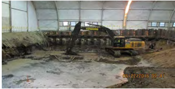
06 22 16 ISS in B1 and sampling
