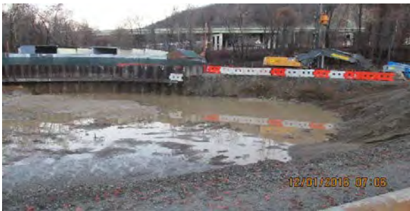
12 01 16 Site after rains
