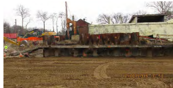
12 08 16 G1 Auger mixing and backfilling B-20
