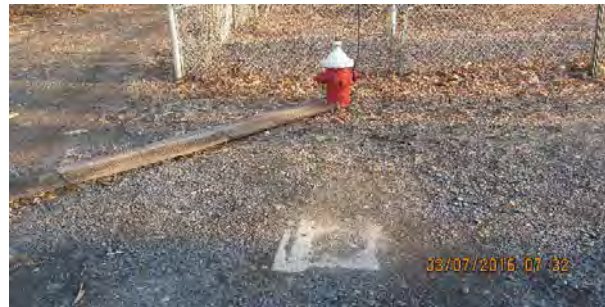
03 07 16 Pre-Construction and Tree Clearing
