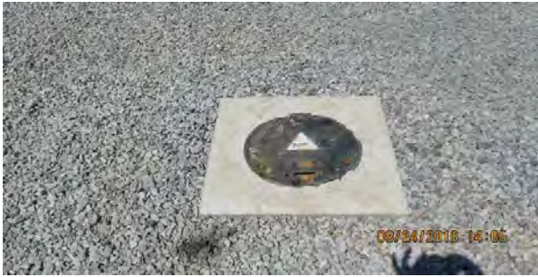
08 24 16 Area A and sparge well pads
