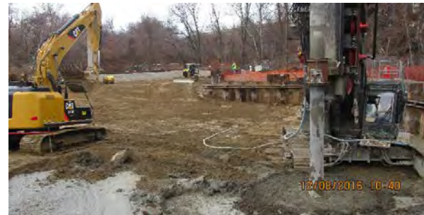
12 08 16 G1 Auger mixing and backfilling B-20
