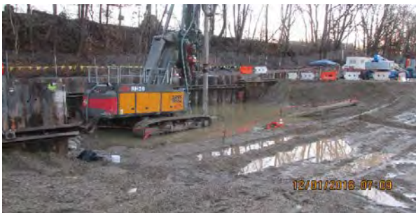
12 01 16 Site after rains
