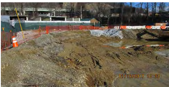
01 19 17 Backfilling
