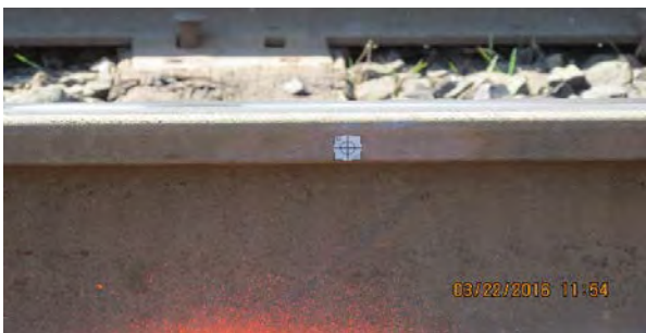
03 22 16 NJT washout and settlement monitor
