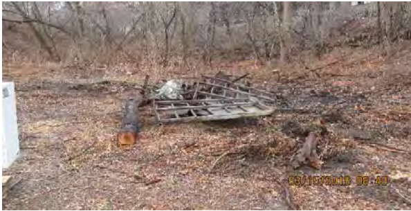
03 15 16 Site Prep continues
