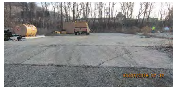
03 07 16 Pre-Construction and Tree Clearing
