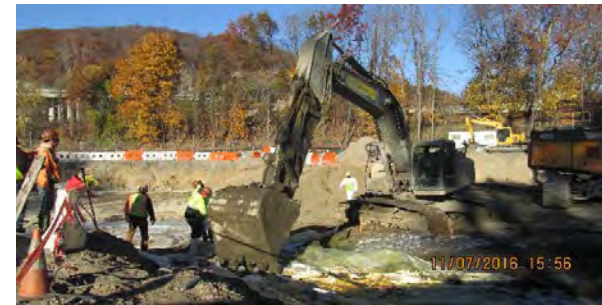
11 07 16 ISS and hydraulic spill from 350
