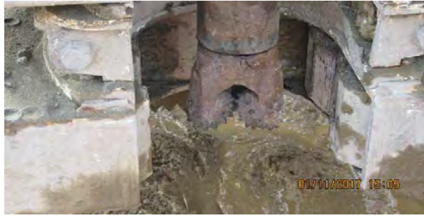
01 11 17 Pilot Holes in Area D
