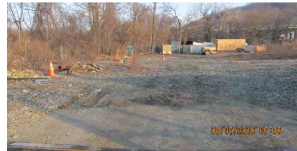
03 07 16 Pre-Construction and Tree Clearing
