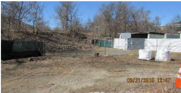
03 21 16 site and WTP area
