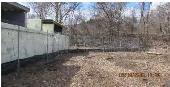
03 18 16 Site Prep continues
