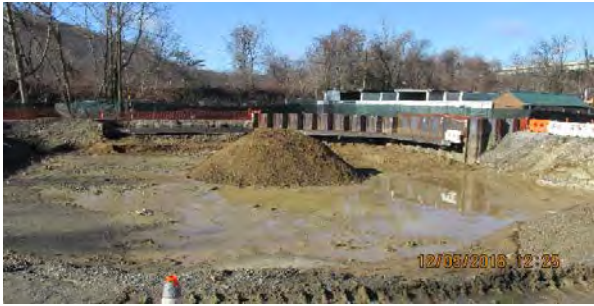
12 05 16 site and bucket mixing
