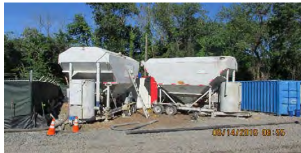
06 14 16 carbon delivery and batch plant
