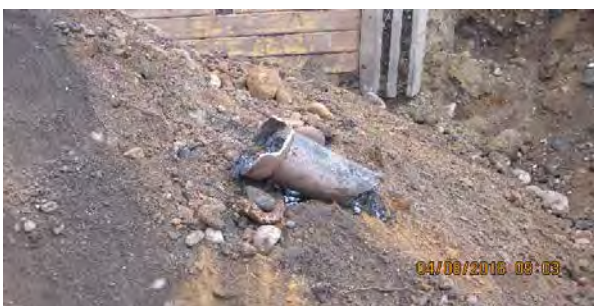
04 08 16 Area C and H old pipe
