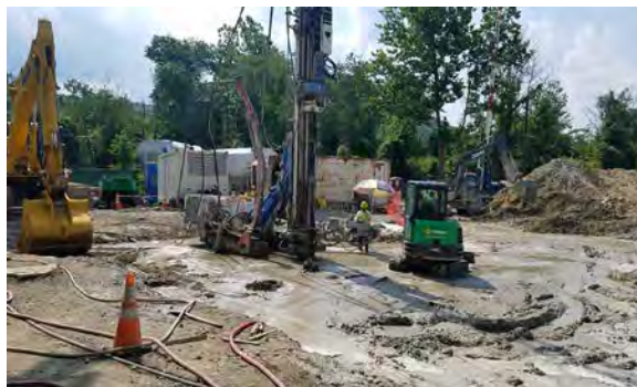
07 12 17 - Jet Grouting Activities Area F
