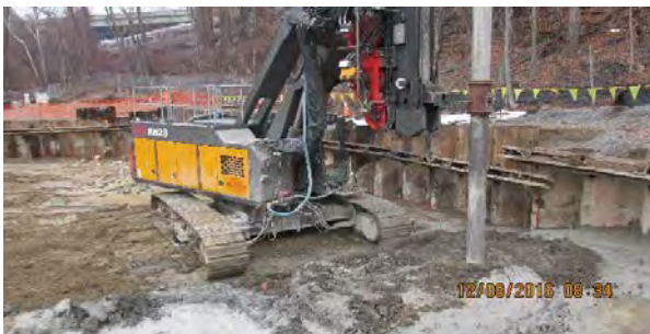
12 08 16 G1 Auger mixing and backfilling B-20
