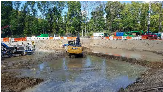
05 16 17 - Segregation Berm Installation AreaD
