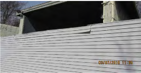
03 07 16 Pre-Construction and Tree Clearing - Gun Club
