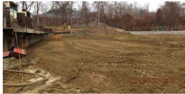
12 08 16 G1 Auger mixing and backfilling B-20
