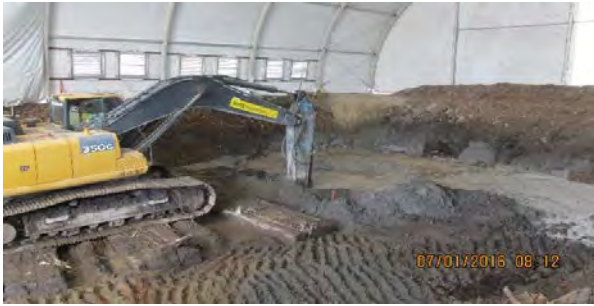
07 01 16 Cell B-5 mixing and sample
