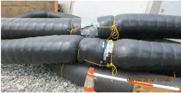
08 05 16 Gas Holder and backfilling
