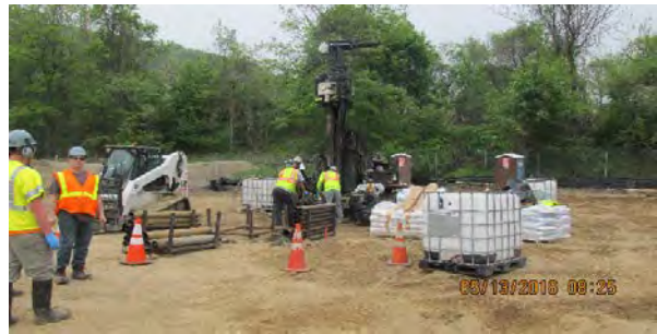
05 13 16 Area A sparge wells backfill and TFS
