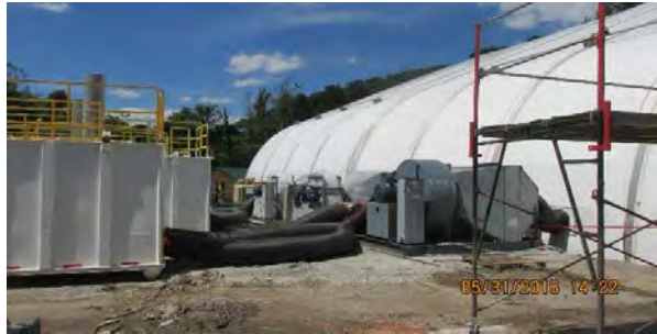
05 31 16 Sparge Well and site
