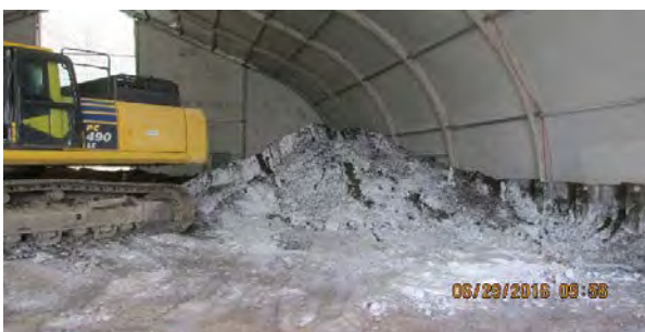
05 13 16 Area A sparge wells backfill and TFS
