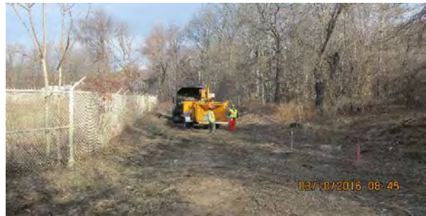
03 10 16 tree cutting and site
