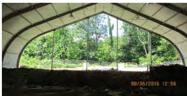
08 05 16 Gas Holder and backfilling
