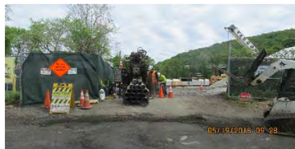
05 19 16 Water line removal and sparge wells
