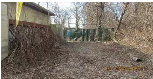
03 10 16 tree cutting and site
