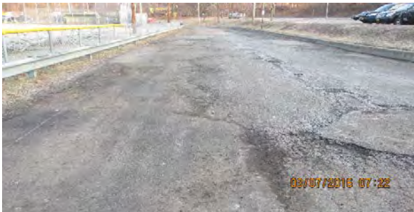
03 07 16 Pre-Construction and Tree Clearing - Pat Malone Drive
