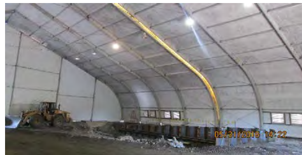
05 31 16 Sparge Well and site
