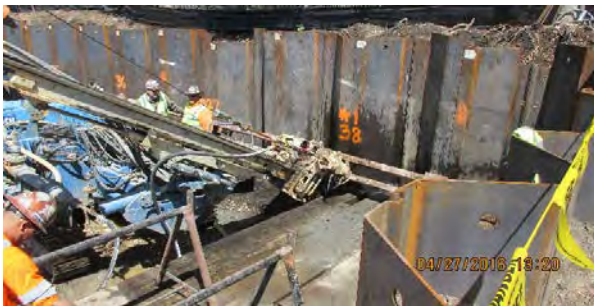
04 27 16 start tie backs
