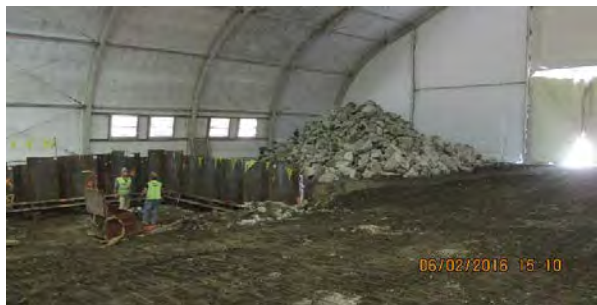
06 02 16 Sparge Install and Main site
