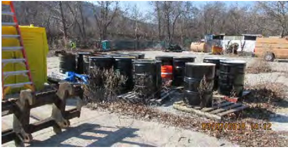
03 07 16 Pre-Construction and Tree Clearing
