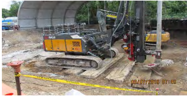
09 07 16 Del Mag and B1 Excavation
