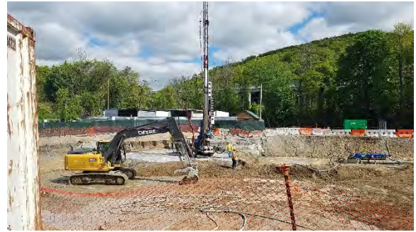
05 10 17 - Jet Grout Rig Set Up Area D
