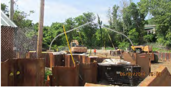
06 02 16 Sparge Install and Main site
