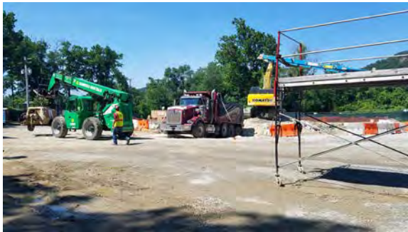
07 21 17 - Site Restoration Activities
