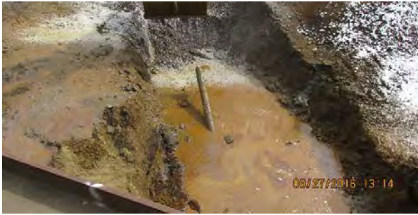
09 27 16 Area D and B1 Backfill
