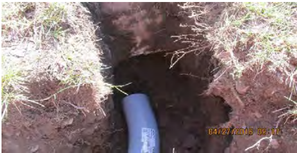
04 27 16 start tie backs
