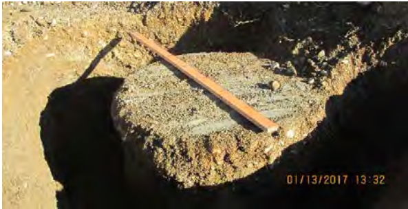
01 13 17 pilot test column excavation
