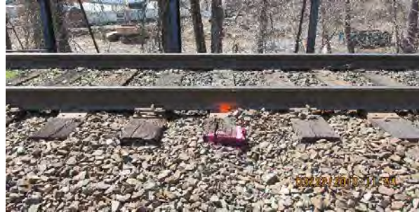
03 22 16 NJT washout and settlement monitor
