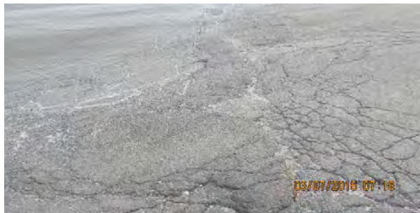
03 07 16 Pre-Construction and Tree Clearing - Pat Malone Drive
