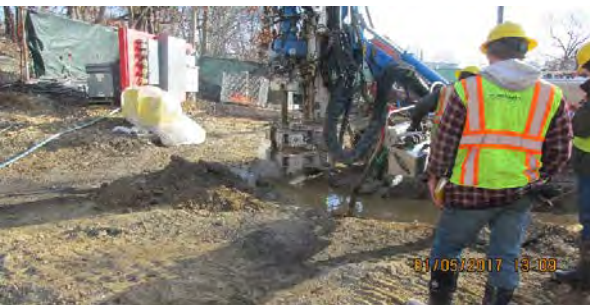
01 05 17 ISS Jet Grout Pilot
