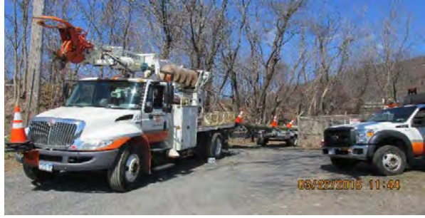
03 22 16 NJT washout and settlement monitor
