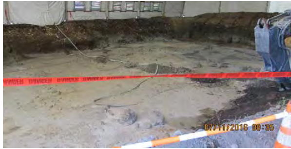
07 11 16 Auger mixing prep
