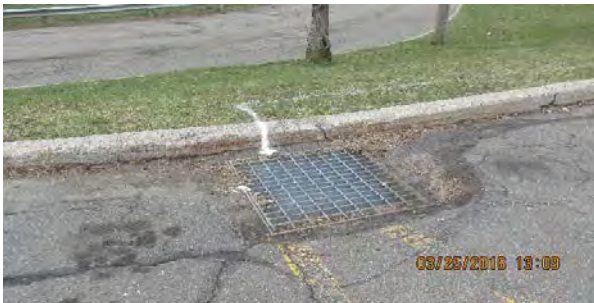
03 25 16 WTP and site
