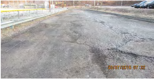
03 07 16 Pre-Construction and Tree Clearing - Pat Malone Drive
