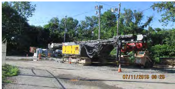
07 11 16 Auger mixing prep
