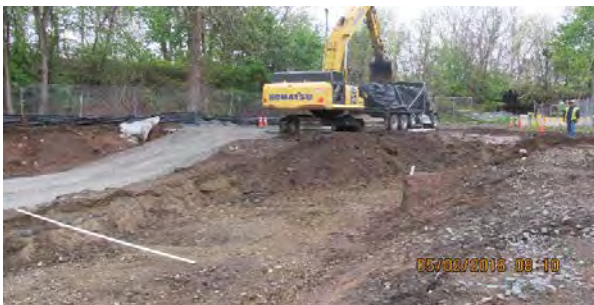
05 02 16 Area A moretrench and sparge wells
