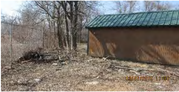
03 07 16 Pre-Construction and Tree Clearing - Gun Club
