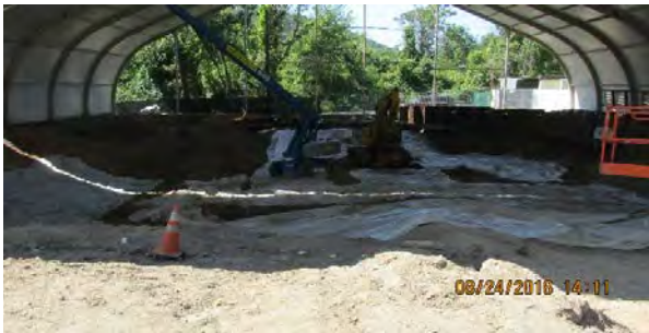
08 24 16 Area A and sparge well pads
