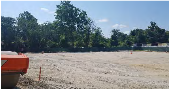
07 31 17 - Site Conditions NW View
