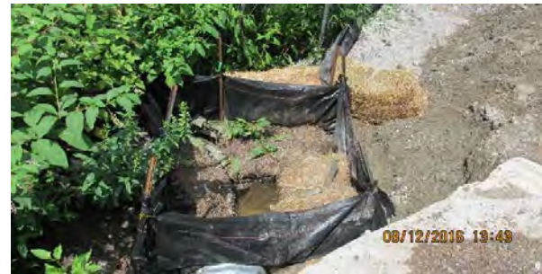
08 12 16 overall site and storm water
