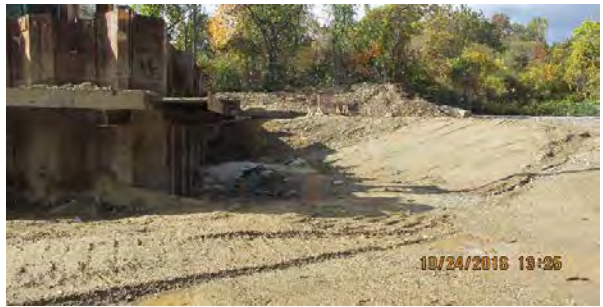
10 24 16 Area F and demolition
