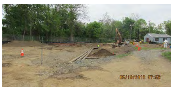
05 19 16 Water line removal and sparge wells
