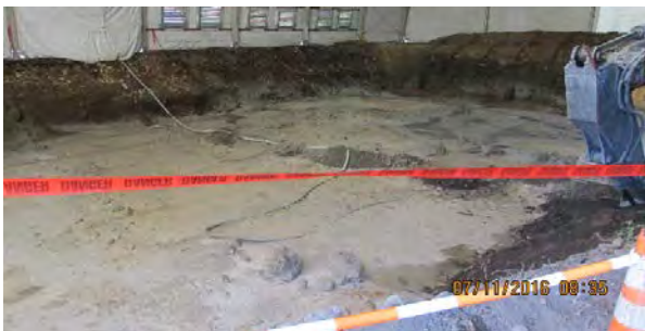
07 11 16 Auger mixing prep
