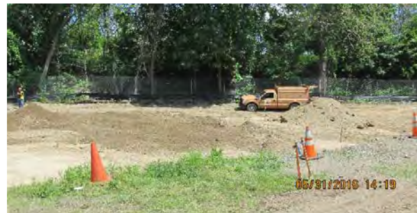
05 31 16 Sparge Well and site
