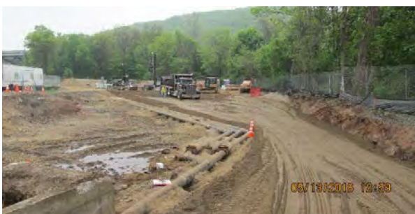
05 13 16 Area A sparge wells backfill and TFS
