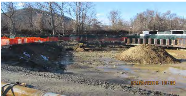
12 05 16 site and bucket mixing
