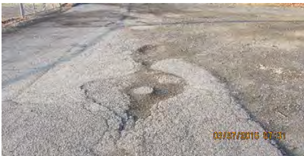
03 07 16 Pre-Construction and Tree Clearing - Pat Malone Drive
