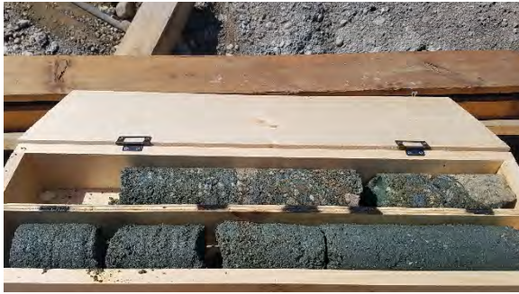
06 22 17- Jet Grout Coring _101207
