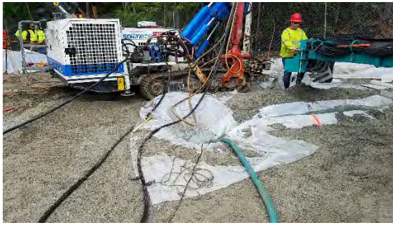
05 05 17 - Pre-Drill Water Sump Area G
