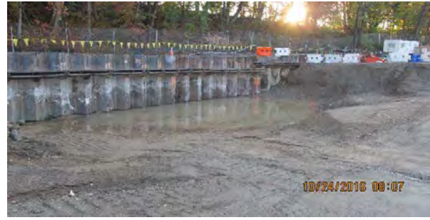
10 24 16 Area F and demolition
