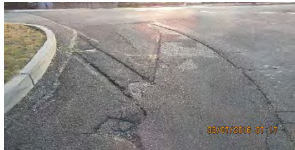
03 07 16 Pre-Construction and Tree Clearing - Pat Malone Drive
