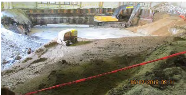
06 27 16 backfilling B1
