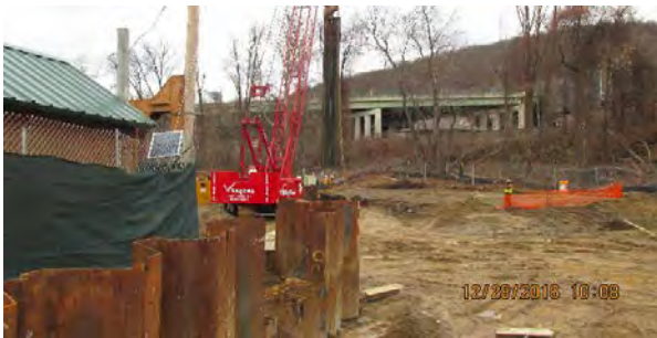
12 28 16 ISS coring and pulling SSP
