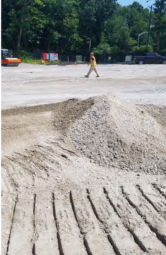
08 03 17 - Backfill Scrape J322
