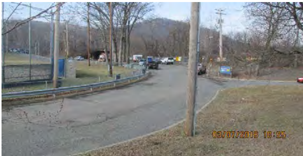
03 07 16 Pre-Construction and Tree Clearing
