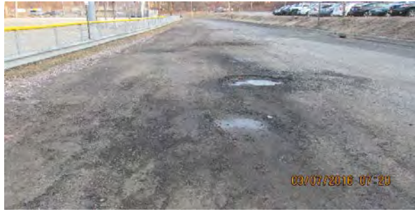
03 07 16 Pre-Construction and Tree Clearing - Pat Malone Drive
