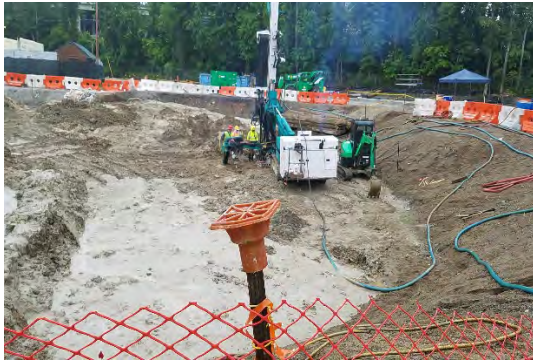
05 25 17 - Pre-Drill Maintenance AreaD
