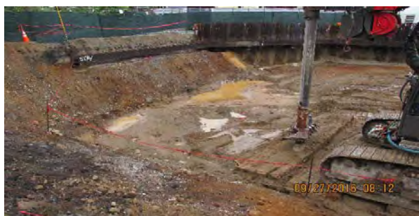
09 27 16 Area D and B1 Backfill
