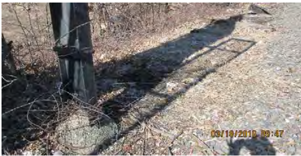
03 18 16 Site Prep continues
