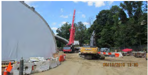
08 15 16 Overall Site and Crane Work
