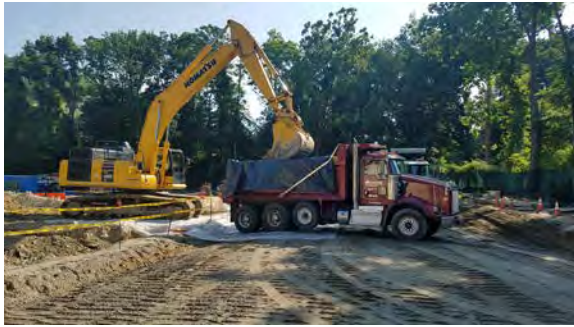
07 15 17 - Spoils Load Out
