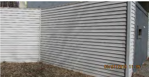
03 07 16 Pre-Construction and Tree Clearing - Gun Club
