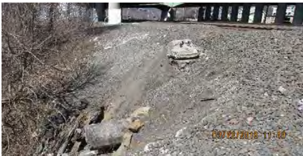
03 22 16 NJT washout and settlement monitor
