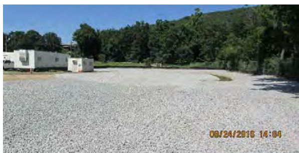
08 24 16 Area A and sparge well pads
