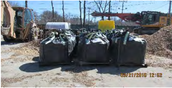
03 21 16 site and WTP area
