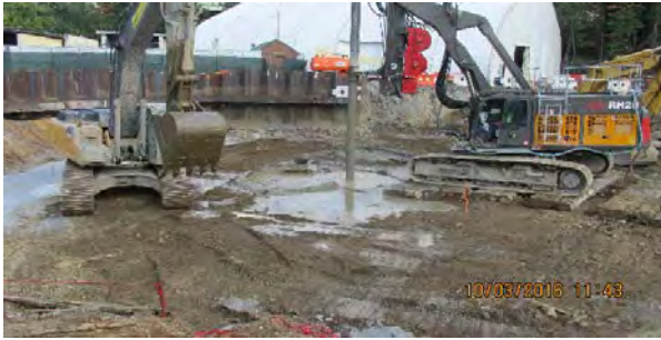
10 03 16 Area D ISS and TFS 5 backfill
