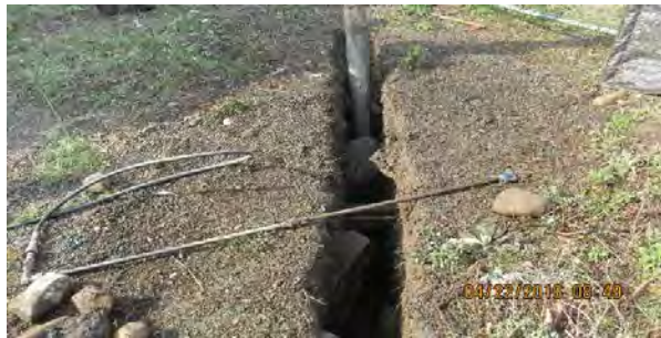
04 22 16 Area A walers and sparge wells
