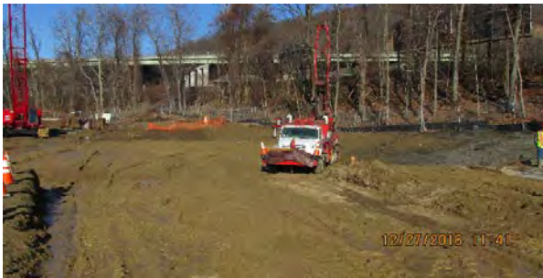
12 27 16 ISS coring and site conditions
