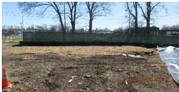
03 21 16 site and WTP area
