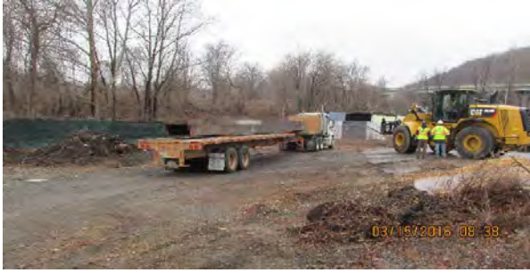
03 15 16 Site Prep continues
