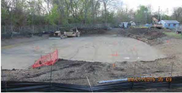
04 27 16 start tie backs
