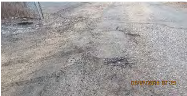
03 07 16 Pre-Construction and Tree Clearing - Pat Malone Drive
