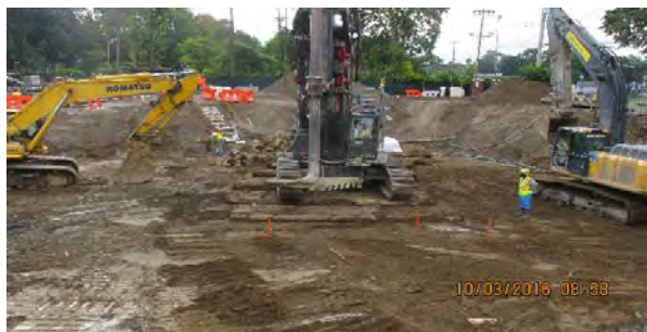
10 03 16 Area D ISS and TFS 5 backfill
