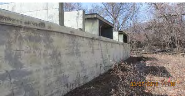
03 07 16 Pre-Construction and Tree Clearing - Gun Club
