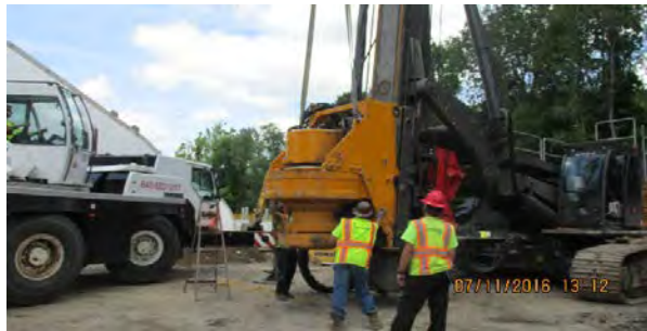
07 11 16 Auger mixing prep
