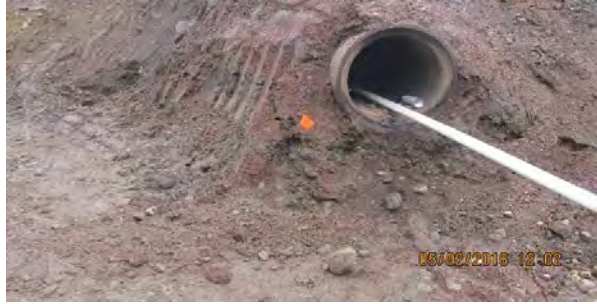
05 02 16 Area A moretrench and sparge wells
