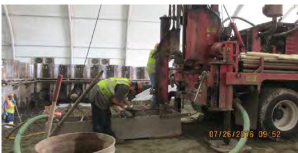
07 26 16 ISS Coring and sampling
