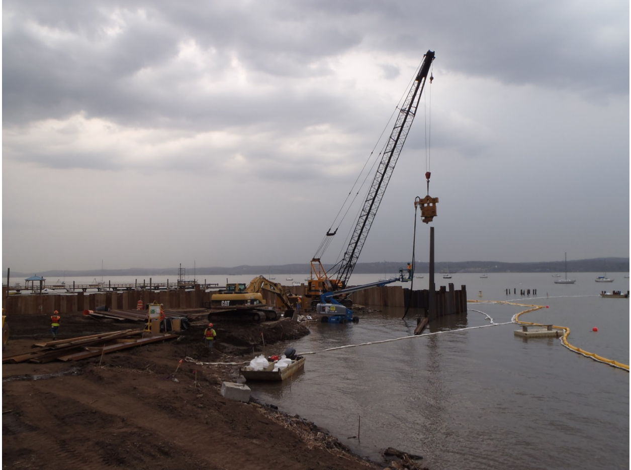
Sheetpile wall installation, looking northeast
