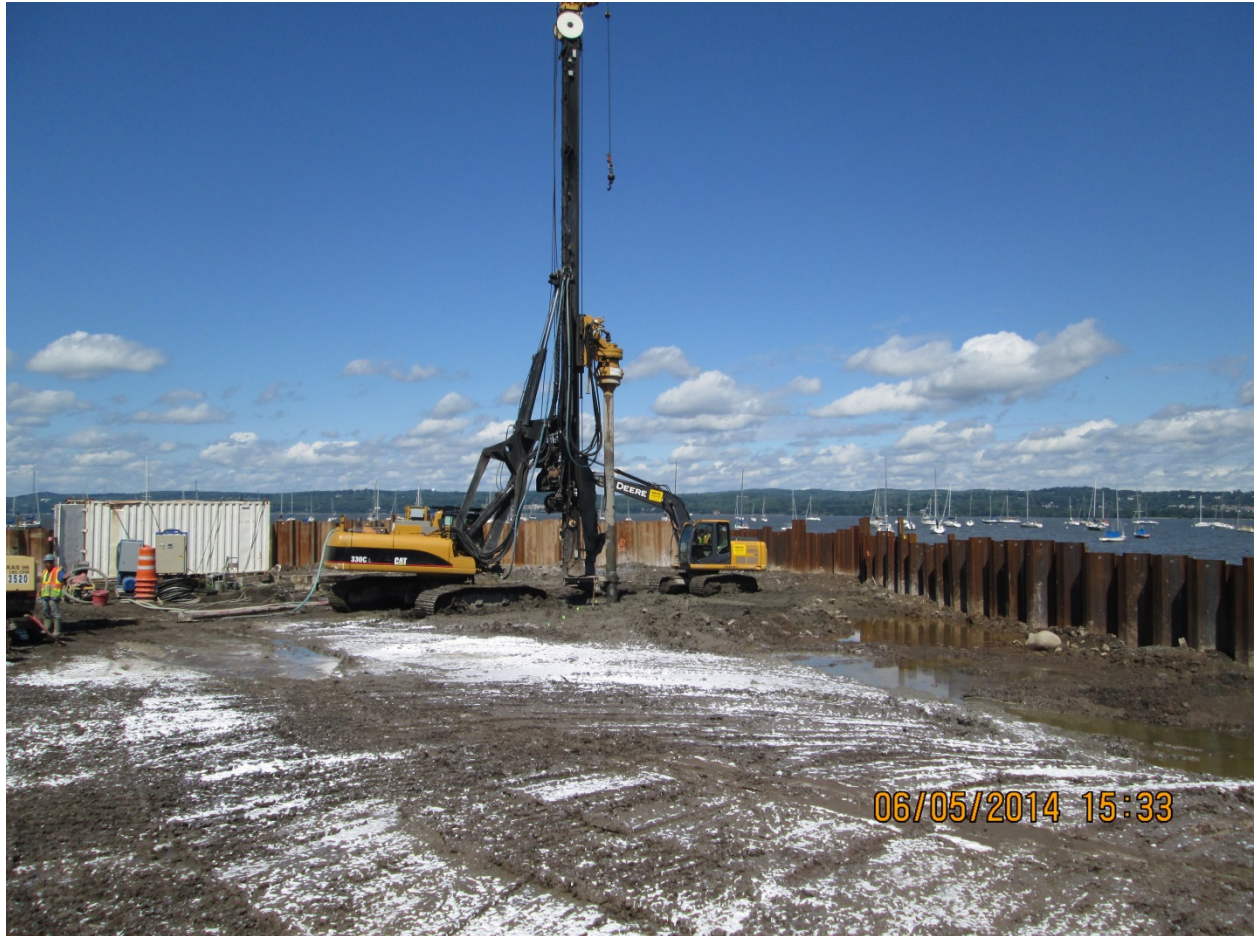
In-Situ solidification (ISS) auger mixing
