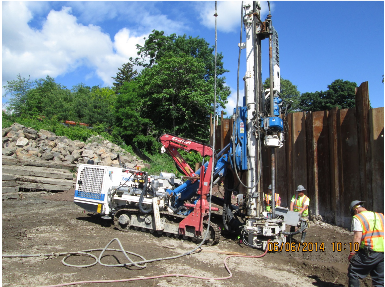
ISS jet-grouting
