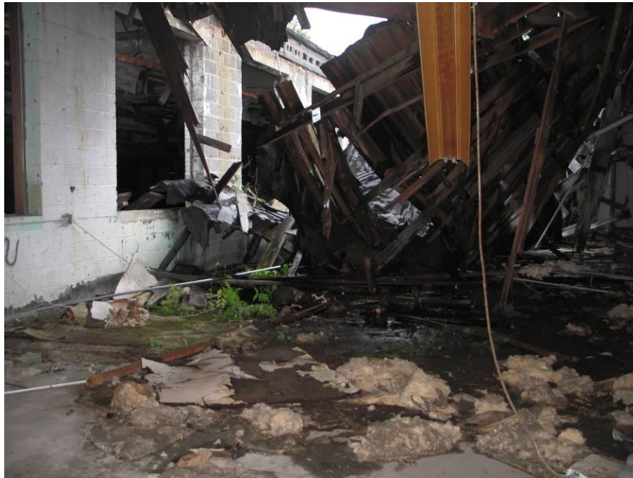
Picture 3 – Collapsed Roof Area
