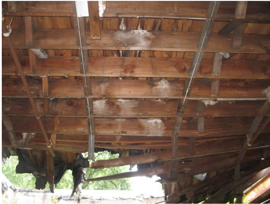
Picture 5 – Cracked Joists Adjacent to Roof Collapse
