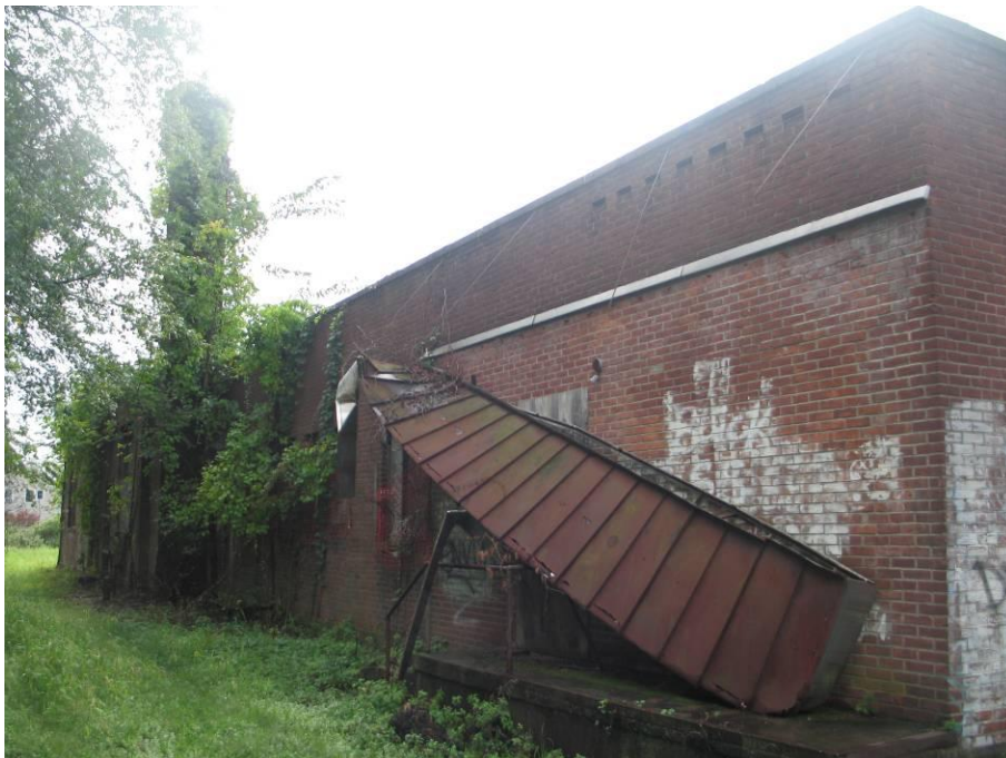
Picture 12 – Collapsed Awning
