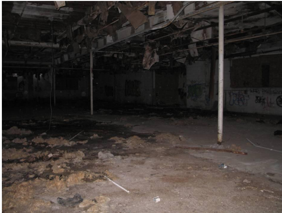
Picture 1 – Roof Leaks and Falling Ceiling Board
