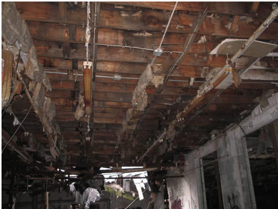
Picture 6 – Cracked Joists
