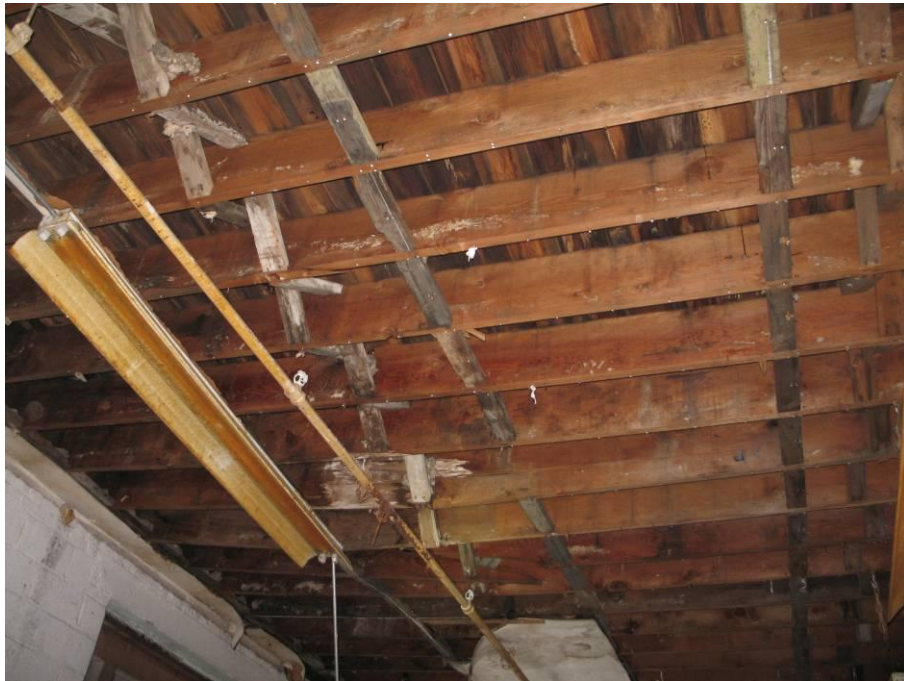
Picture 9 – Cracked Joists
