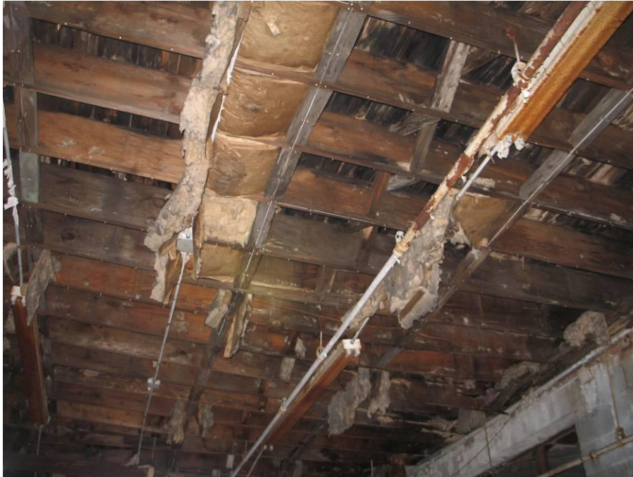
Picture 7 – Cracked Joists
