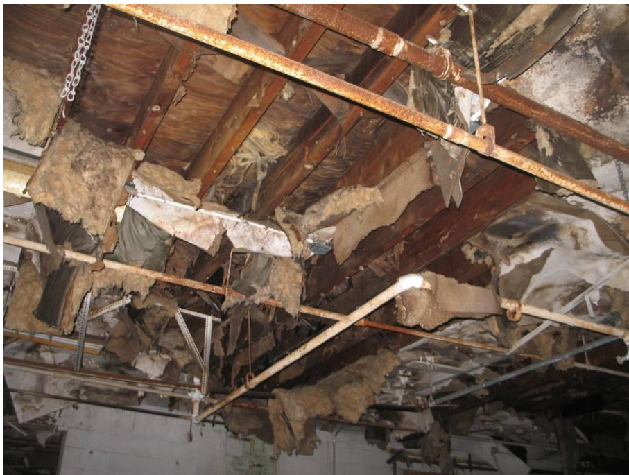
Picture 10 – Plywood Deck Disintegration
