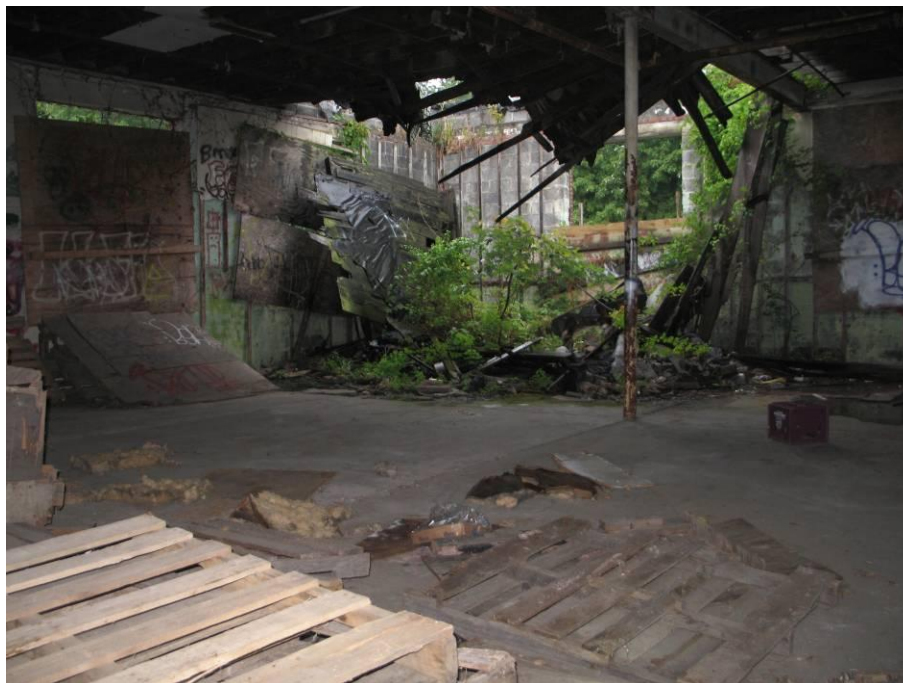
Picture 4 – Collapsed Roof Area
