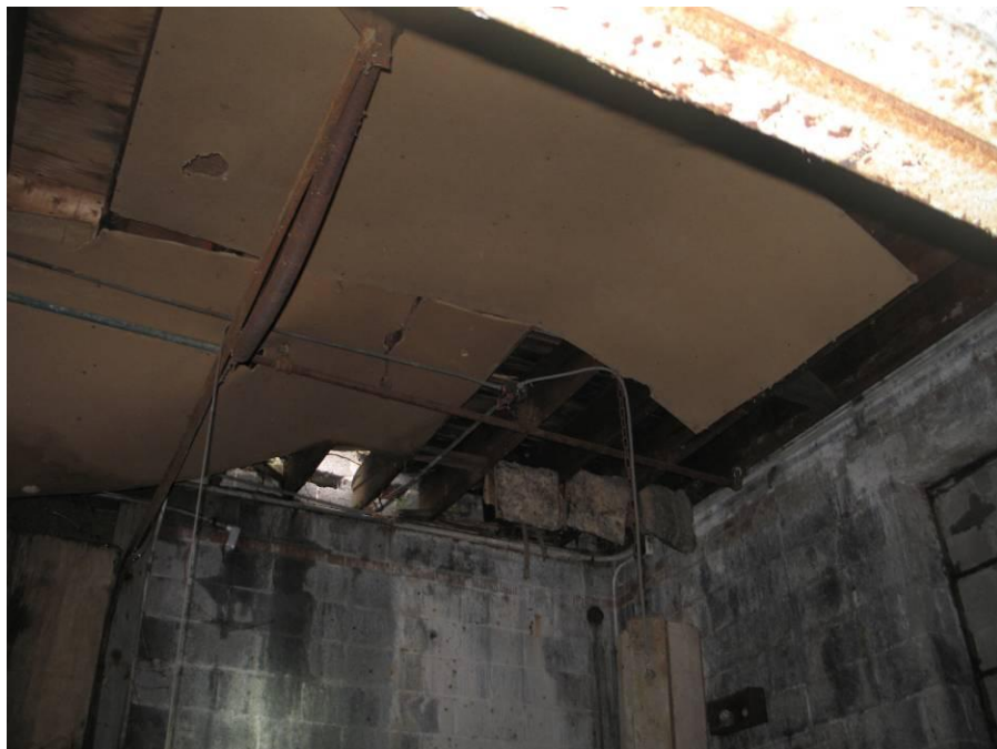
Picture 8 – Cracked Joist at Support
