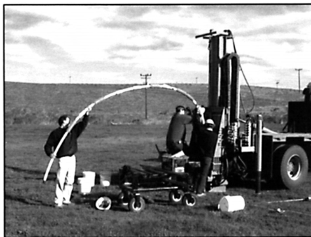
Figure 8. Inserting a CMT multilevel well equipped with bentonite packers and prepacked sand packs.
