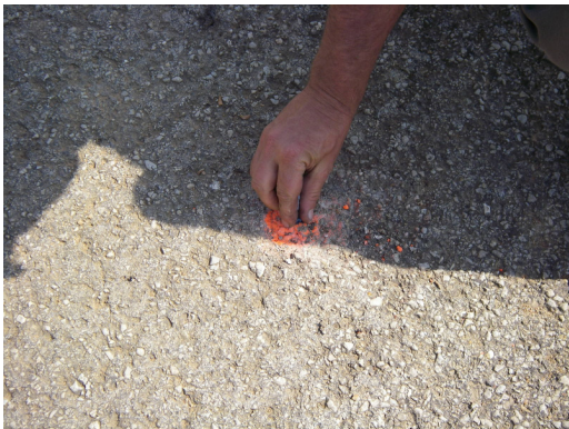
Insert Backer Rod Material
