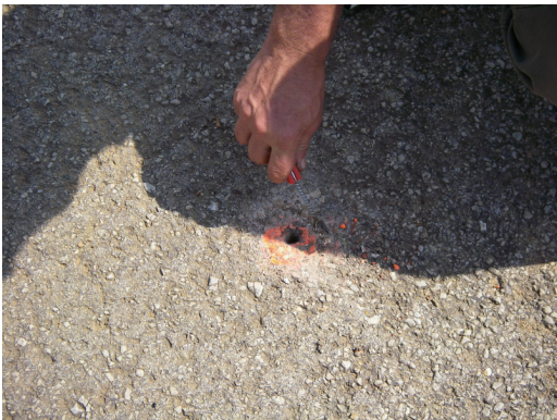
Prepare to Insert Backer Rod Material
