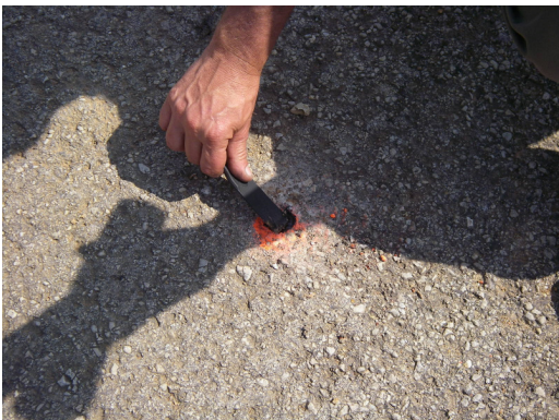
Smooth Patch Material with Putty Knife
