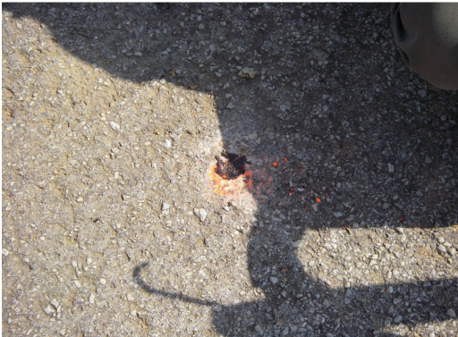
Completed Asphalt Patch (Marking Paint Fades Over Time)
