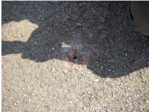
Electrode Stake Hole Ready for Patching
