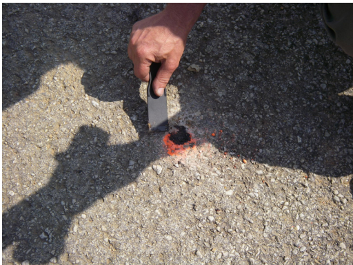
Prepare to Smooth Patch Material
