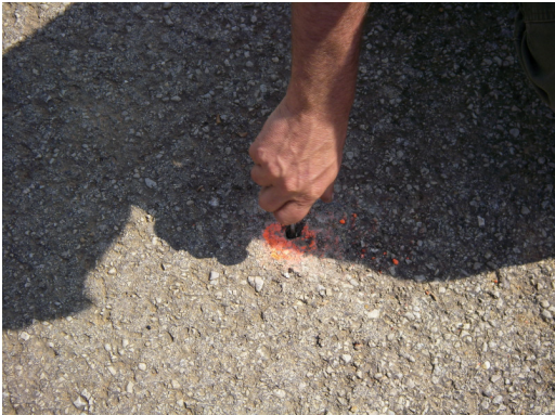
Clean out hole with wire brush
