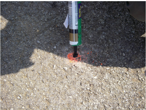
Fill hole with Caulk Patch Material
