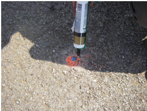
Prepare Patch Caulk Material
