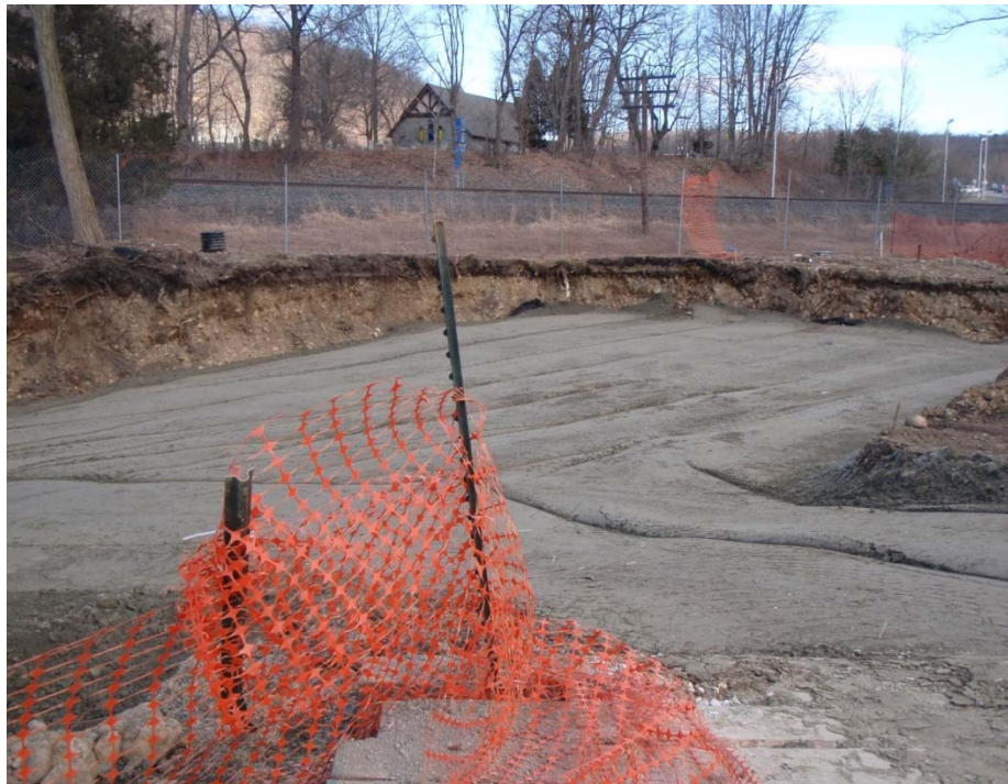
Figure12: Compacted backfill within PS-1
