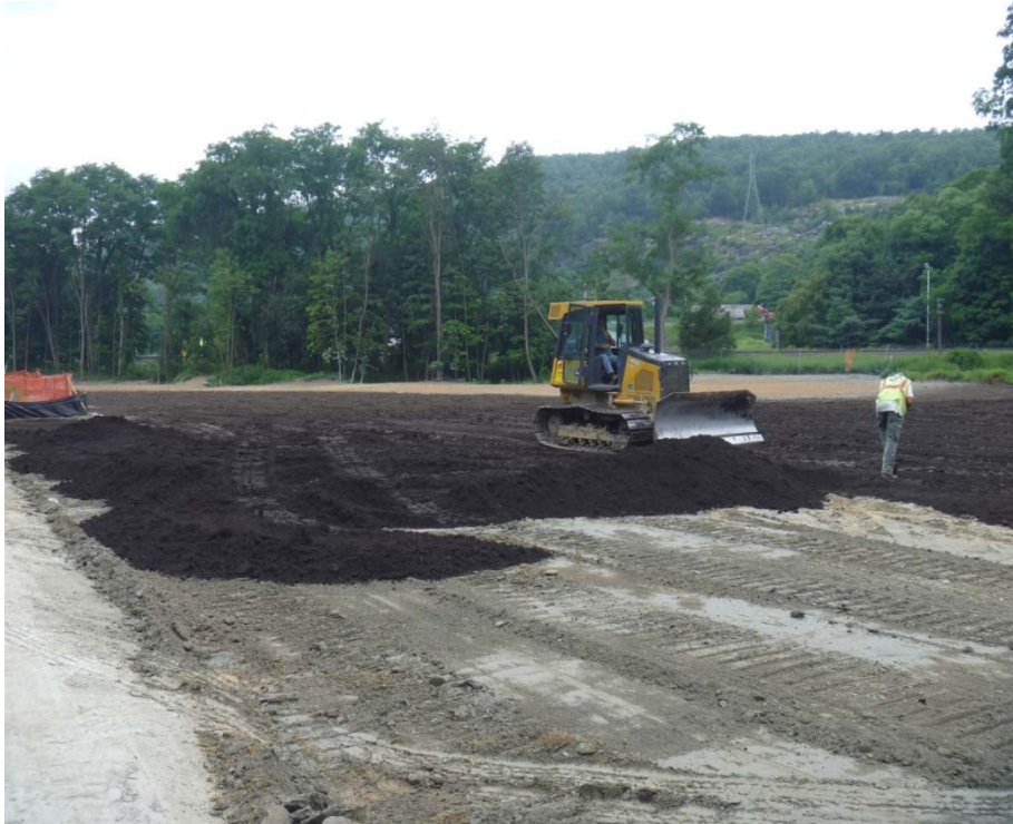
Figure 23: PS-2 Site Restoration (placement of topsoil)
