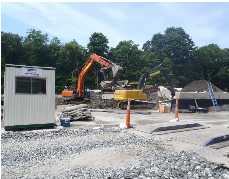
Figure 16: Loading the screener in the Material Storage Area
