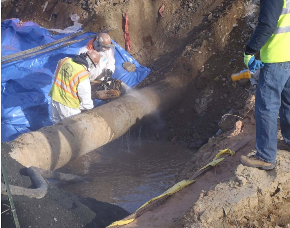
Figure 33: Removal of the Concrete Reinforced Pipe
