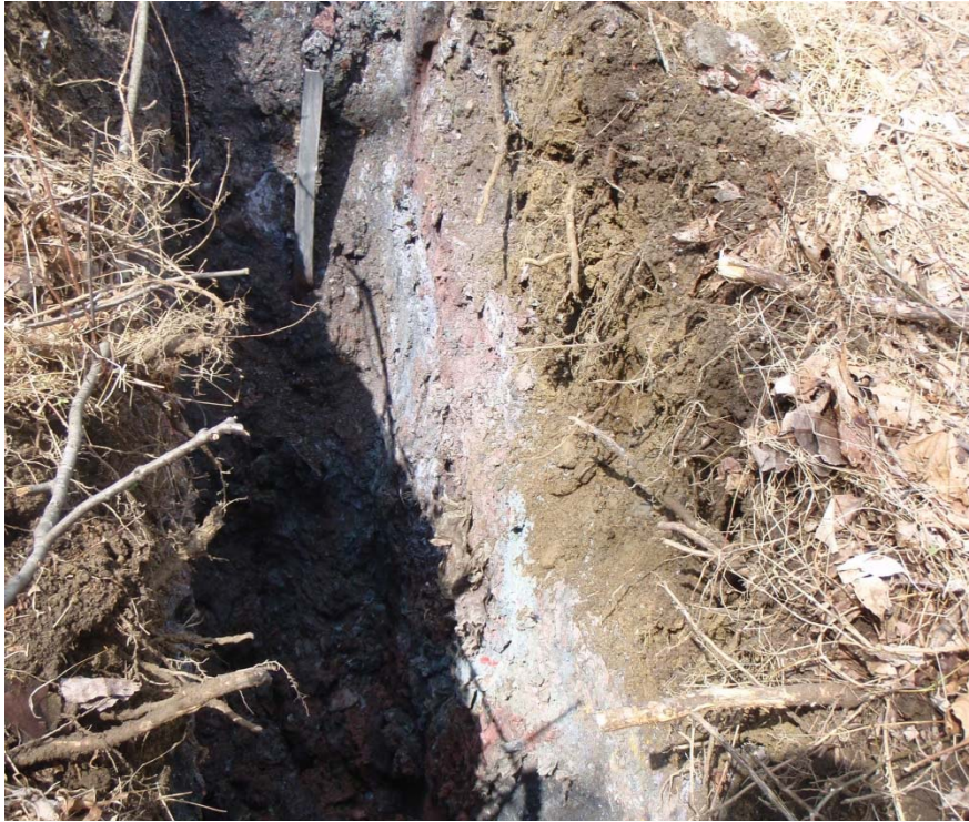
Figure 1: Open Excavation containing Paint Sludge and Impacted Material
