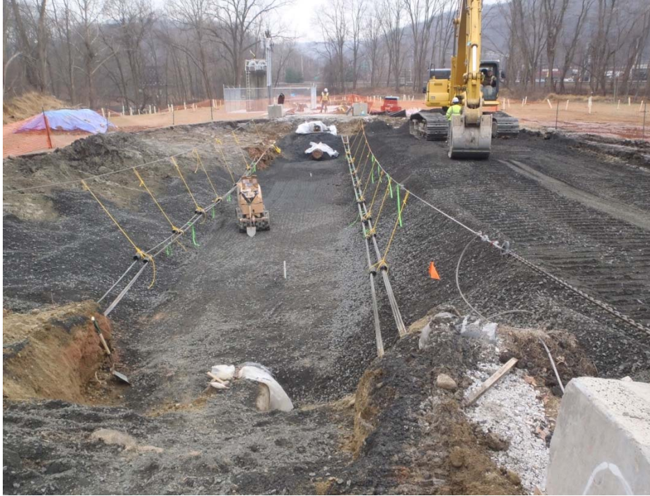
Figure 35: Site Restoration (Backfill of PS-2 Utility Corridor)
