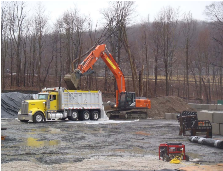
Figure 20: Load out procedures in the Material Storage Area
