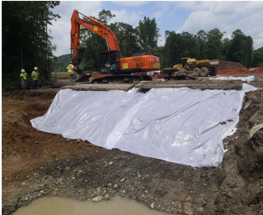
Figure 11: Plastic sheeting to protect the paint sludge and impacted material excavation face
