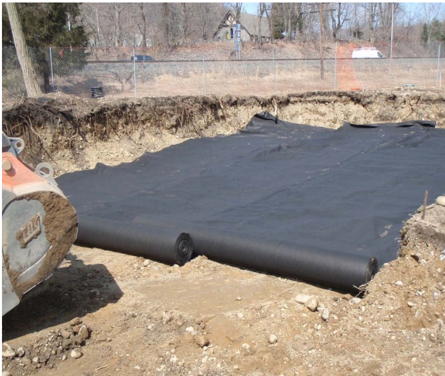
Figure 10: Geotextile fabric demarcation layer in PS-1
