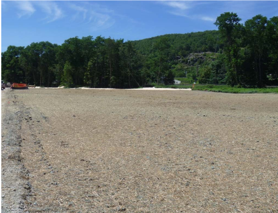
Figure 25: PS-2 Site Restoration (topsoil and seeding)
