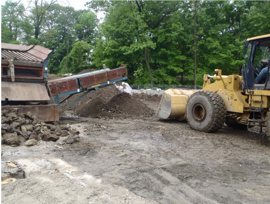
Figure 17: Sorting and segregating paint sludge and impacted material
