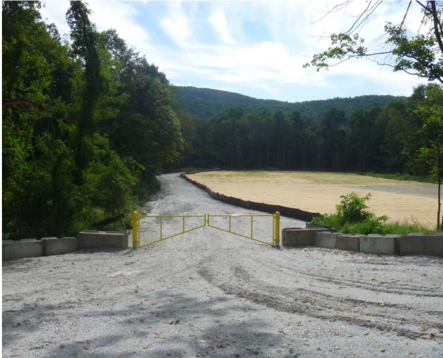
Figure 27: Material Storage Area Site Restoration (seeding and erosion matting)
