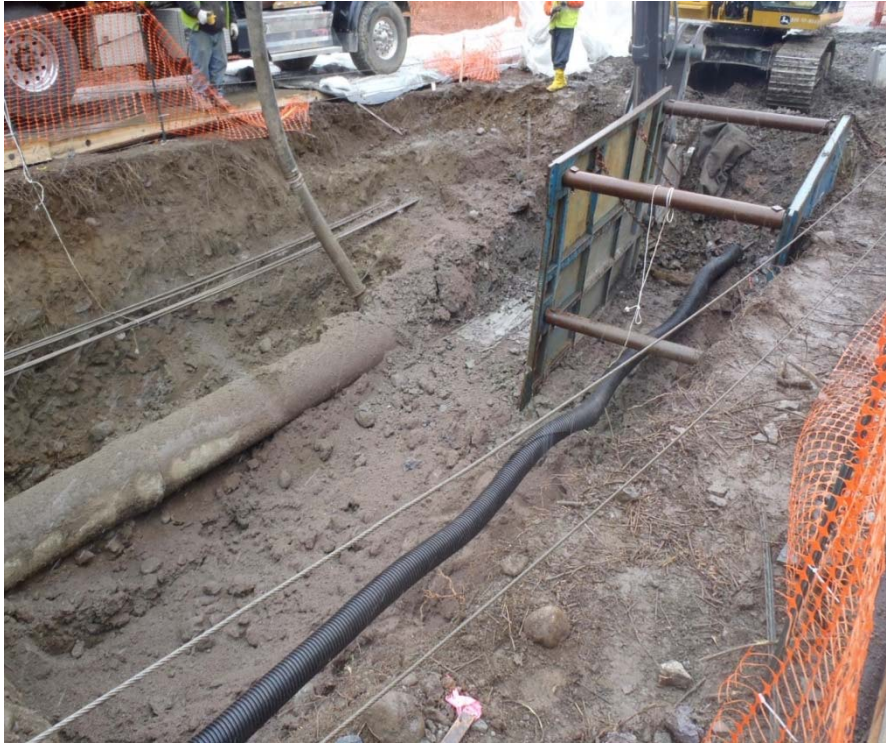
Figure 3: Soil being removed from the PS-3 Utility Corridor
