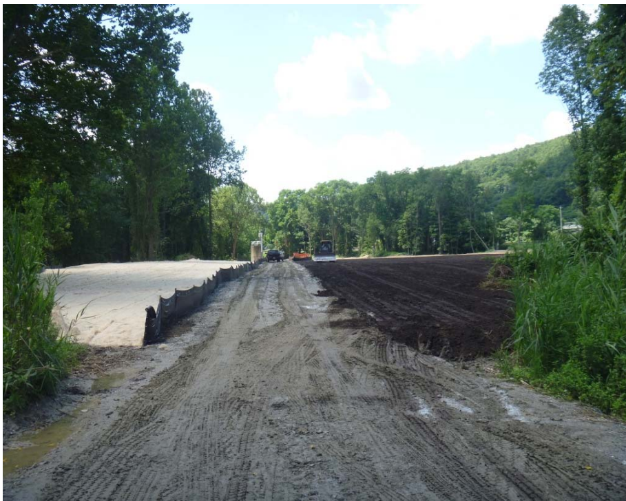
Figure 24: Site Restoration (topsoil seeding and erosion matting)
