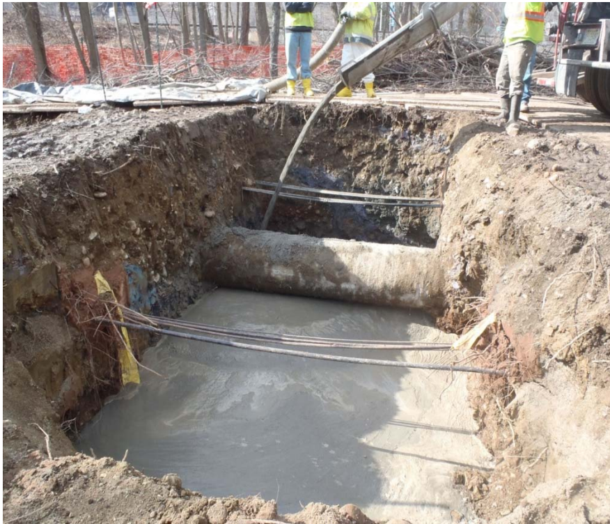
Figure 5: Flowable fill added to an excavated cell within the PS-1 Utility Corridor
