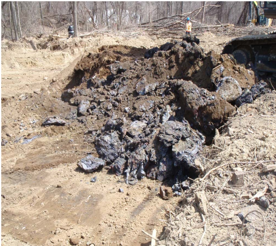
Figure 8: Paint sludge and impacted material encountered in PS-2
