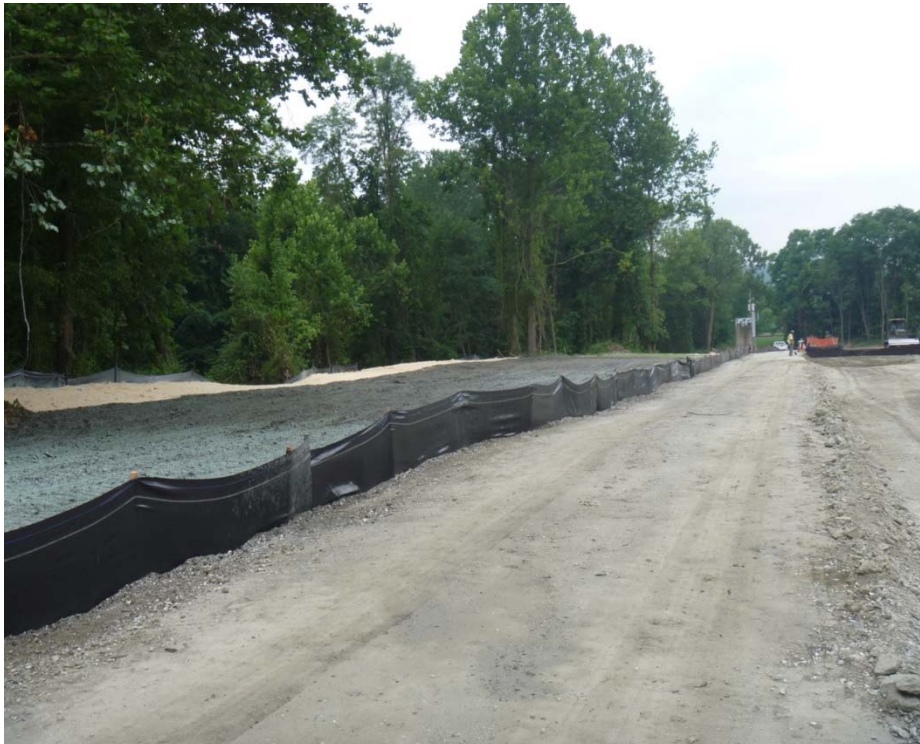
Figure 22: PS-3 Site Restoration (topsoil and seeding)
