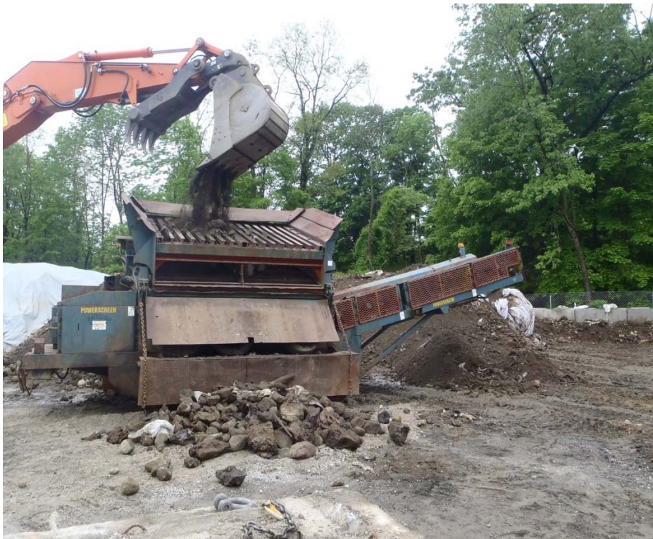
Figure 18: Sorting and segregating paint sludge and impacted material
