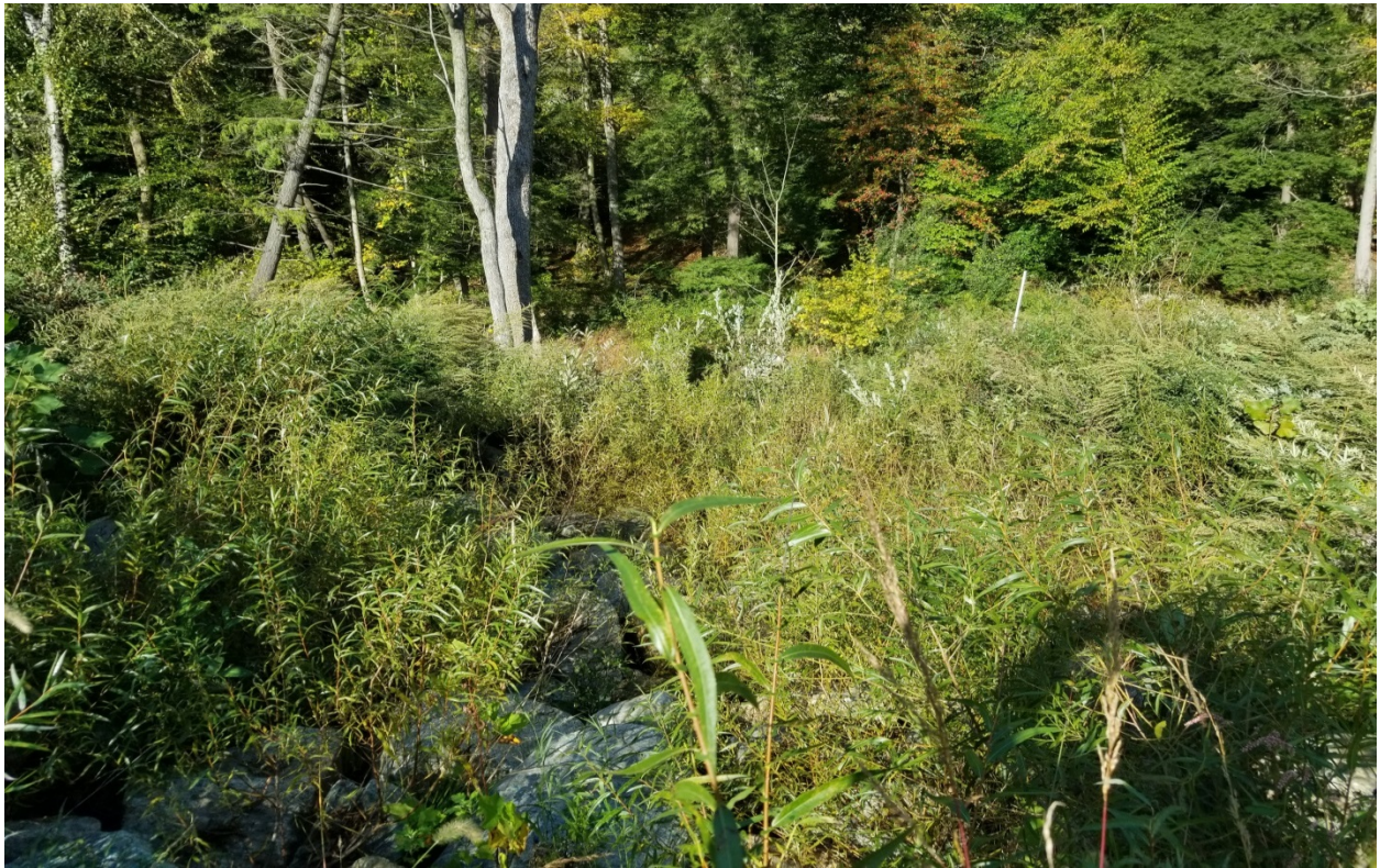
View of the rip rap spillway that flows to Torne Brook showing the establishment of willow live stakes near MP-3.
