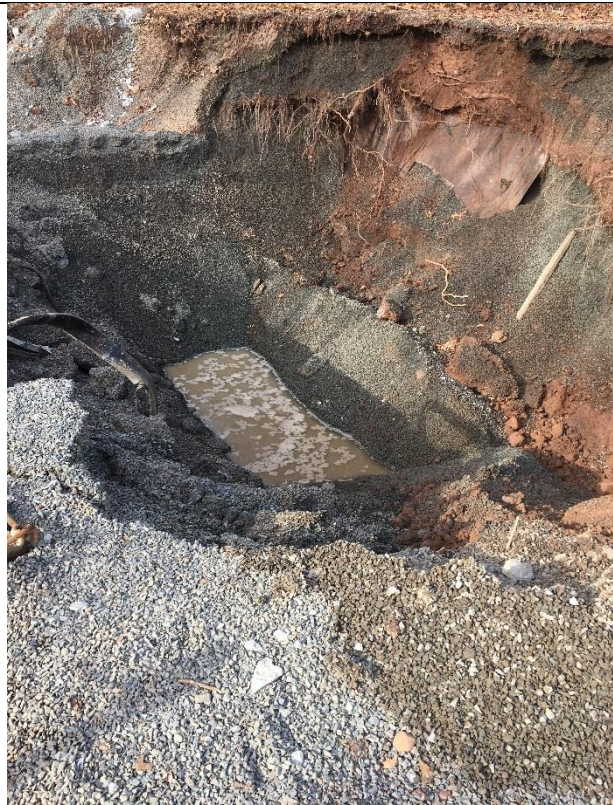
Photograph: 5 | Groundwater experienced in excavation
