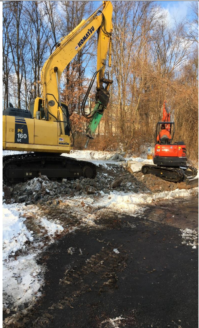
Photograph: 1 | Breaking of concrete
