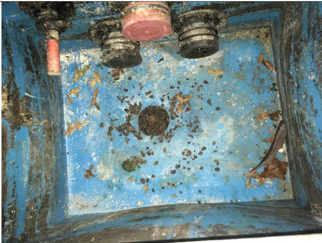
Photograph: 9 | Sump in building and sample location
