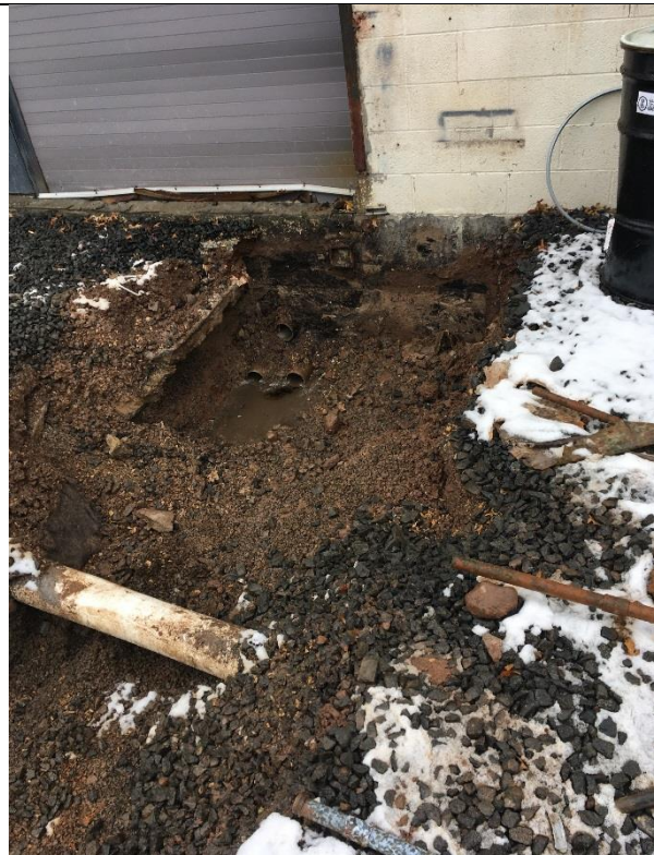
Photograph: 8 | Pipe entrance to building
