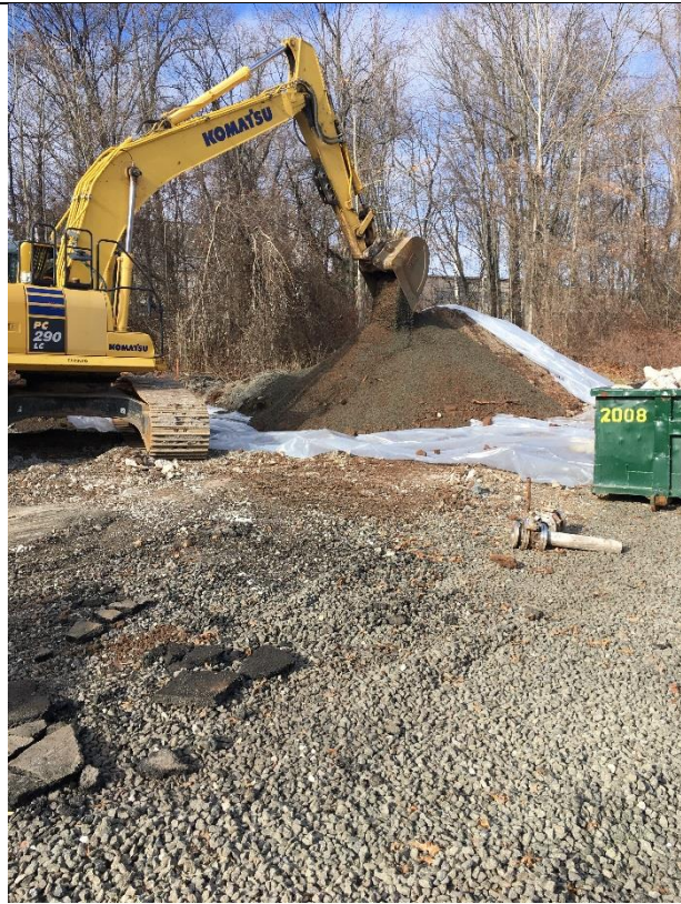
Photograph: 11 Temporary stockpile and backfill for re-use
