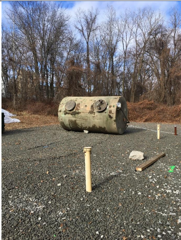
Photograph: 3 | Excavated tank
