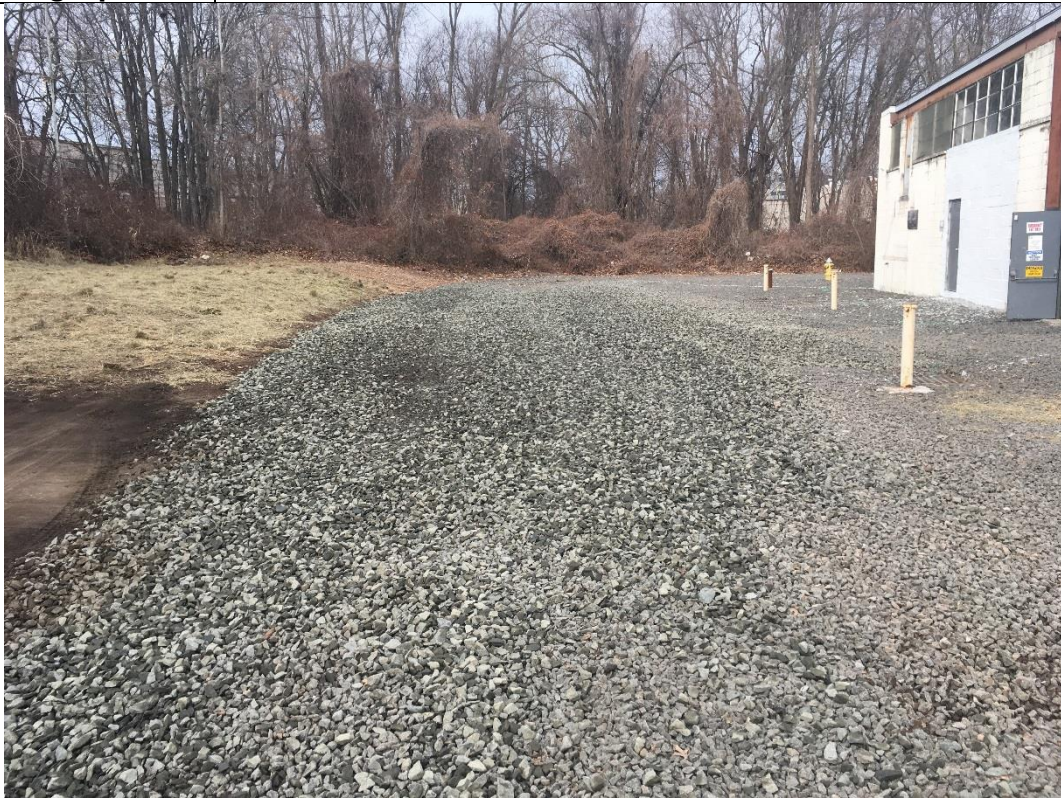
Photograph: 16 Site complete
