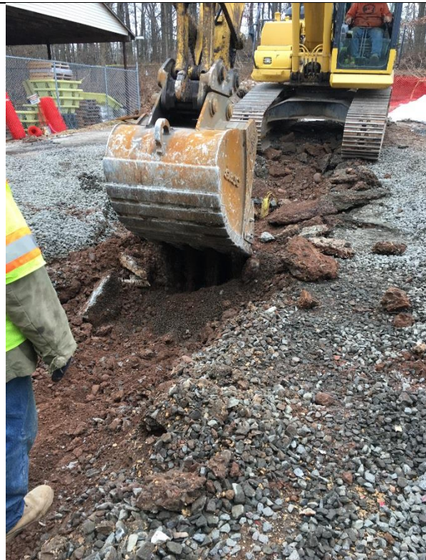
Photograph: 6 | Excavating pipe run
