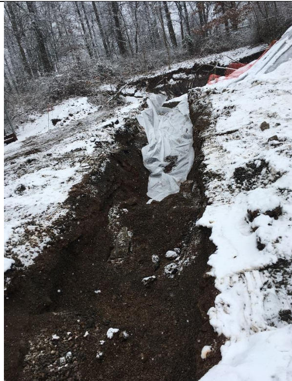
Photograph: 12 Pipe run being backfilled over demarcation layer
