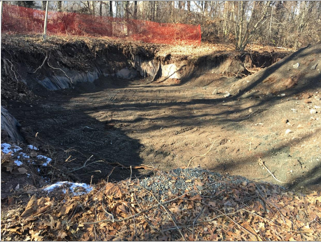
Photograph: 13 Backfill in tamped lifts
