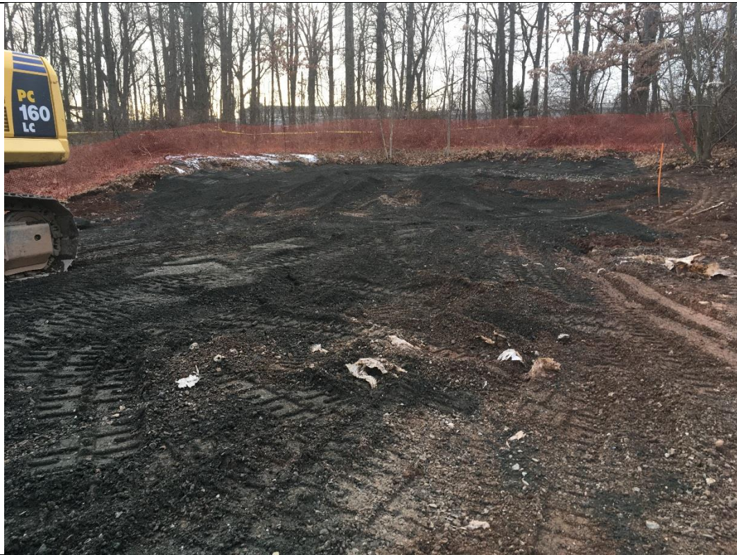
Photograph: 14 Topsoil over backfill
