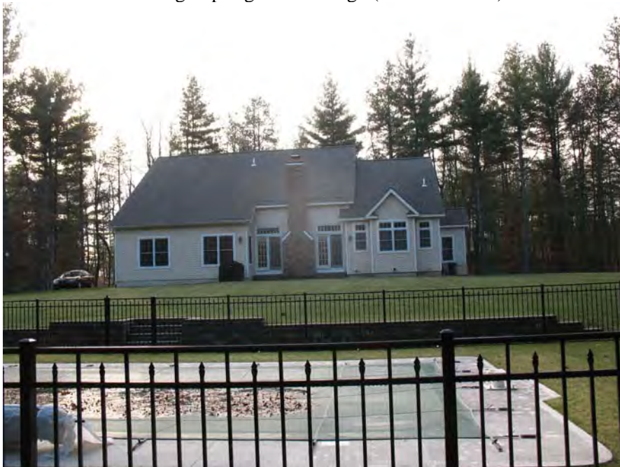
Photograph 2: View south from swimming pool at 15 Liz Ann Drive. Bullet shell casing were found in soil removed from excavation (5 December 2008) Saratoga Springs Rifle Range (RRNY000025)
