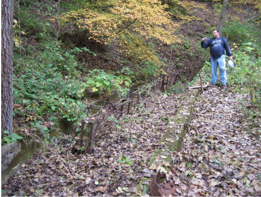
Photograph 7: Target butts with 4 iron target raising mechanisms, partially buried, for shorter distance rifle range (14 October 2008) Rochester Rifle Range (RRNY000024)
