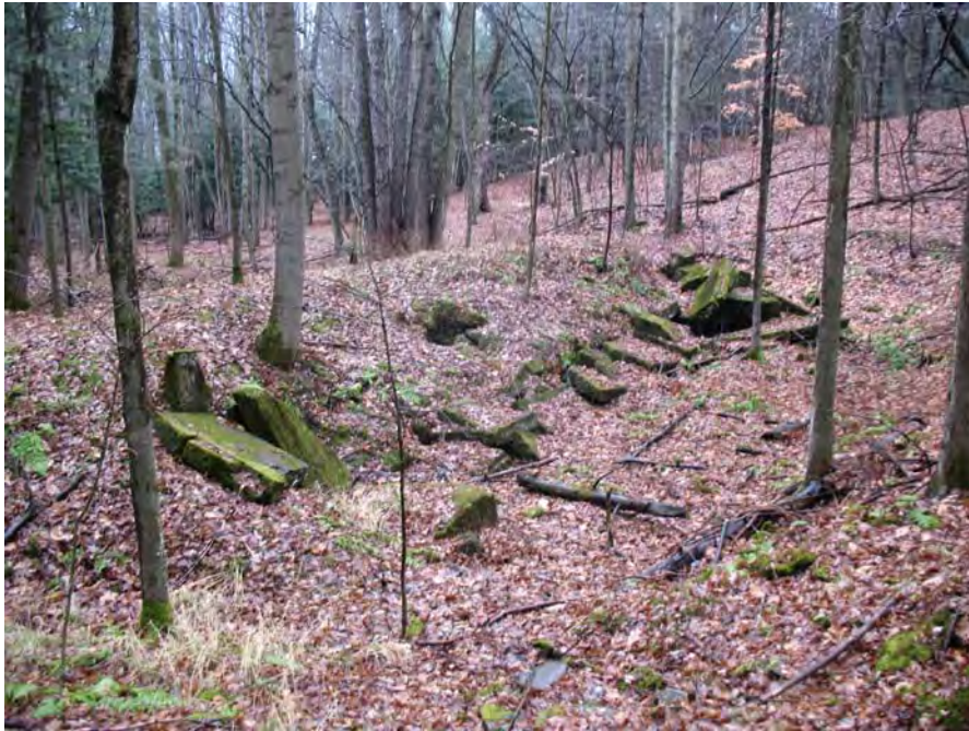
Photograph 1: View east of collapsed target berm wall (4 December 2008) Oneonta Rifle Range(old) (RRNY000021)
