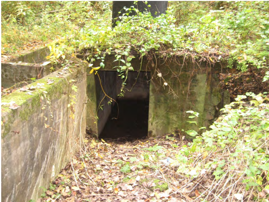
Photograph 7: Target butts with 4 iron target raising mechanisms, partially buried, for shorter distance rifle range (14 October 2008) Rochester Rifle Range (RRNY000024)
