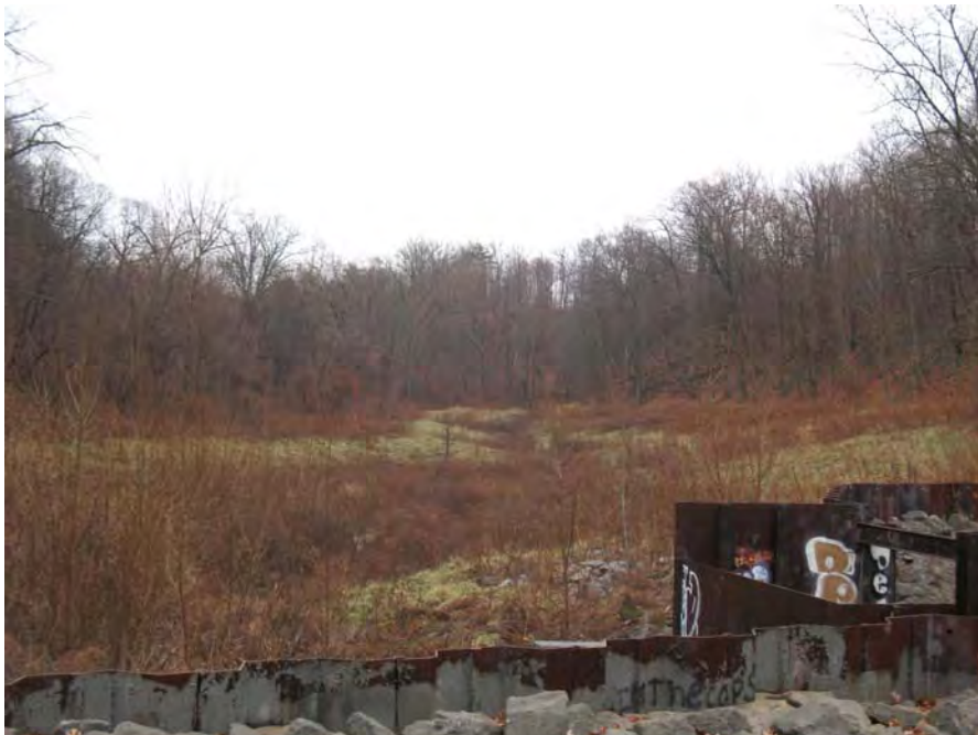
Photograph 4: View northeast, from the dam toward the target berm (10 December 2008) Rensselaer Wyck Target Range (RRNY000023)
