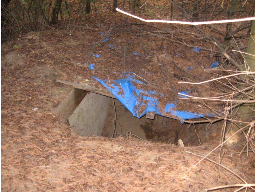
Photograph 1: Concrete target butt (15 October 2008) Glens Falls Rifle Range (RRNY000010)
