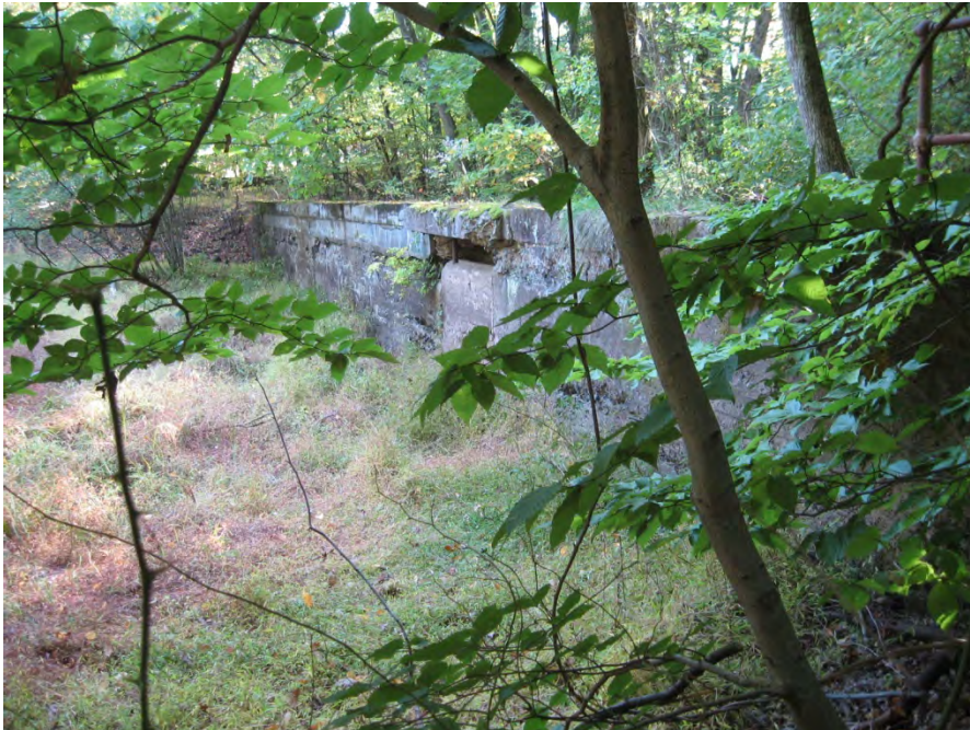
Photograph 4: Concrete dam near residence on Valenza Lane (9 October 2008) Camp Blauvelt (RRNY000003)
