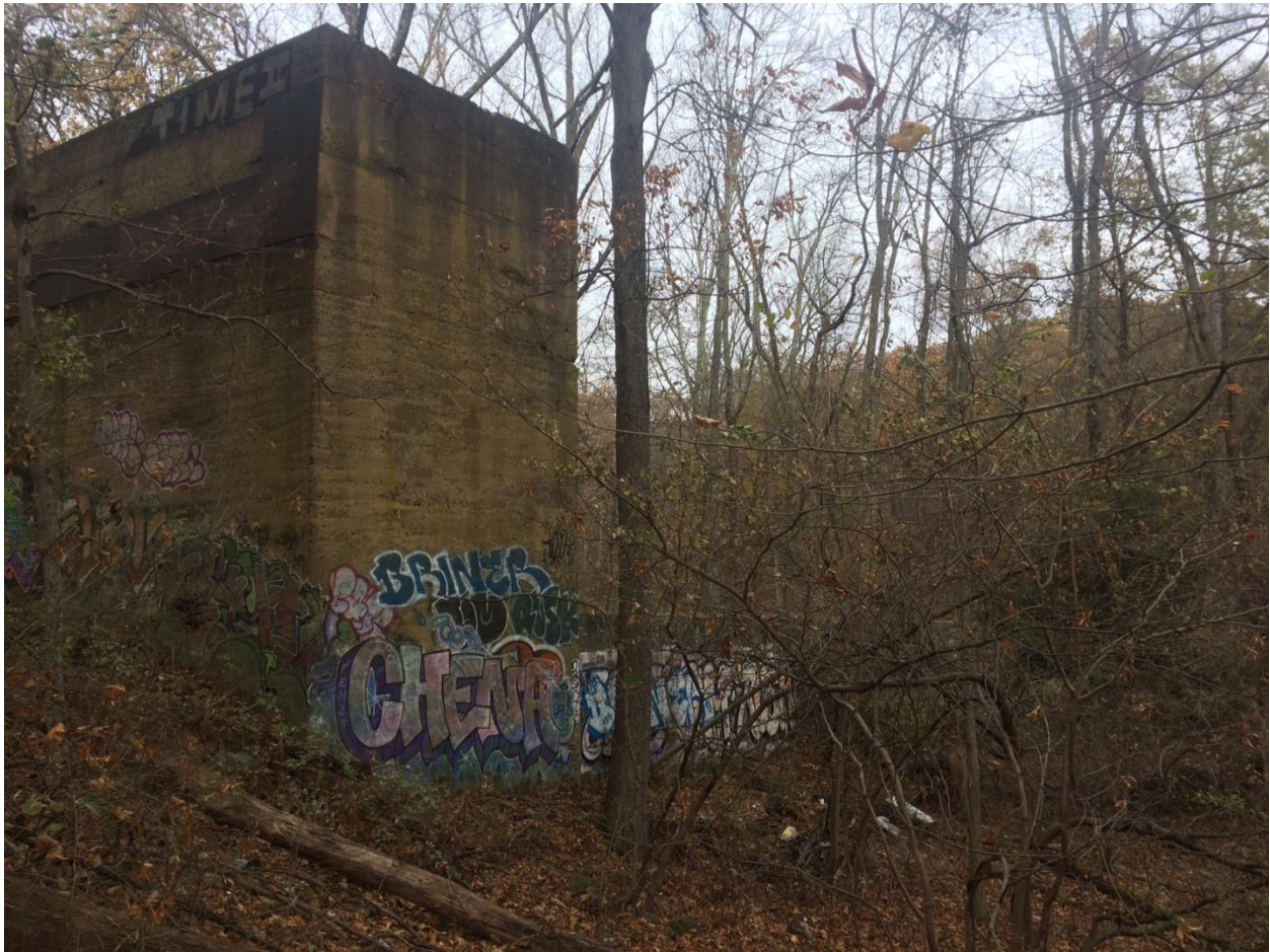
Photograph 4: View looking northeast towards the southern edge of the 600-yard target wall. A concrete tunnel begins at the base of the target wall and runs east up the hill away from the 600-yard target wall to the 1,000-yard wall. The lack of soil in front of the target wall is evident in this view.
