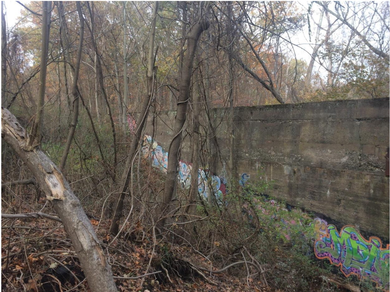
Photograph 3: View looking northeast at the front of 600-yard target wall. Thick vegetation covers the area in front the target wall. The range floor is eroded away directly in front of the wall. No soil was piled up against this target wall. The firing direction is from left to right in this field of view.
