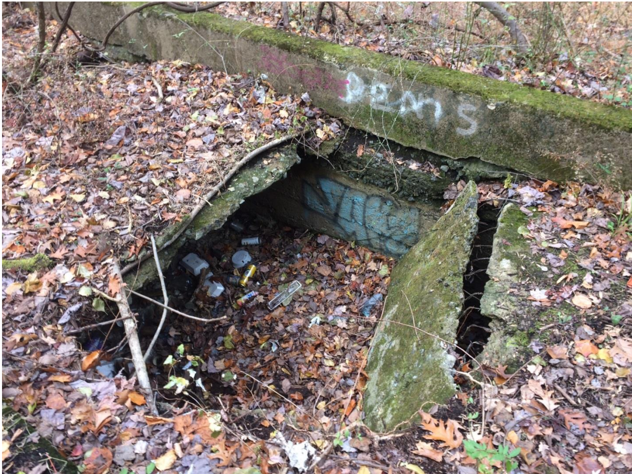
Photograph 9: Collapsed tunnel behind the 1,000-yard target. Belowground tunnels spanned the distance of the 1,000-yard target wall behind the wall in addition to the aboveground tunnels that connected the target walls at 600 yards and 1,000 yards.
