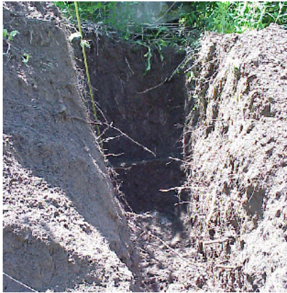
Photos shows limits of excavation Soil Pile 3, native soil at 7 feet below ground surface.
