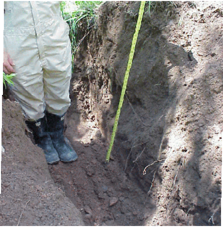
Photos shows limits of excavation at Soil Pile 2, native soil at 3.5 feet below ground surface.
