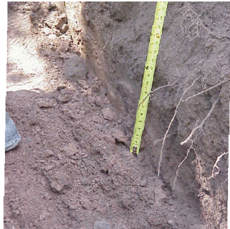
Photos shows limits of excavation at Soil Pile 2, native soil at 3.5 feet below ground surface.
