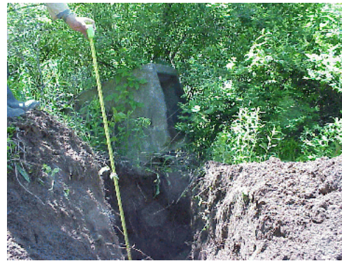
Photos shows limits of excavation Soil Pile 3, native soil at 7 feet below ground surface.
