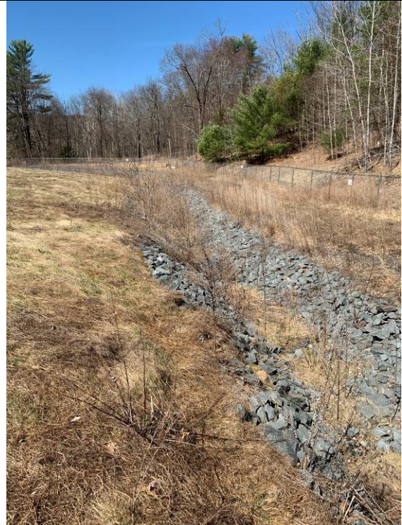
Photo 4: Looking west. View of the northern rip rap channel.
