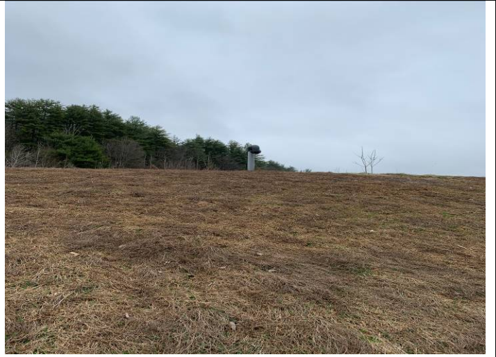
Photo 12: Looking northeast. View of a typical vent.
