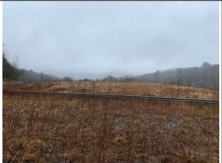
Photo 8: Looking east. View of the western cap slope.
