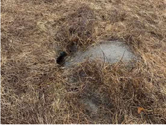
Photo 9: View of rodent burrow on western side of cap.
