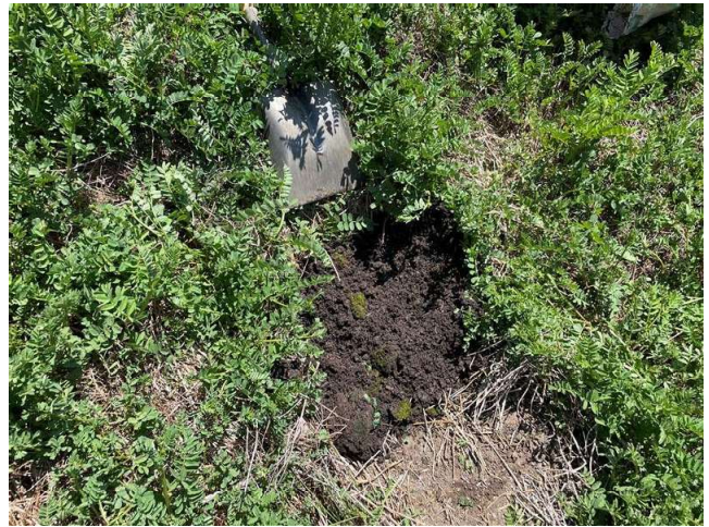
Photo #8: Photograph of the rodent hole after TRC filled in the hole with topsoil. Facing west.
