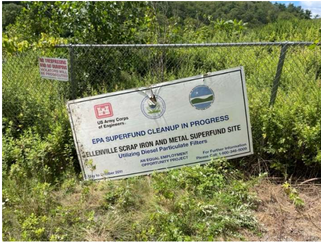
Photo #1: View of the entrance of the landfill. Sign is deteriorating and will need replacing, facing SW.
