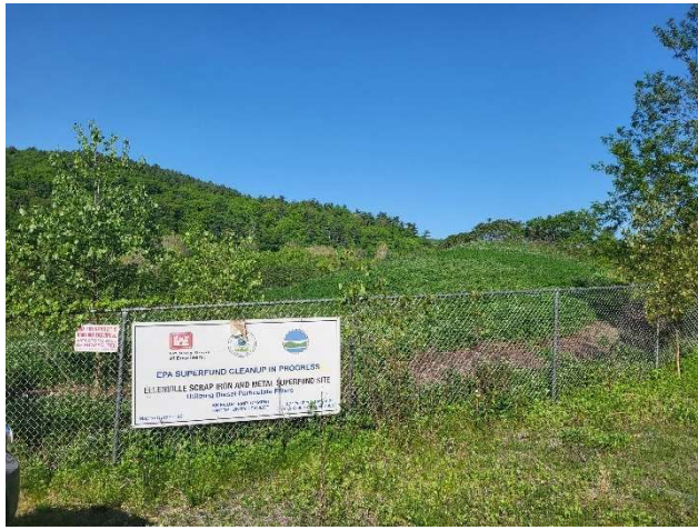
Photo #1: View of the entrance of the landfill, facing northwest.
