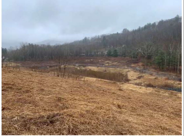
Photo 10: Looking east. View of the southern cap slope and detention basin.
