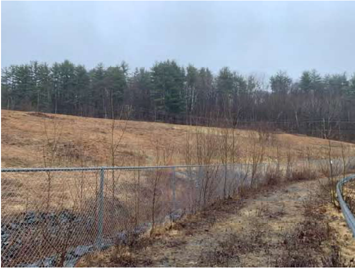
Photo 5: Looking north. View of the eastern landfill hillside and access road.
