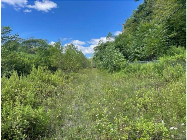
Photo #2: View of vegetation and saplings present within the northern drainage channel, facing west.
