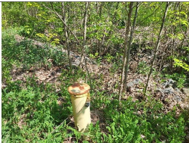
Photo #5: View of EPA-09, which was in good condition, facing north.
