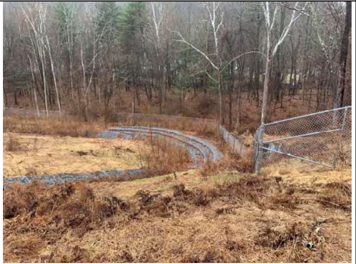
Photo 12: Looking south-southwest. View of the drainage channel and gabion wall.
