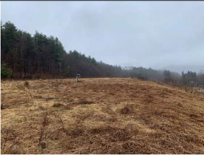
Photo 11: Looking east. View of the landfill cap and vents.
