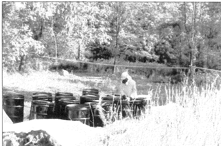
Photo 2. Pumping out tank into drums in staging area. (9-24-97)
