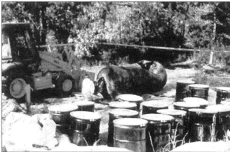
Photo 7. Tank opening after removal to complete cleaning. (9-24-97)
