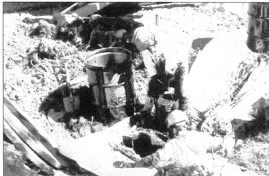
Photo 4. Hand removal of sludge. (9-24-97)
