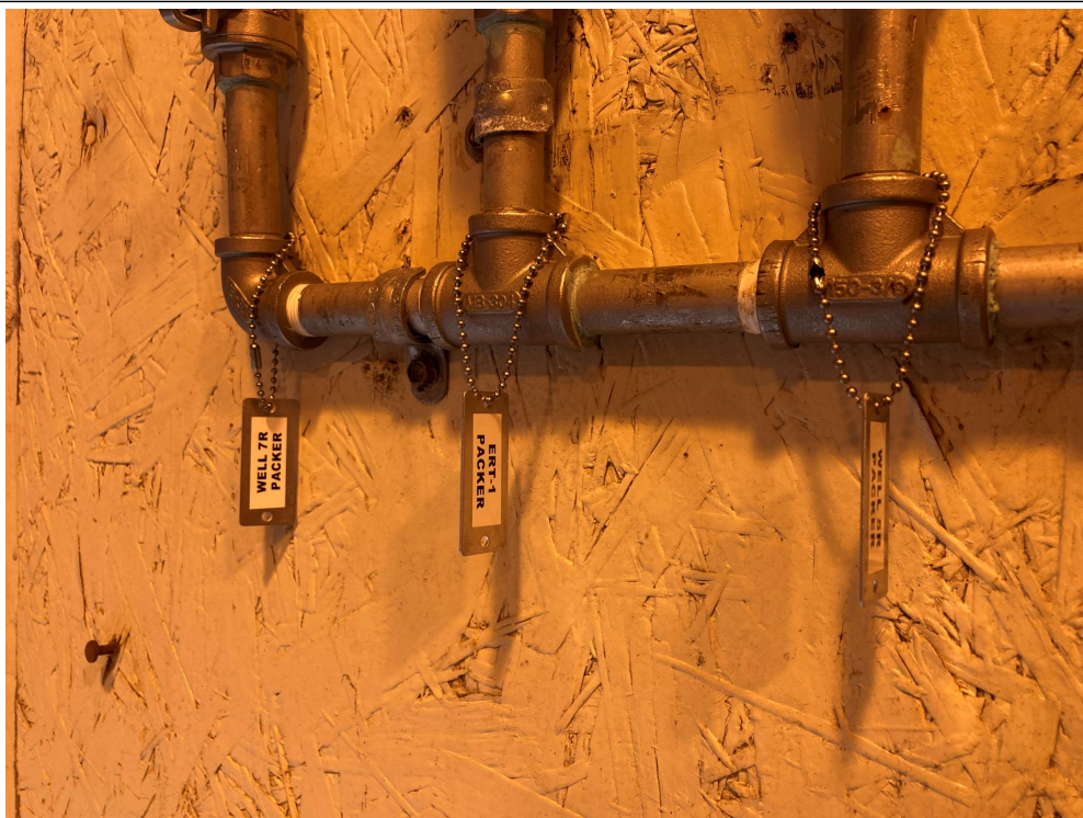
Photo 10: Nitrogen Supply Manifold.
