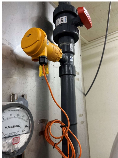
pH sensor shown following reinstallation into the line
