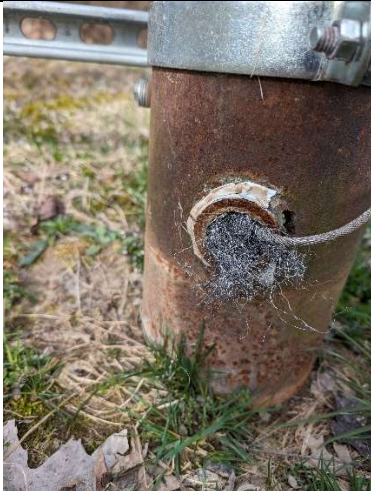
Steel wool used to deter rodents that might want to enter (covered after photo taken).
