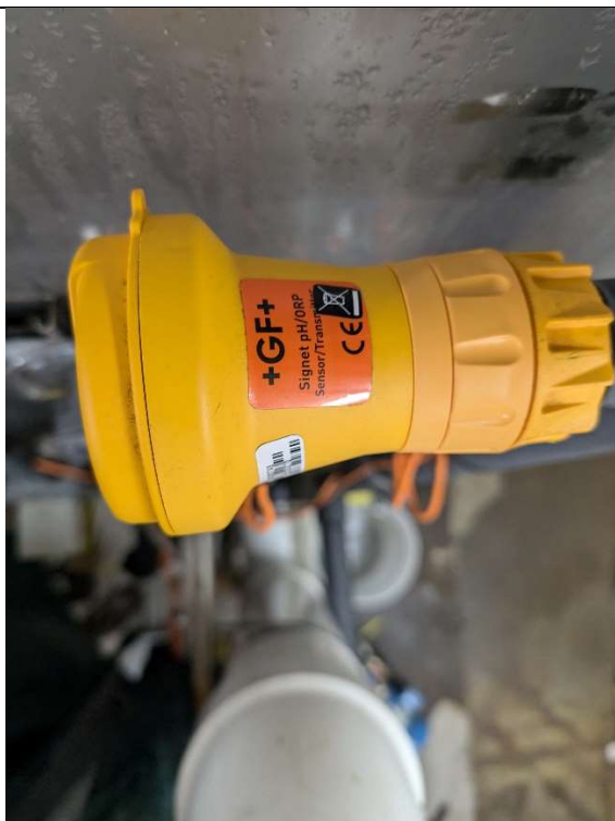
New pH electrode installed
