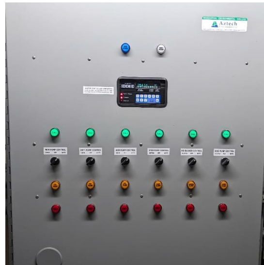
Main Control Panel with Hand/Auto/Off Switches
