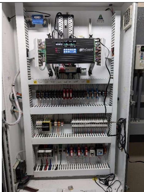
Panel box that sends VFDs commands
