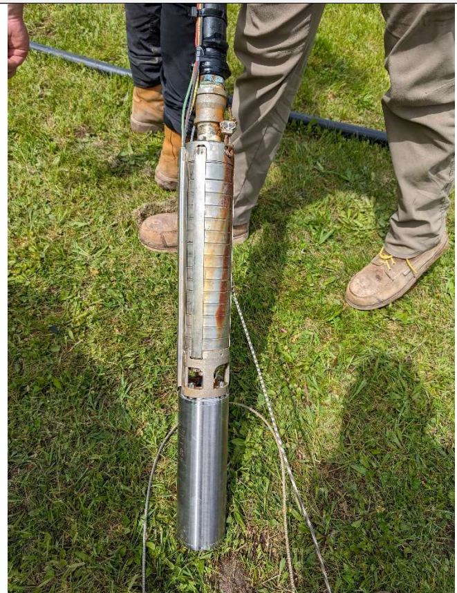
New motor attached to existing pump.
