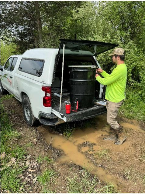
Tightening drum containing purged SVE water prior to transport to the GWETS
