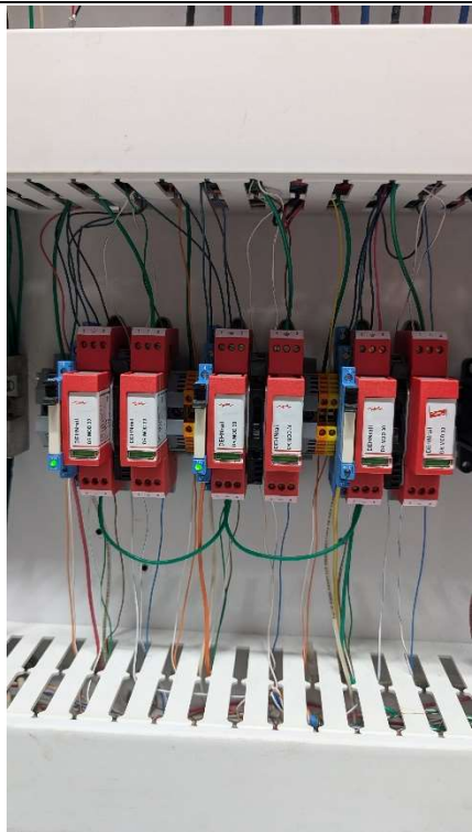
New Surge Suppressors installed (red devices)
