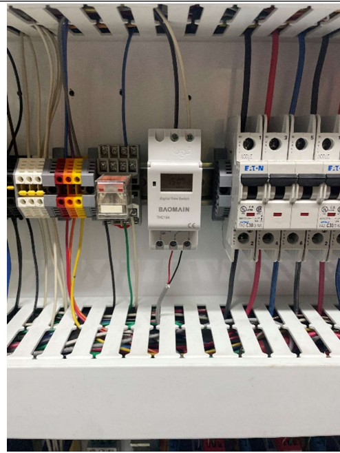
Time delay relay switch installed
