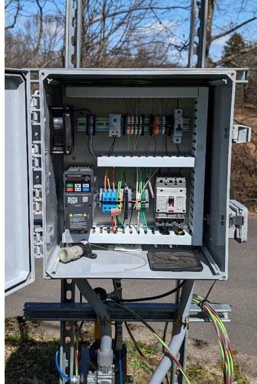
MW-5R pump leads removed ready for motor replacement.
