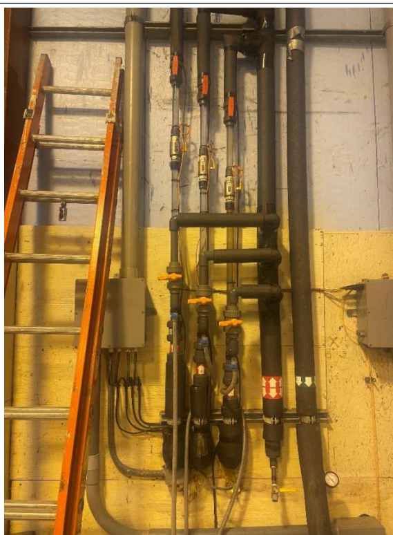
Flow meters of recovery wells.
