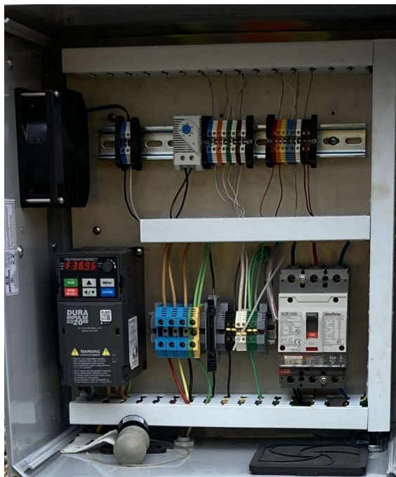
Photo 12: Wellhead Electrical Upgrades – Panel Box Closeup (VFD – Bottom Left)
