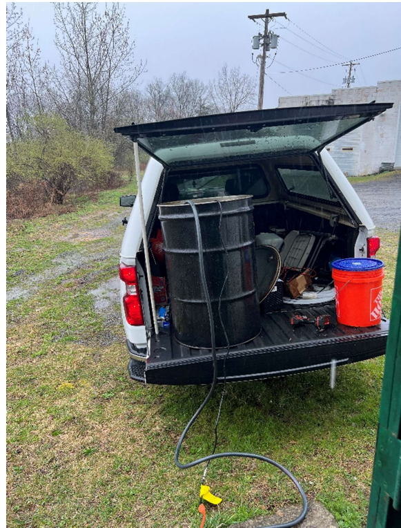
-Pumping water out of barrel used to contain water from the wells.
