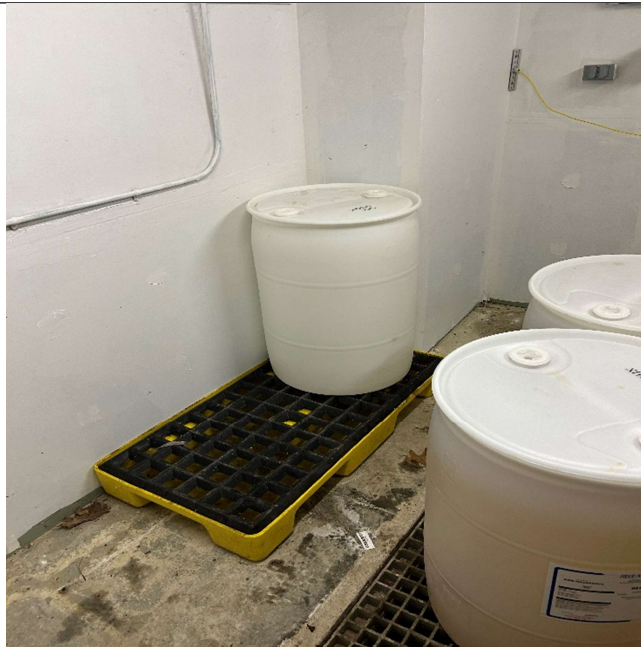
View of empty drum on containment after transferring the rest of chemical contents into the active pumping drum
