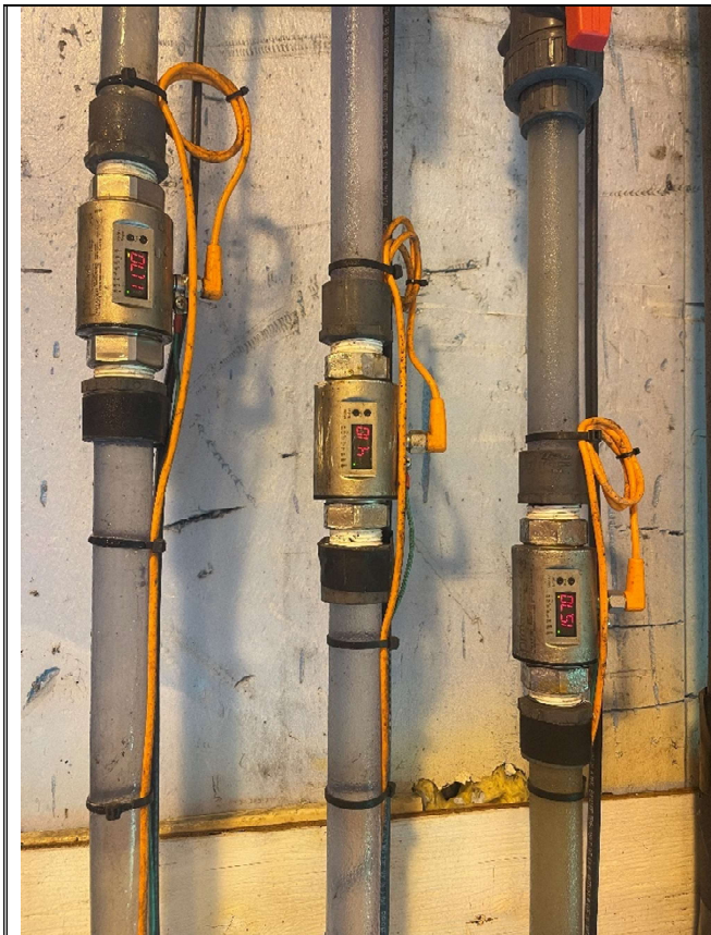
Flow meters of recovery wells.
