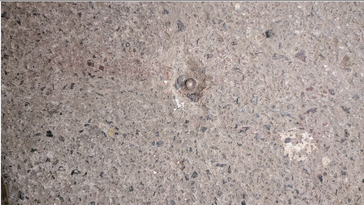
Photo 2: Vapor point for Mohonk SSDS system
