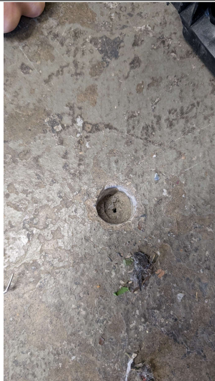
Photo 10: SGP-11 is damaged. Vacuum = 0.028 inWC
