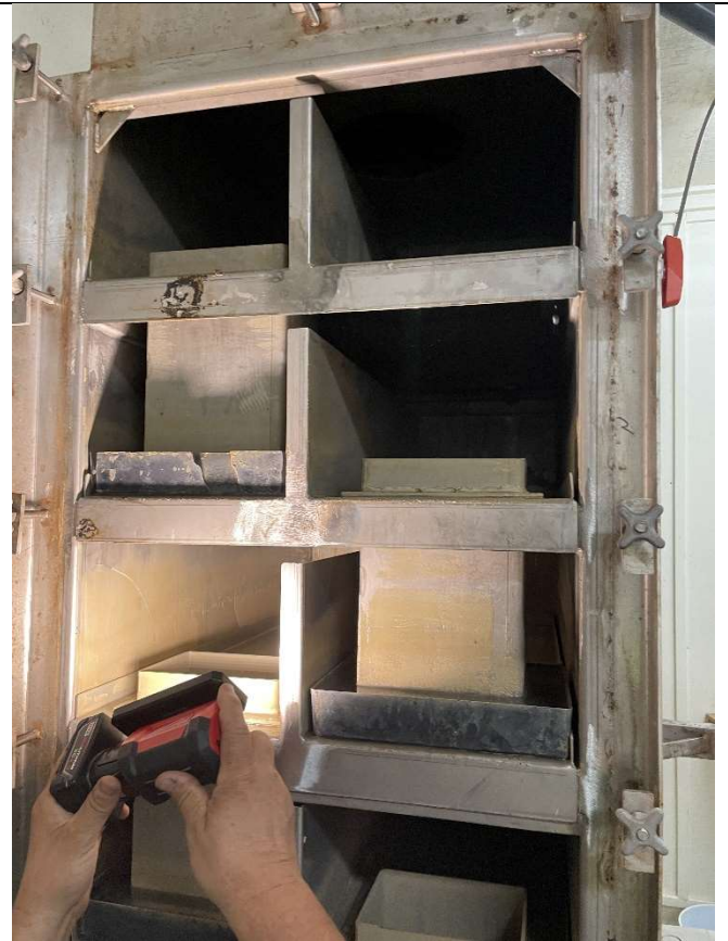
Air Stripper maintenance
