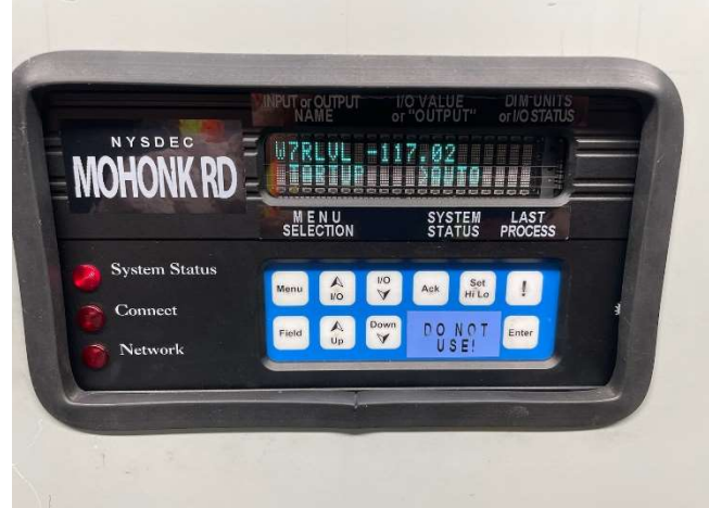
Level in Recovery Well 7R reading as -117' bgs.
