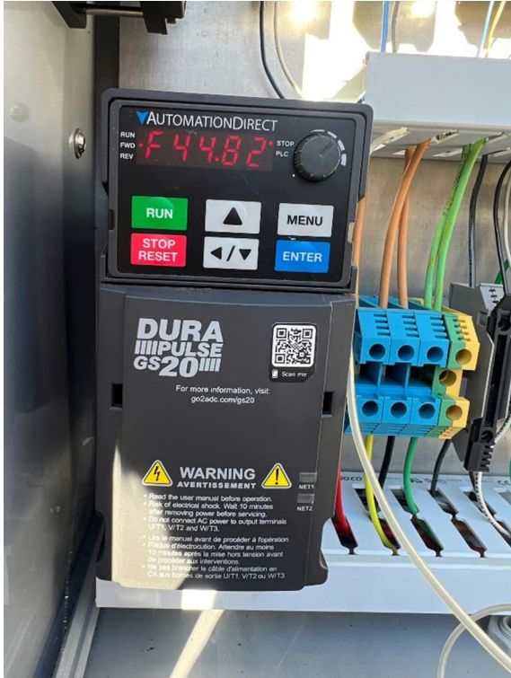
VFD in the RCP is powered up, getting a “forward” speed control signal of 45+/- hz but not getting a “run” signal from the main control panel (MCP).
