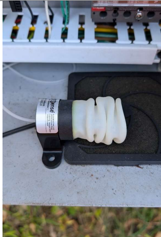
New Bellows installed at each extraction well
