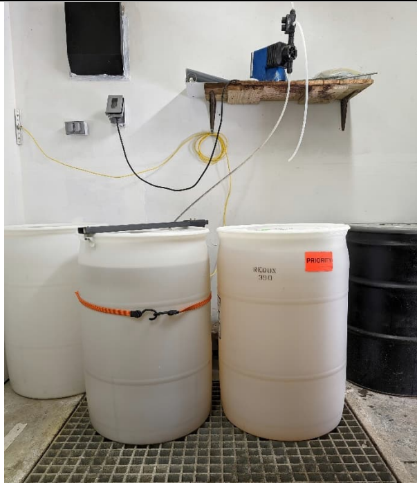
Two Full Redux Drums (One In Service)
