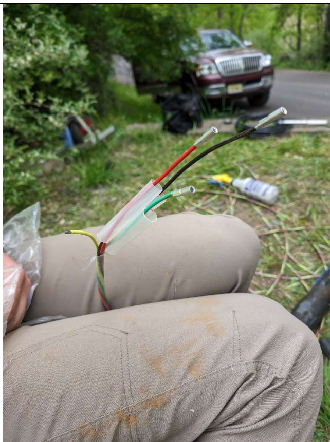
Pump motor wires being spliced.
