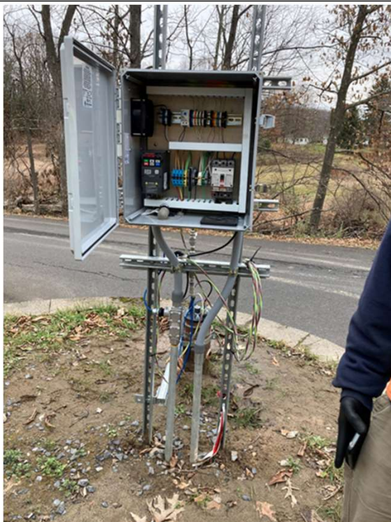
Photo 12: Wellhead Electrical Upgrades – Panel Box Closeup (VFD – Bottom Left)
