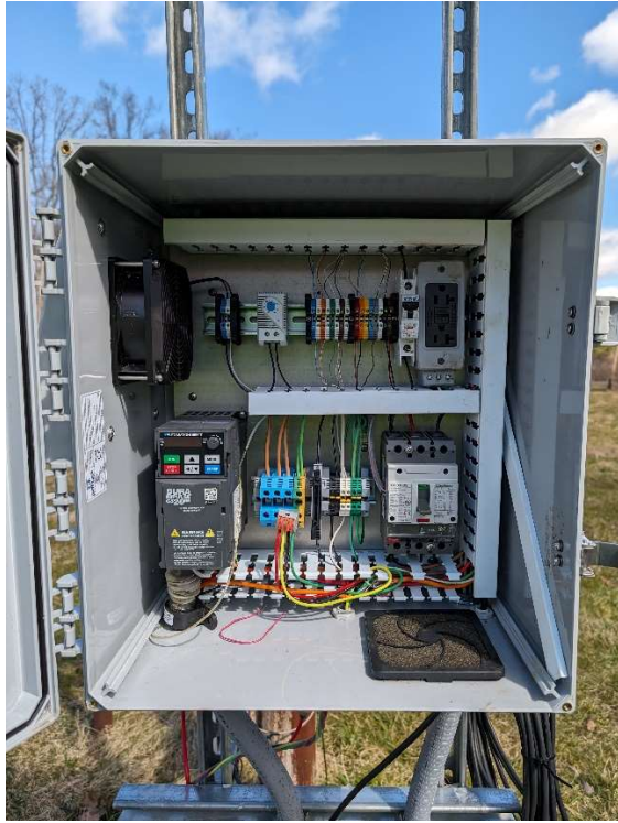
ERT-1 pump leads removed ready for motor replacement. The VFD in the lower left of the box also needs to Be replaced. Error code b4GEFF.
