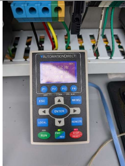
Tool used by TB to program VFDs at ERT-1 & MW-5R
