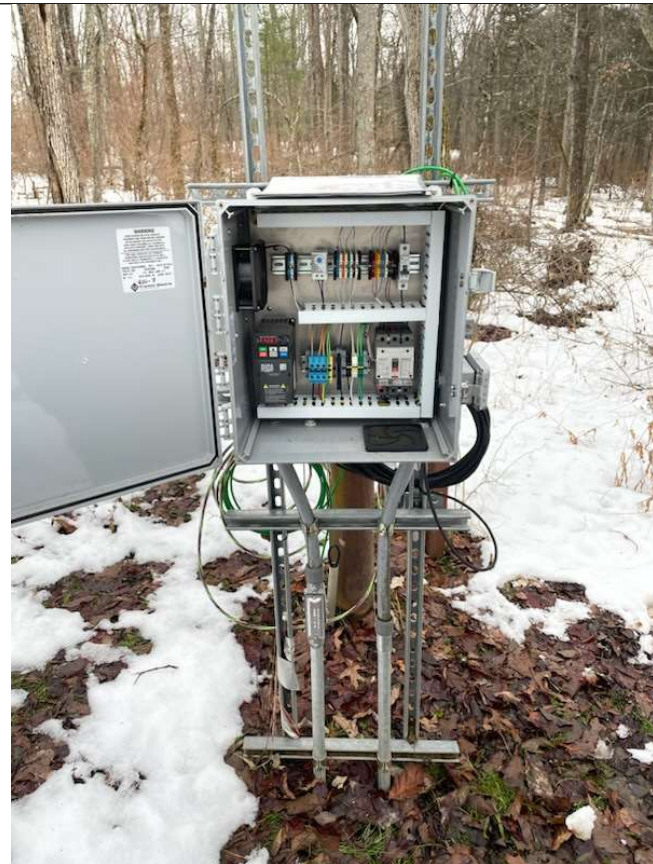
Panel box at 7R found dry and undamaged.
