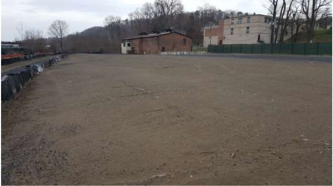
Photograph 29: Photograph facing northwest following the installation of the protective site cover.
