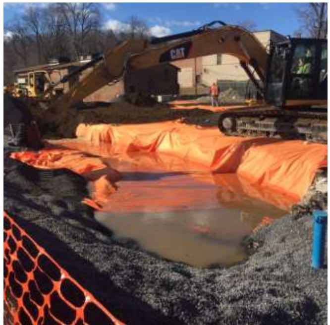
Photographs 18, 19, & 20: A demarcation layer consisting of construction fencing and/or filter fabric was placed above existing site soils and covered with imported backfill. Photographs facing northwest.
