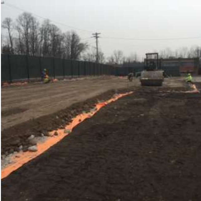
Photographs 21 and 22: A protective site cover consisting of imported soil (left) or imported stone product (right) was installed over the footprint of the site.
