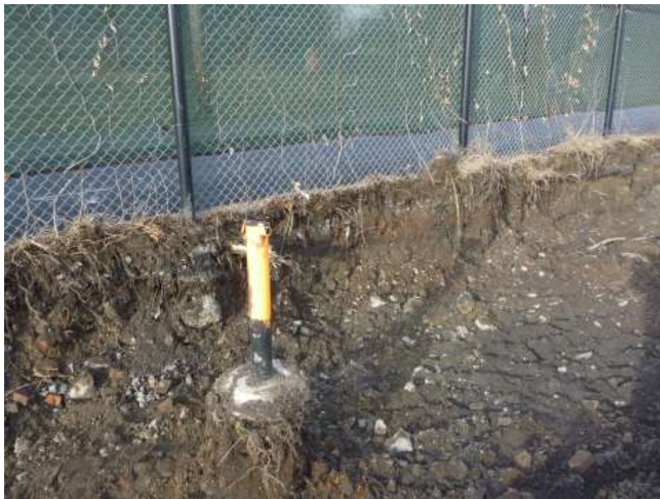
Photograph 13: The area surrounding MW-13 (photocenter) was excavated by Ulster Excavating to locate well MW-3. No evidence of MW-3 was observed and is presumed to have been previously removed.
