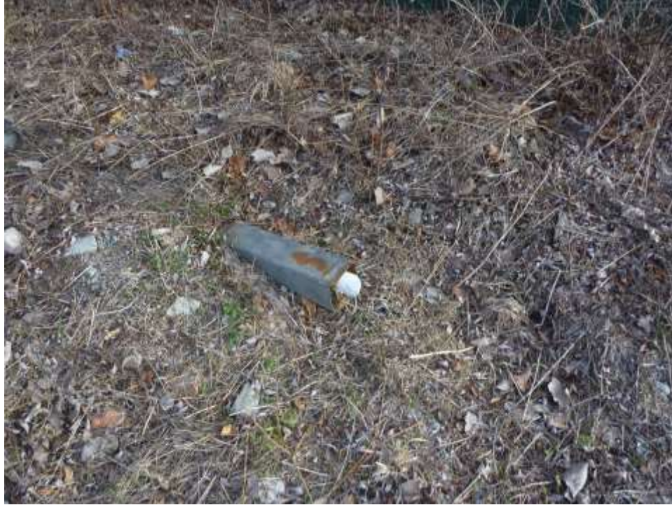
Photograph 12: Monitoring Well MW-4R, adjacent to MW-11, was observed during IRM field activities to be irreparably damaged and was subsequently decommissioned by ADT in accordance with CP-43.
