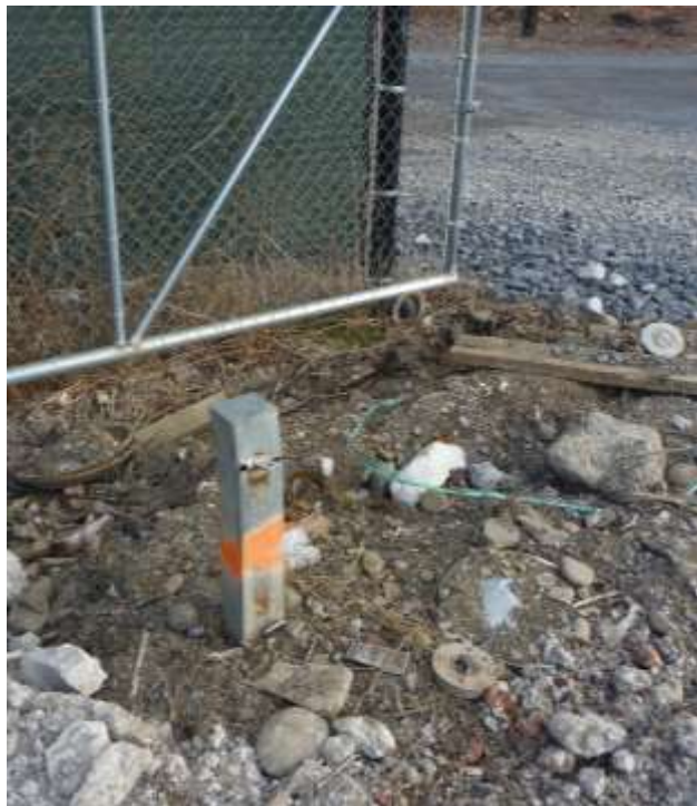
Photographs 23 and 24: Monitoring Well MW-10 was damaged during the installation of the protective site cover.
