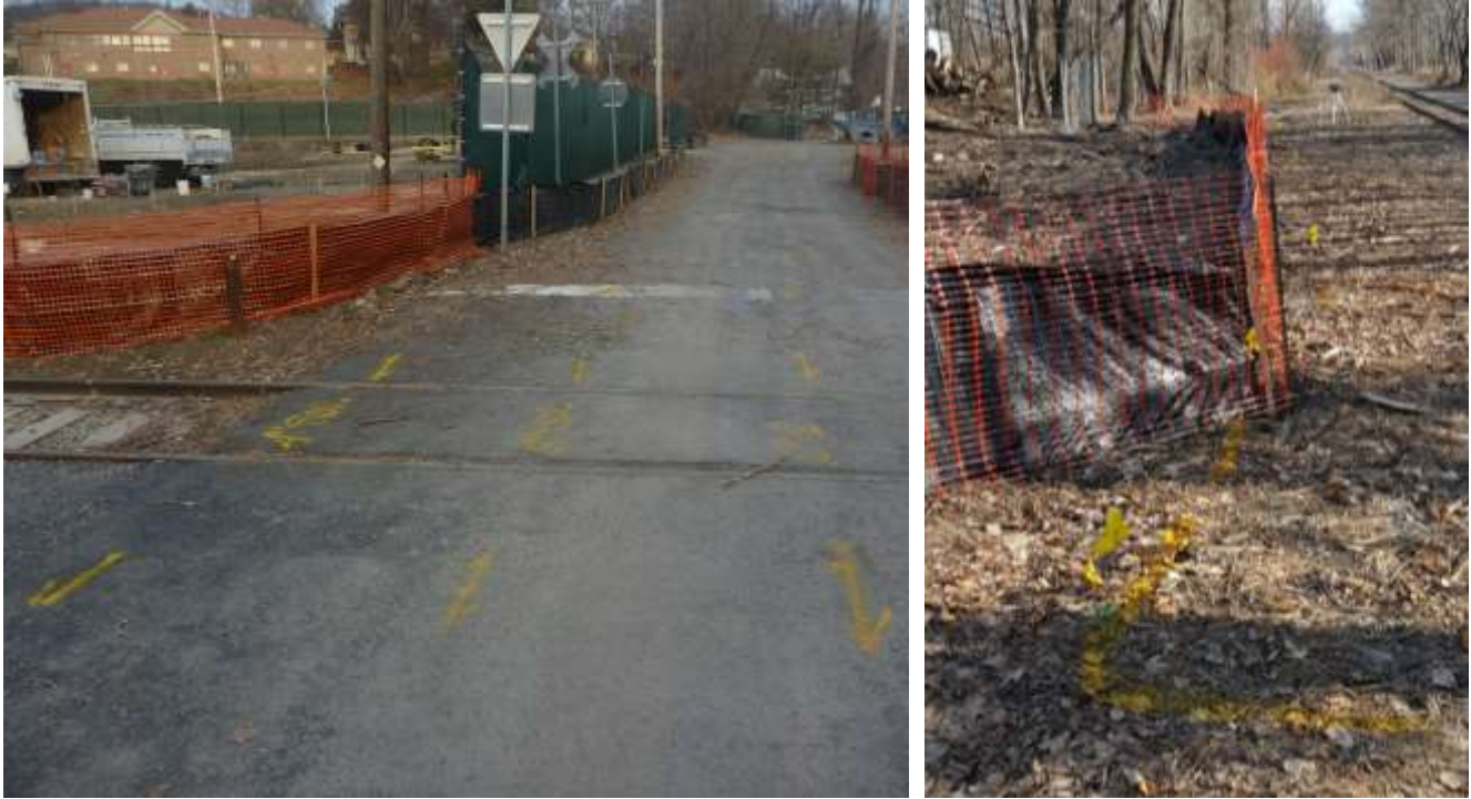
Photographs 1 & 2: Underground utilities were marked with spray paint and flags during site preparation activities and prior to ground intrusive activities.
