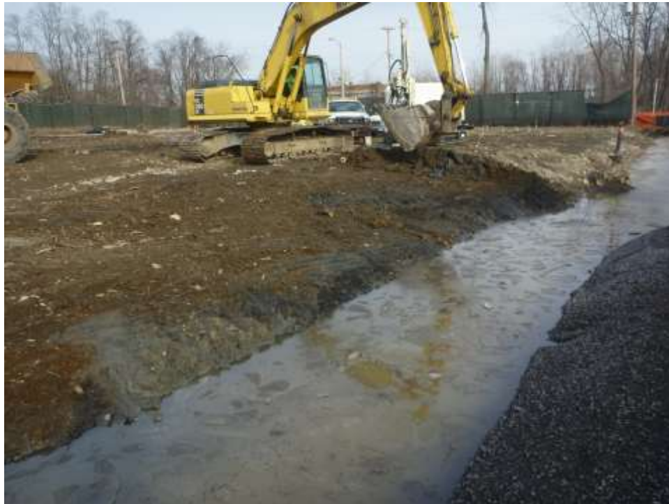
Photograph 15: Visibly stained soil was excavated spanning approximately 80 feet east-west and 20 feet north-south near MW-14 (shown far right). Photograph facing northeast.
