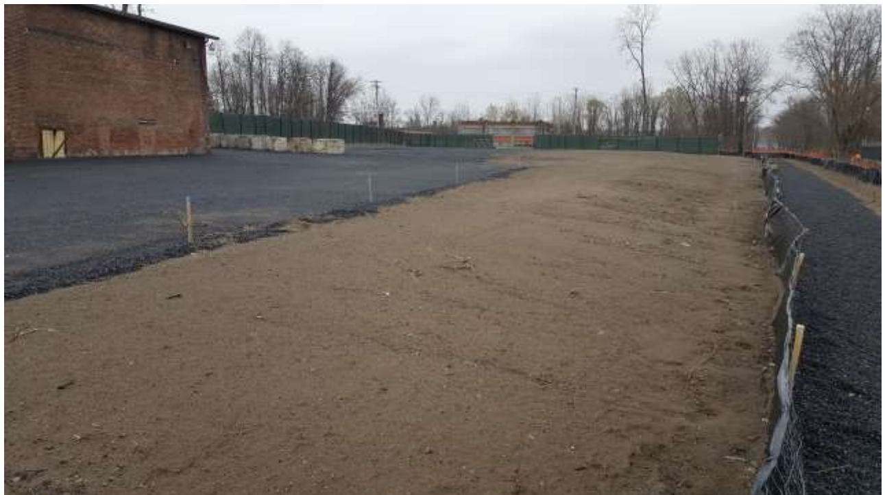
Photograph 28: Photograph facing northeast following the installation of the protective site cover.
