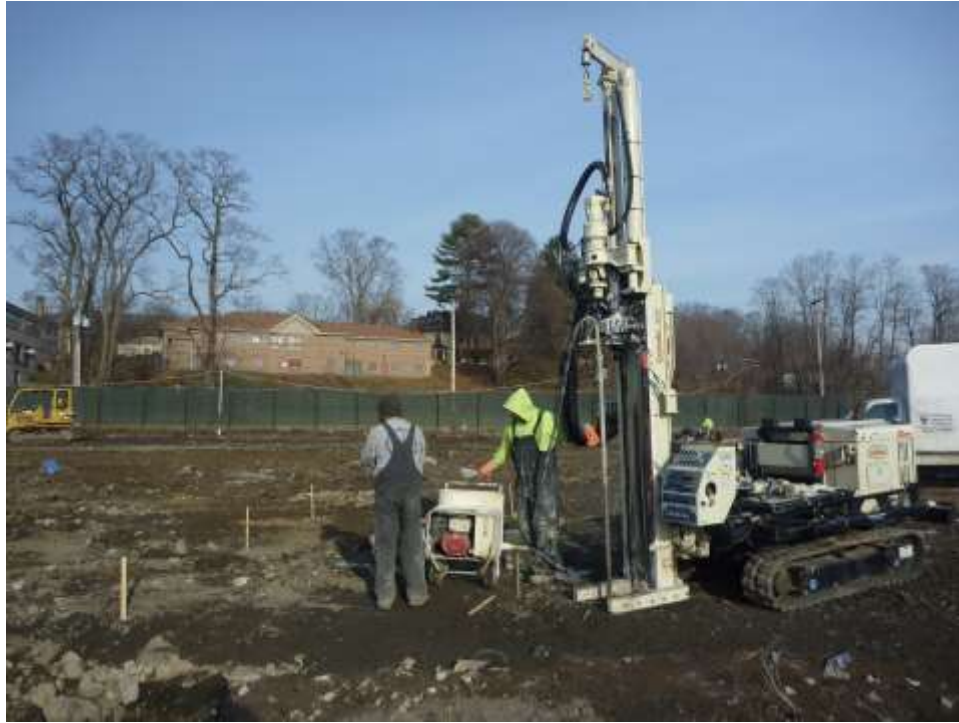
Photograph 8: Aquifer Drilling & Testing, Inc. (ADT) performed mixing and injection of ORC.
