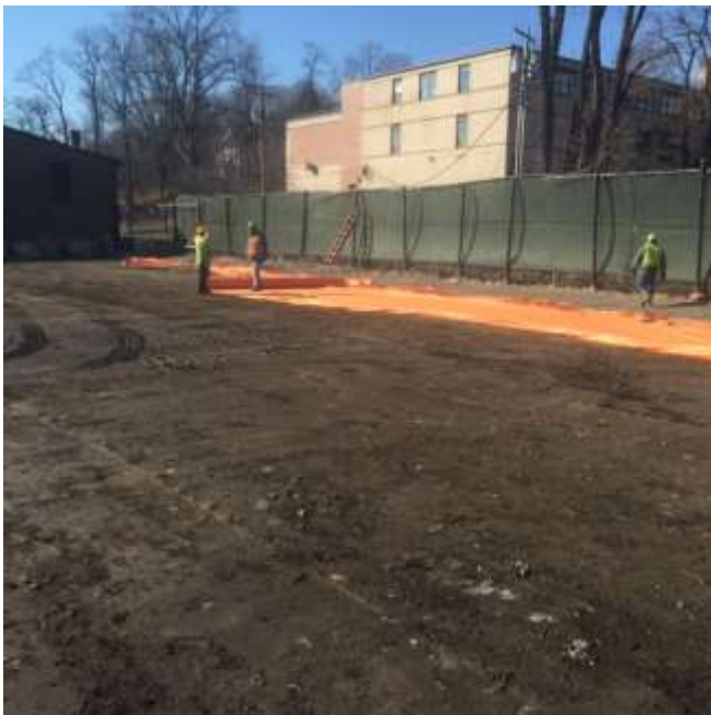
Photographs 18, 19, & 20: A demarcation layer consisting of construction fencing and/or filter fabric was placed above existing site soils and covered with imported backfill. Photographs facing northwest.
