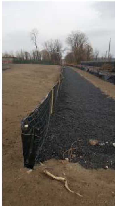
Photograph 30: Stormwater control ditch following completion, facing east.
