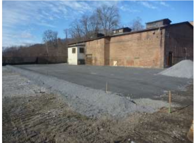
Photographs 21 and 22: A protective site cover consisting of imported soil (left) or imported stone product (right) was installed over the footprint of the site.
