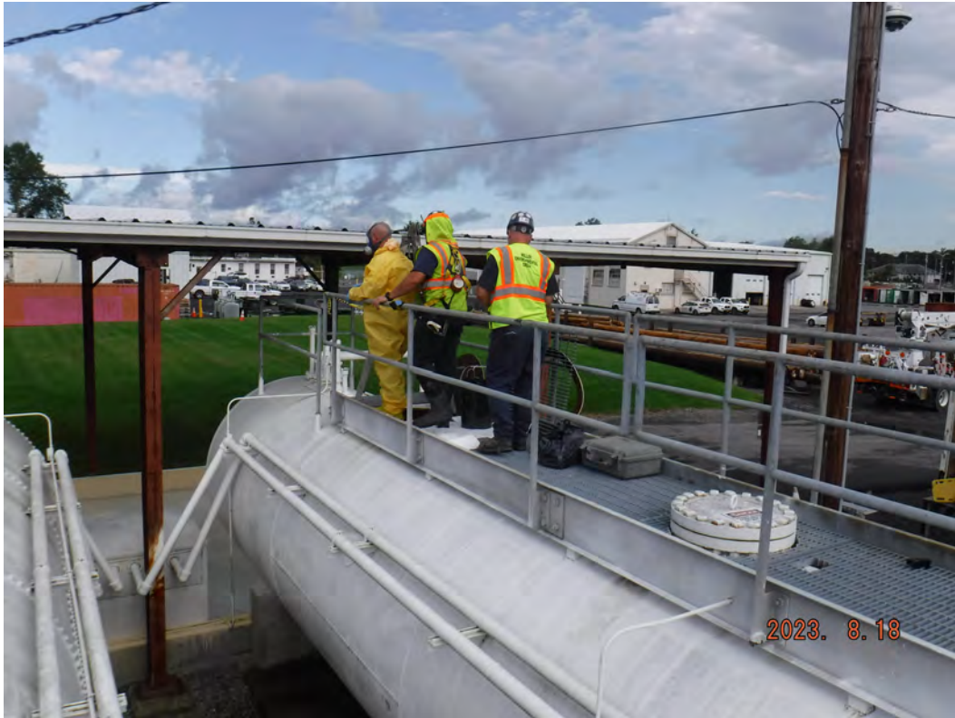
CONFINED SPACE ENTRY INTO 6,000-GALLON AST
