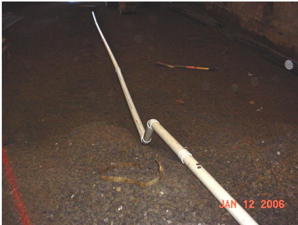
Photo 1 - Installation of 81 Broadway sub-slab depressurization system piping.
