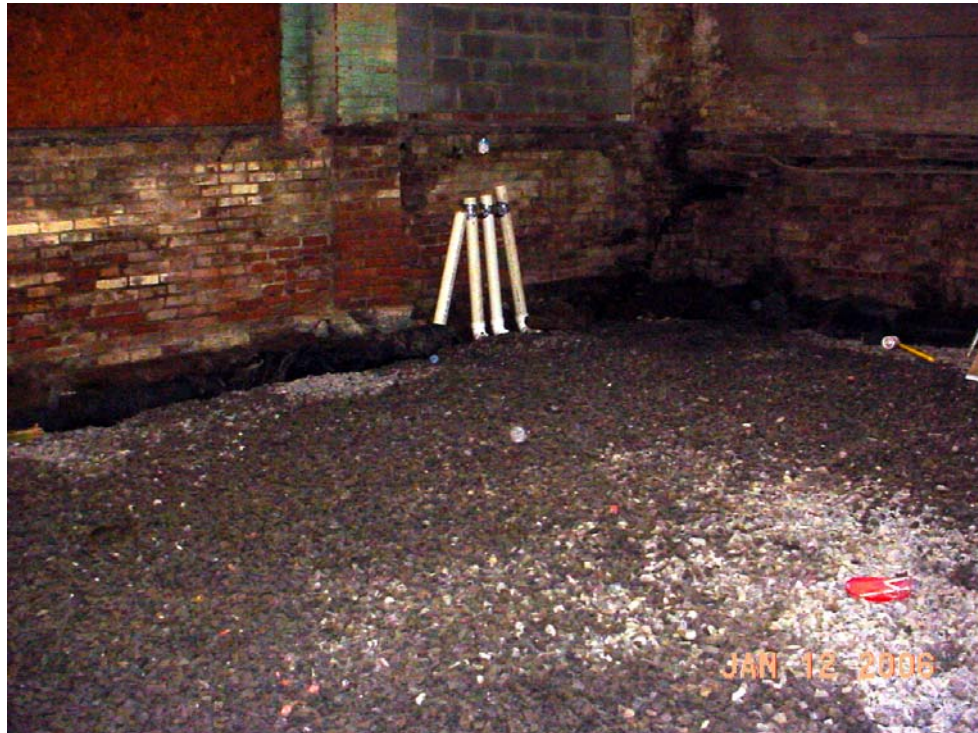
Photo 6 - Gravel placed over SSD piping.
