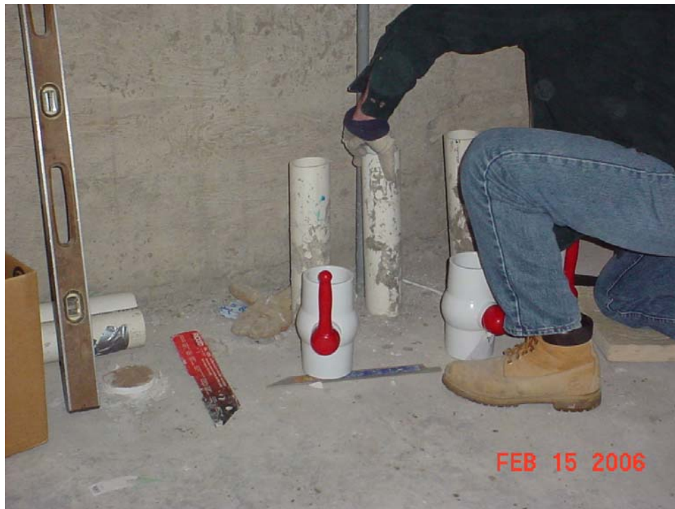
Photo 9 - SSD piping rising out of concrete floor.
