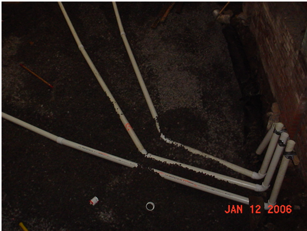
Sub slab piping with risers to valve bank.
