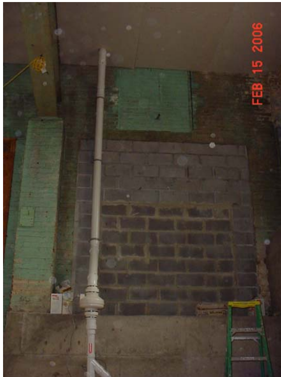
Photo 14 - Completed riser through ceiling.
