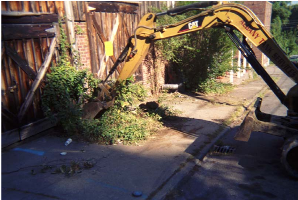
Photo 1 - Excavating to locate USTs below sidewalk in front of 38 Post Street.
