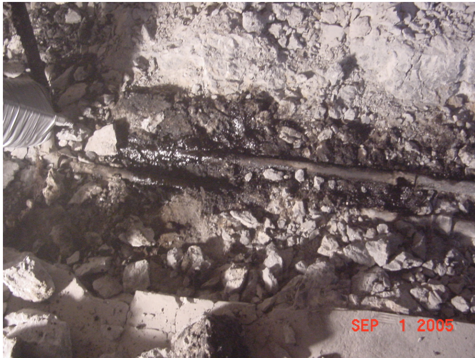
Photo 3 – Oily piping in concrete floor of 38 Post Street.
