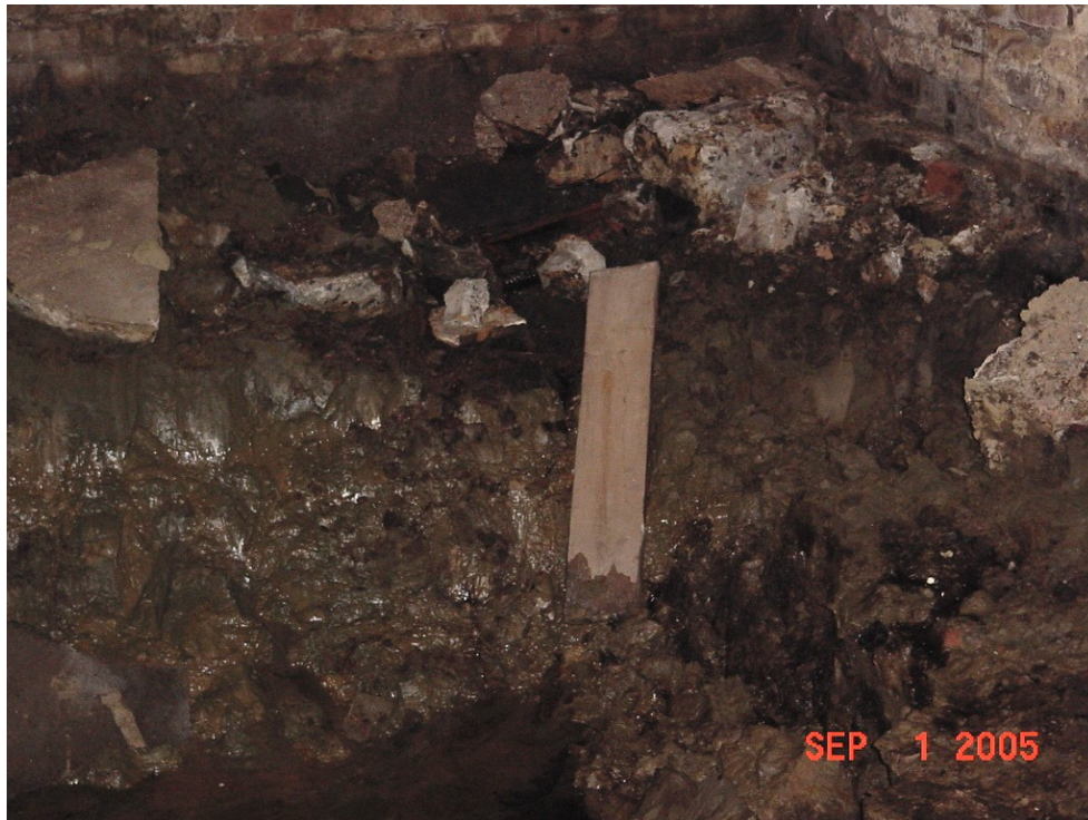
Photo 1 - Oily water seeping into 81 Broadway along southern wall foundation discovered after concrete floor was removed.
