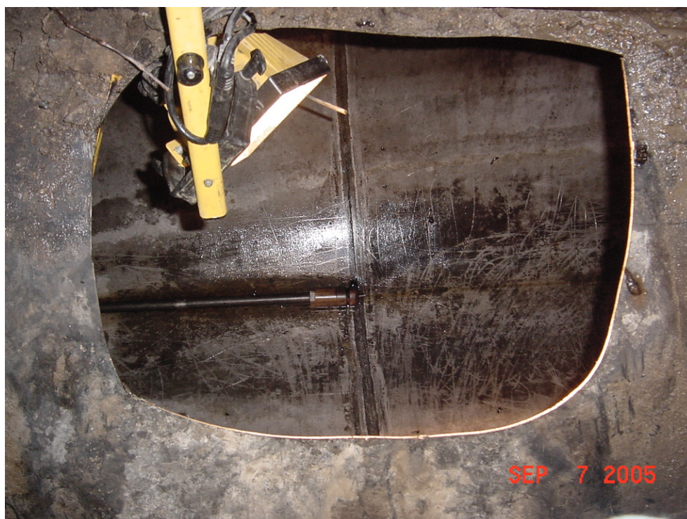
Photo 4 - 1,500 gallon UST opened and cleaned.
