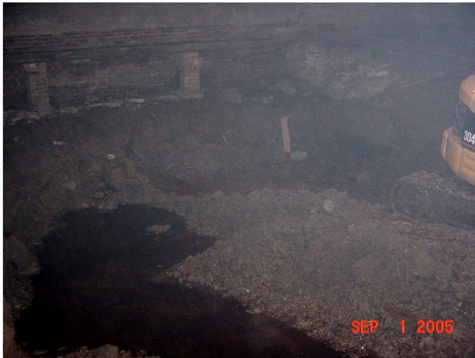
Photo 2 - Accumulated water and oil impacted soil inside 81 Broadway after concrete floor was removed.
