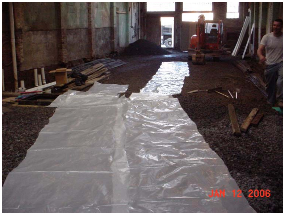
Photo 7 - Preparation for laying out polyethylene sheeting over gravel prior to pouring concrete.
