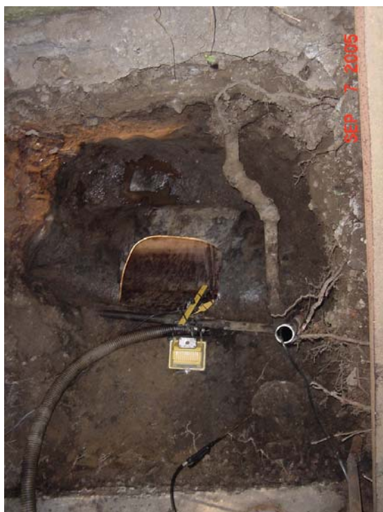
Photo 3 - Uncovered 1,500 gallon UST behind 38 Post Street.
