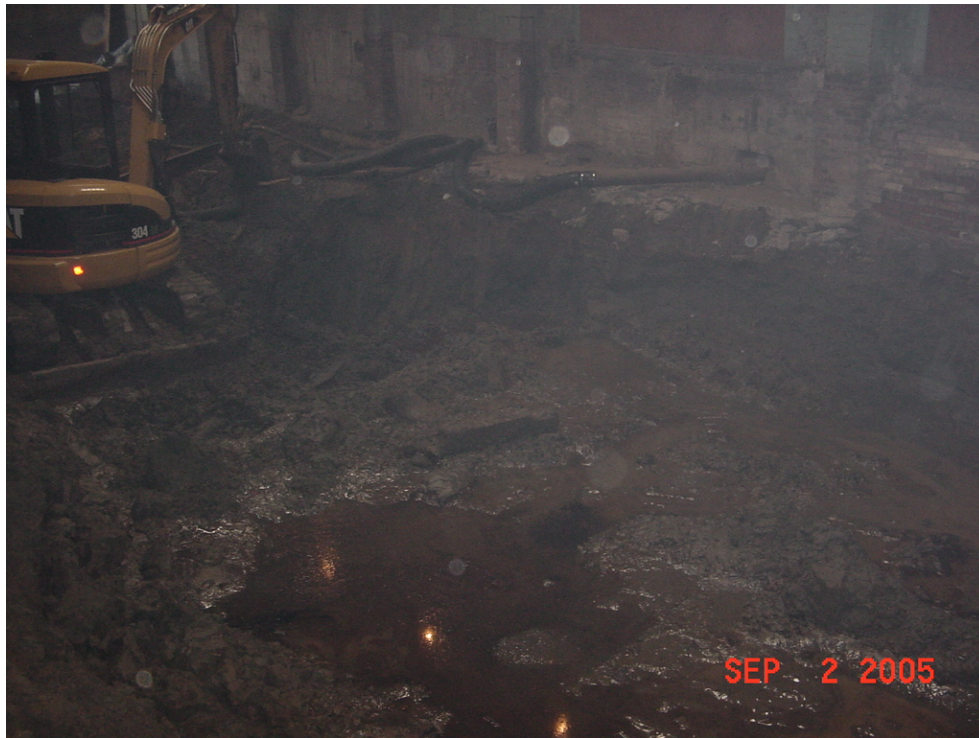
Photo 3 – Primary area in southern portion of 81 Broadway where oil impacted soil and accumulated water were removed from 81 Broadway.
