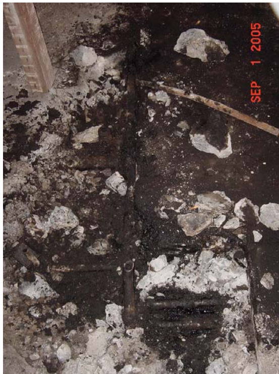
Photo 5 - Oily piping below concrete in 38 Post Street basement.
