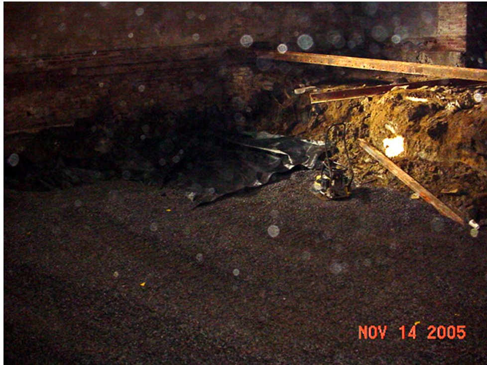
Photo 8 - Gravel layer in excavation inside 81 Broadway.
