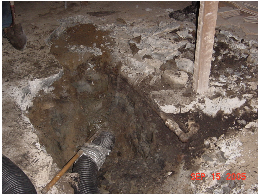
Photo 6 - Concrete and soil excavation in 38 Post Street basement.
