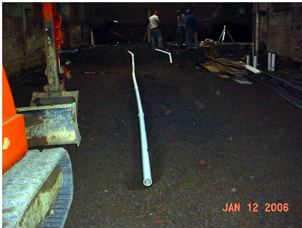
Photo 5 - Installation of 81 Broadway sub-slab depressurization system piping.
