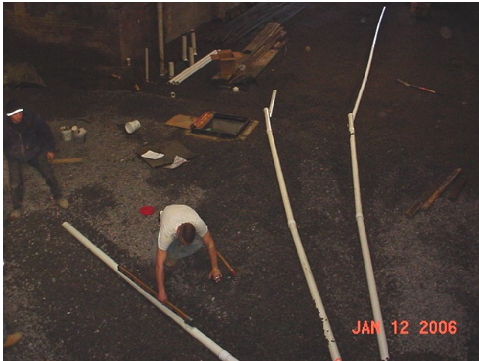
Photo 4 - Installation of 81 Broadway sub-slab depressurization system piping.
