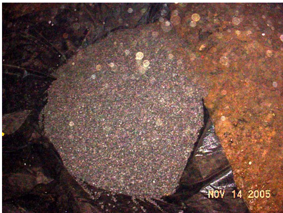
Photo 6 - Gravel being placed in excavation in 81 Broadway.
