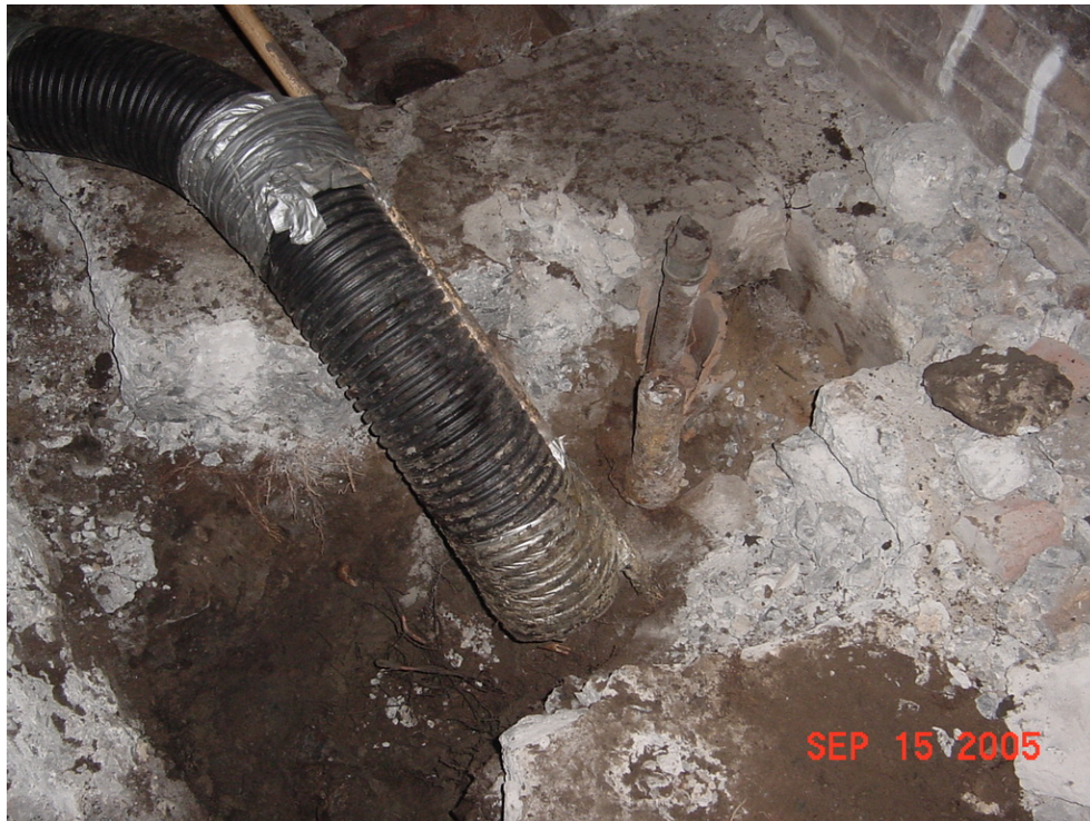
Photo 7 - Piping cut at concrete floor surface along eastern wall of 38 Post Street basement.
