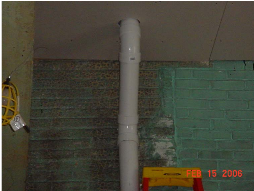
Photo 15 - SSD riser pipe exiting through roof of 81 Broadway. Need to insert picture of roof vent
