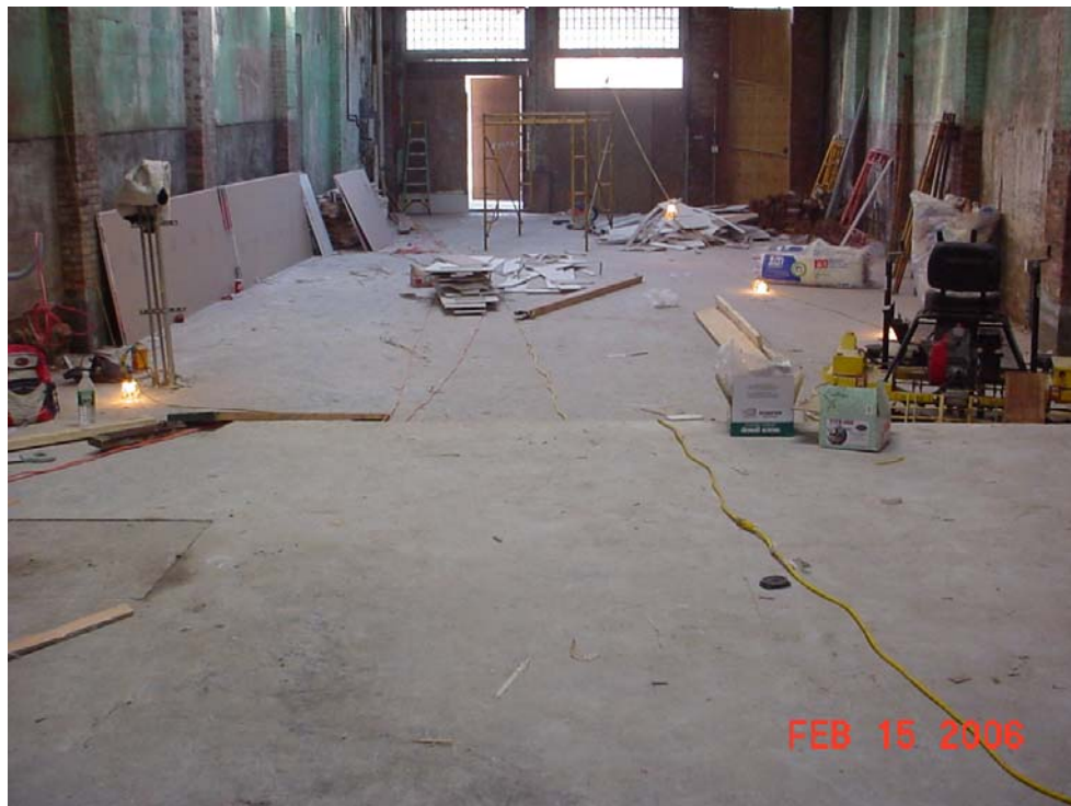
Photo 8 - Finished concrete floor over SSD piping system.
