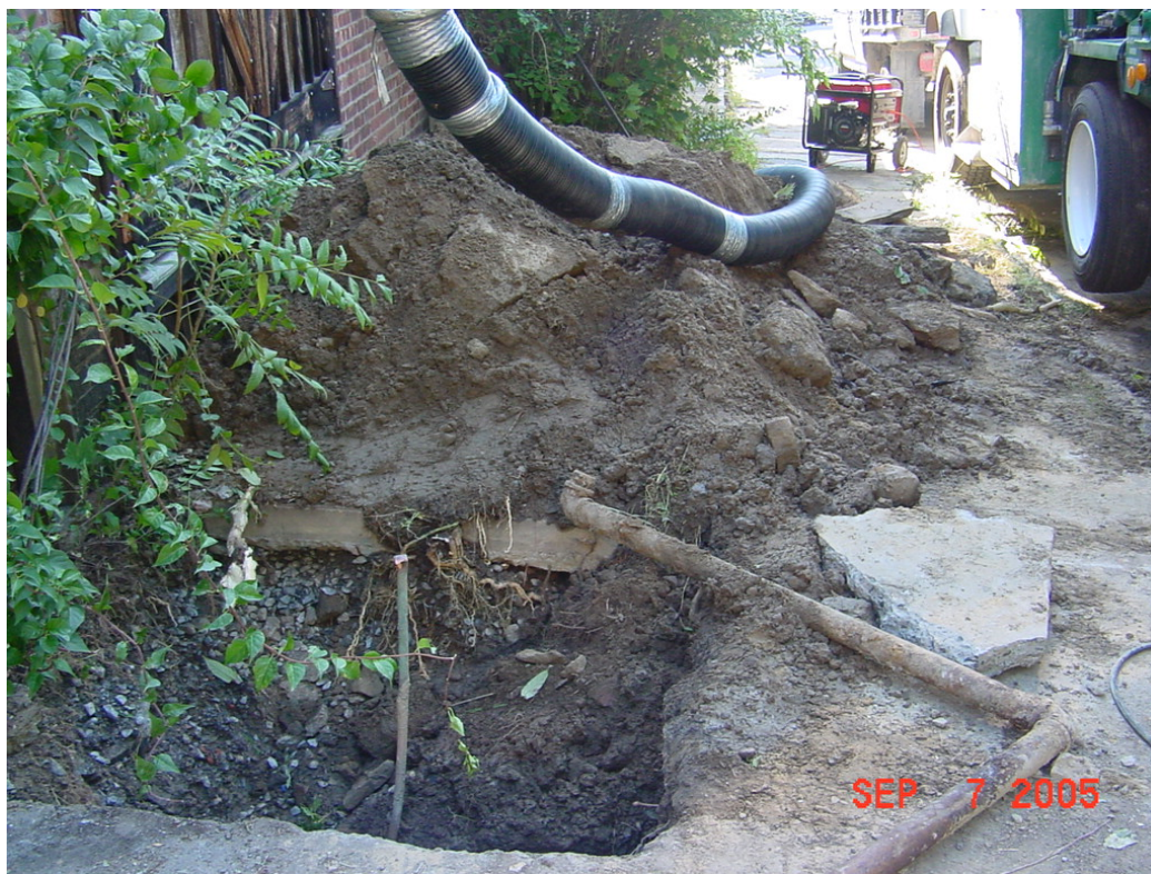
Photo 4 – Excavation area around 4,000-gallon UST in front of 38 Post Street showing broken water line pipe and broken UST vent pipe.
