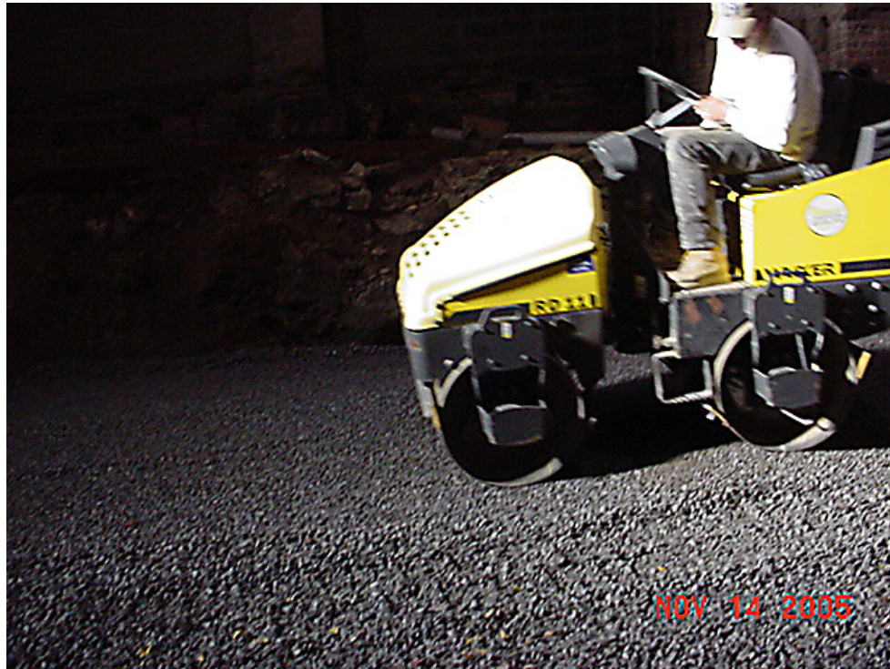
Photo 10 – Compaction of gravel inside excavation in 81 Broadway.
