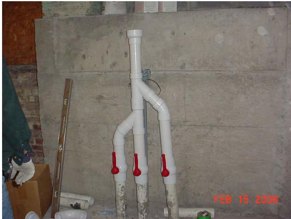
Photo 10 - SSD piping manifolded together.
