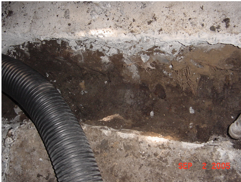
Photo 8 - Trench excavated across basement floor to pipes along eastern basement wall.
