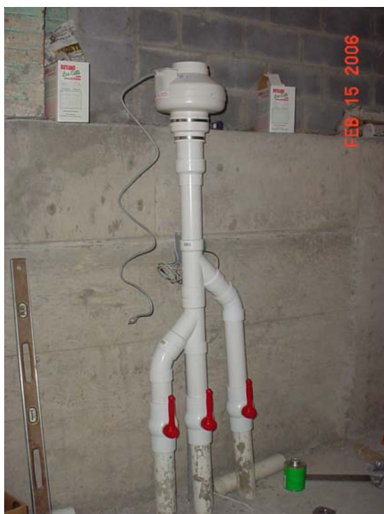
Photo 11 - SSD piping with depressurization fan.
