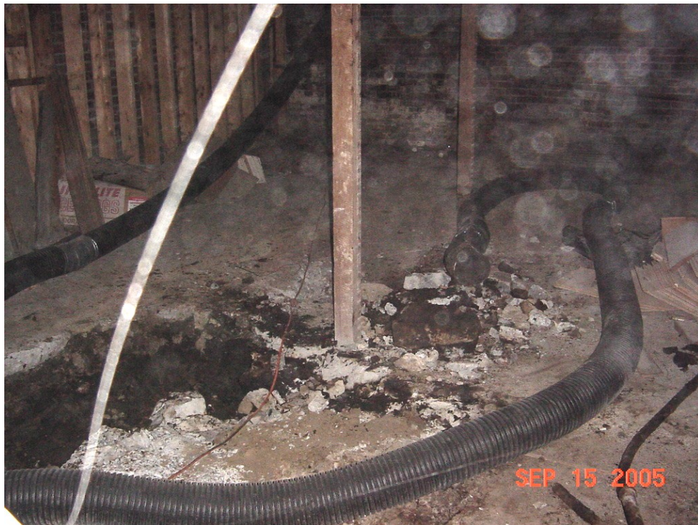
Photo 4 – Soil and concrete excavation in 38 Post Street basement.
