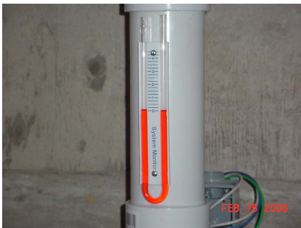
Photo 12 - Visual manometer used to demonstrate fan operation; fan is off.
