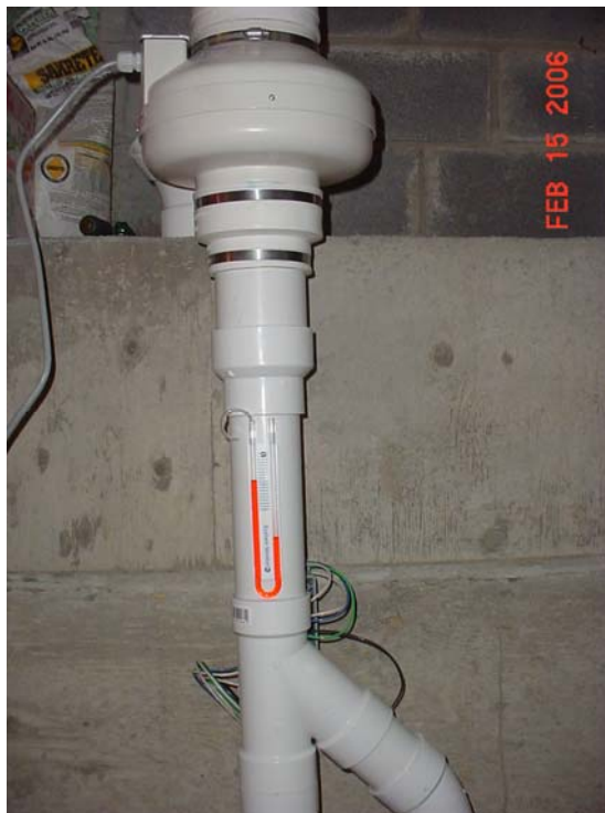
Photo 17 - Visual manometer demonstrating vacuum pressure with fan operating.
