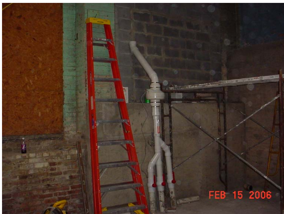
Photo 13 - Riser angled to wall for extension up through roof.
