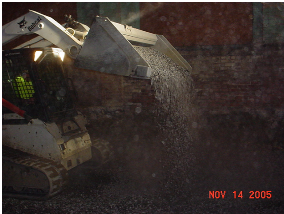
Photo 7 - Gravel being emplaced in excavation inside 81 Broadway.
