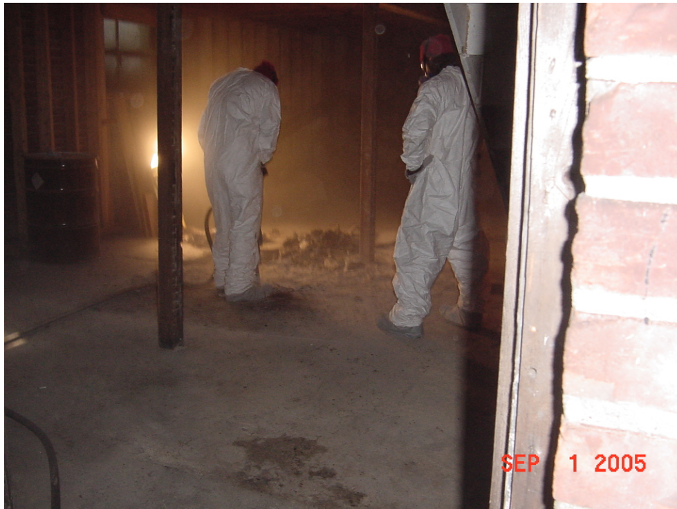
Photo 2 - Concrete and soil removal in 38 Post Street basement.
