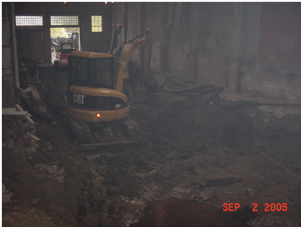
Photo 4 – Soil removal activities at 81 Broadway with dump trucks being loaded through door in background.
