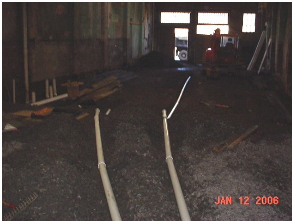
Photo2 - View northward of sub-slab depressurization system piping inside 81 Broadway.
