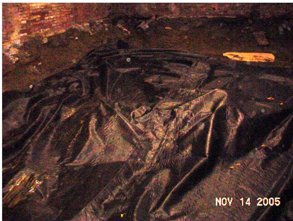
Photo 5 - Geotextile laid in base of excavation in 81 Broadway prior to backfilling with gravel.
