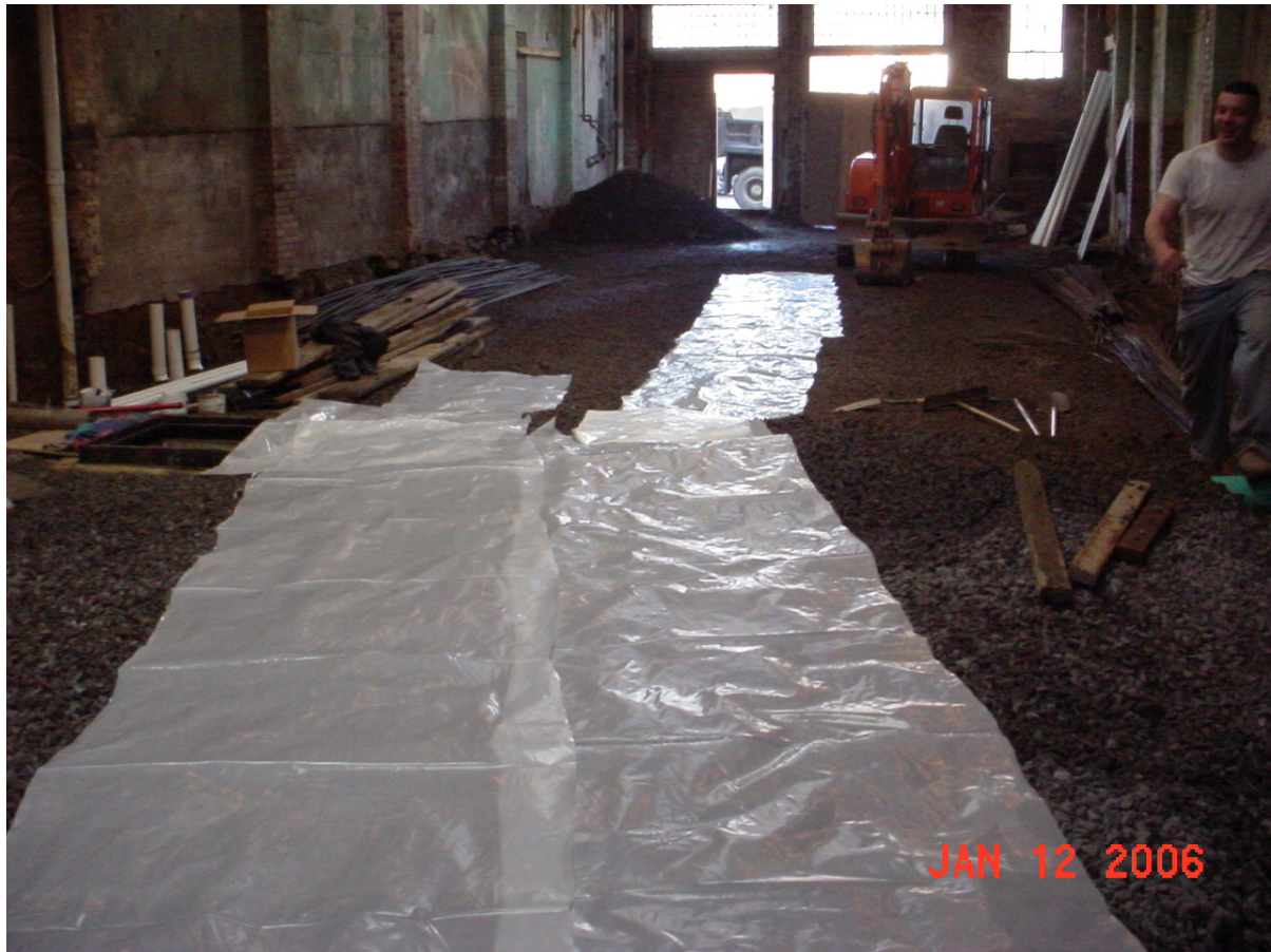
Plastic sheeting being installed over sub slab aggregate.
