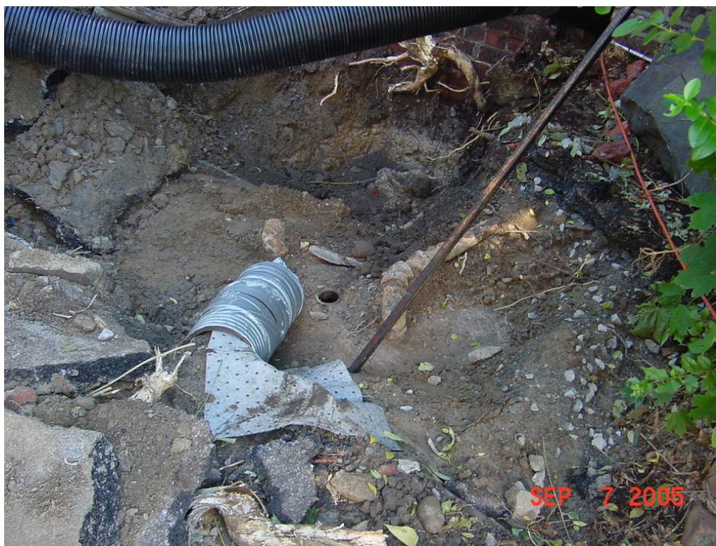
Photo 3 – Top of eastern portion of 4,000-gallon UST showing vent pipe.
