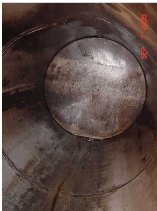
Photo 5 - Inside of cleaned 1,500 gallon UST.
