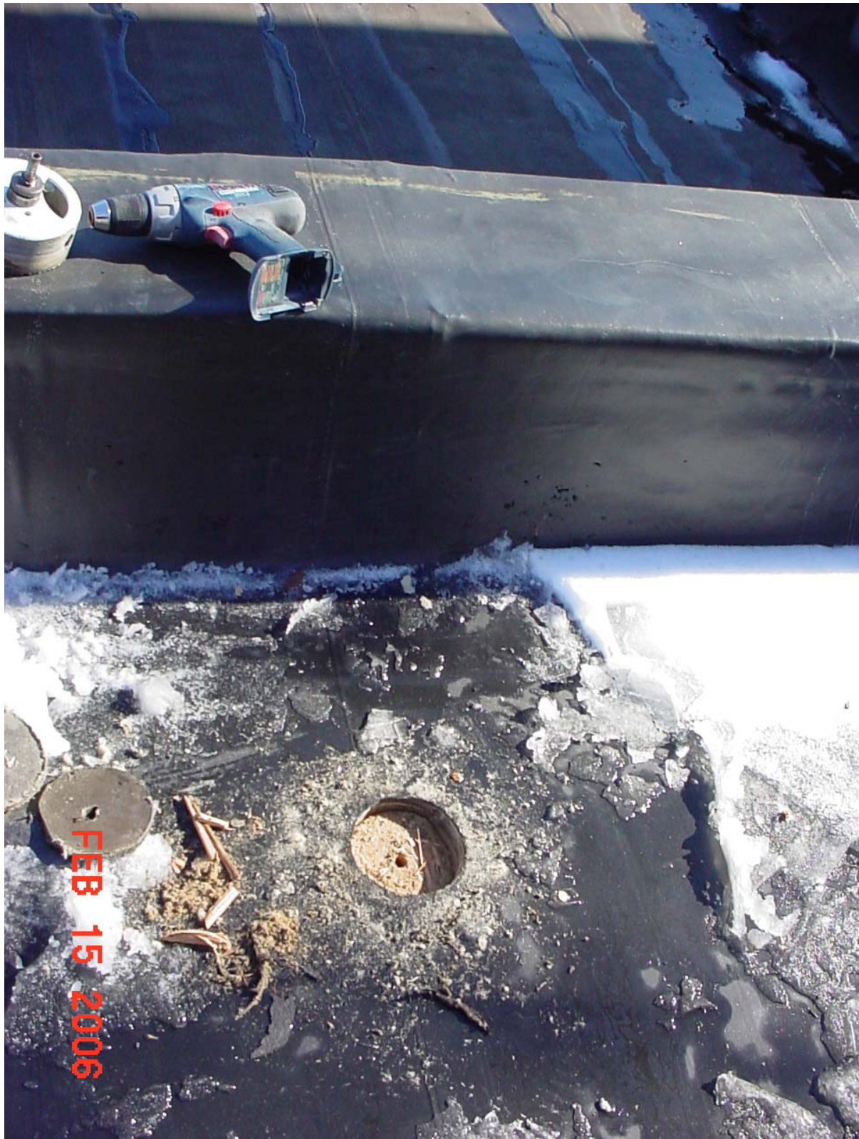
Roof penetration for manifolded exhaust stack.
