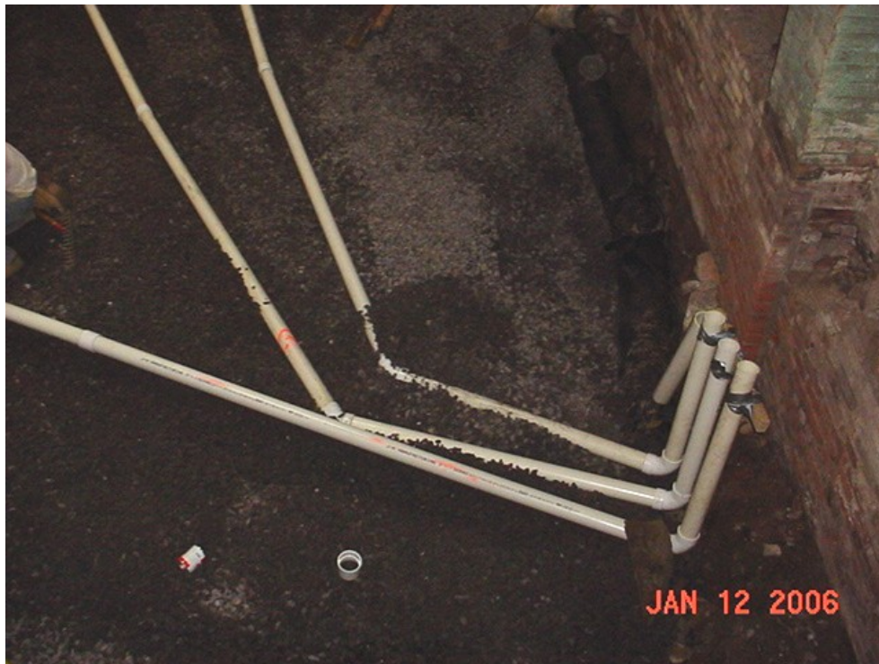
Photo 3 - Installation of 81 Broadway sub-slab depressurization system piping.
