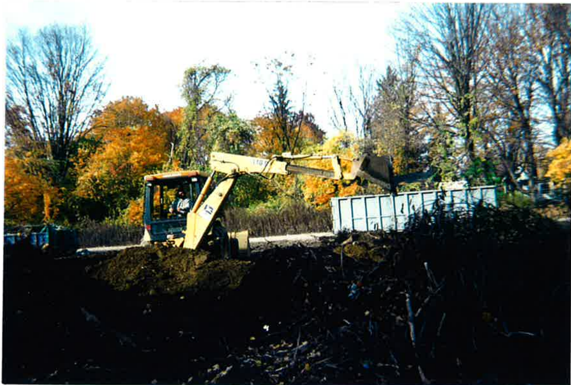
Below: Site Clearing.
