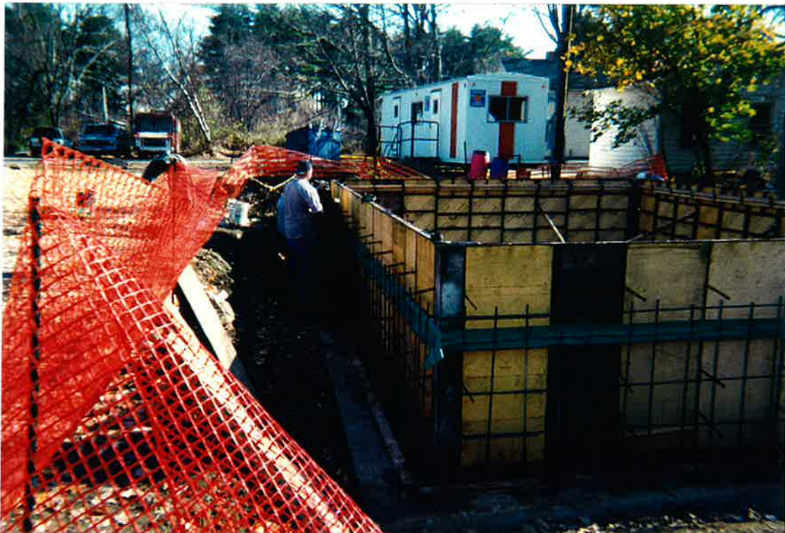
Below: Form Setup for Treatment Building Footer Wall.
