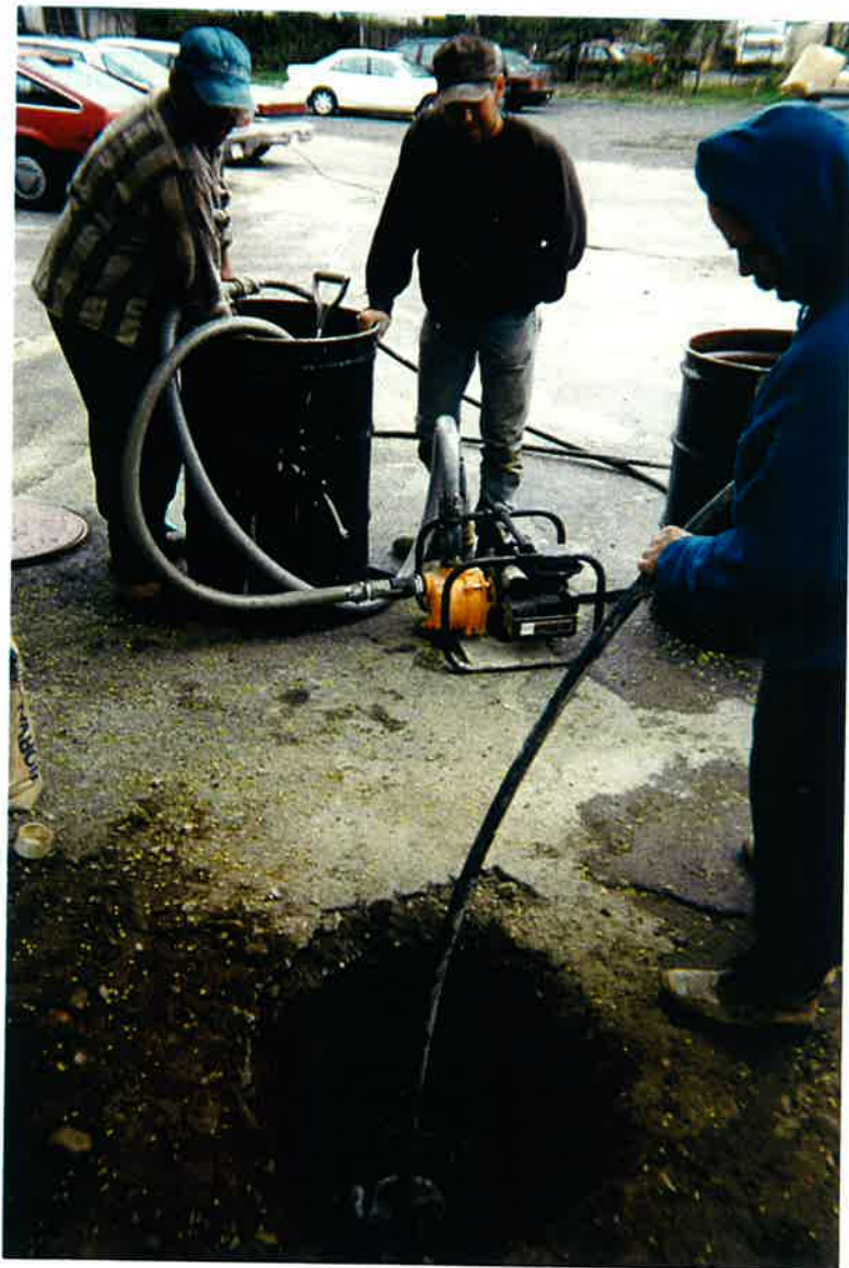
Installation of Electrical and Control Wiring, Pump and Sensor at EW-3.
