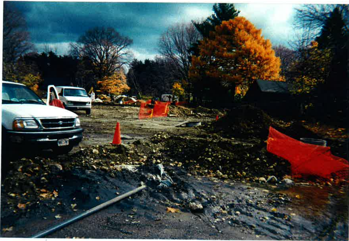
Above: Overview of Site During Construction Activities.
