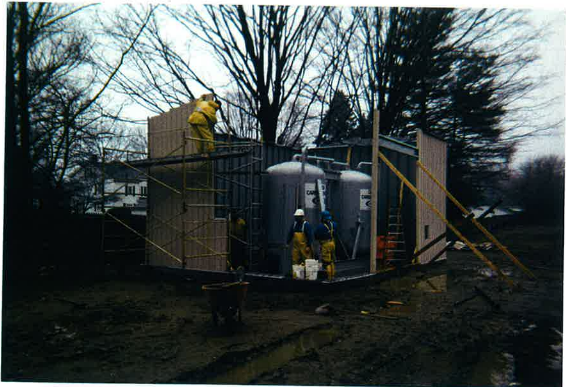
Below: Treatment Building Construction.
