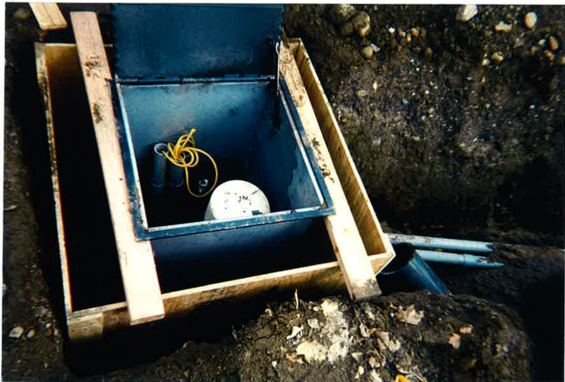
Below: EW-1 Vault Installation.
