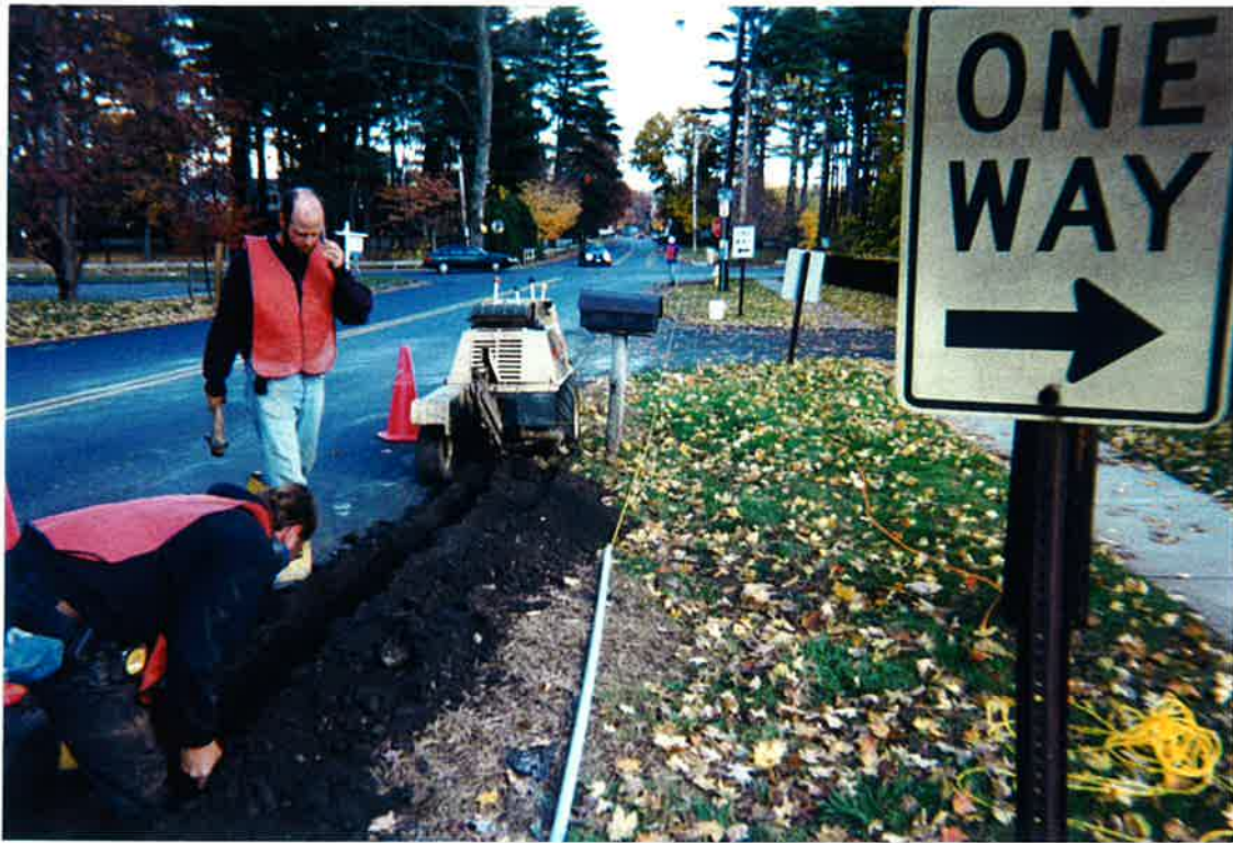
Above: Conduit Installation Along Bedford Road.
