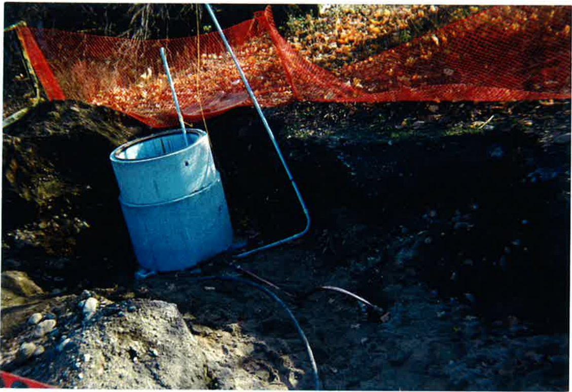
Above: Water Connection from Water Main to Manhole.
