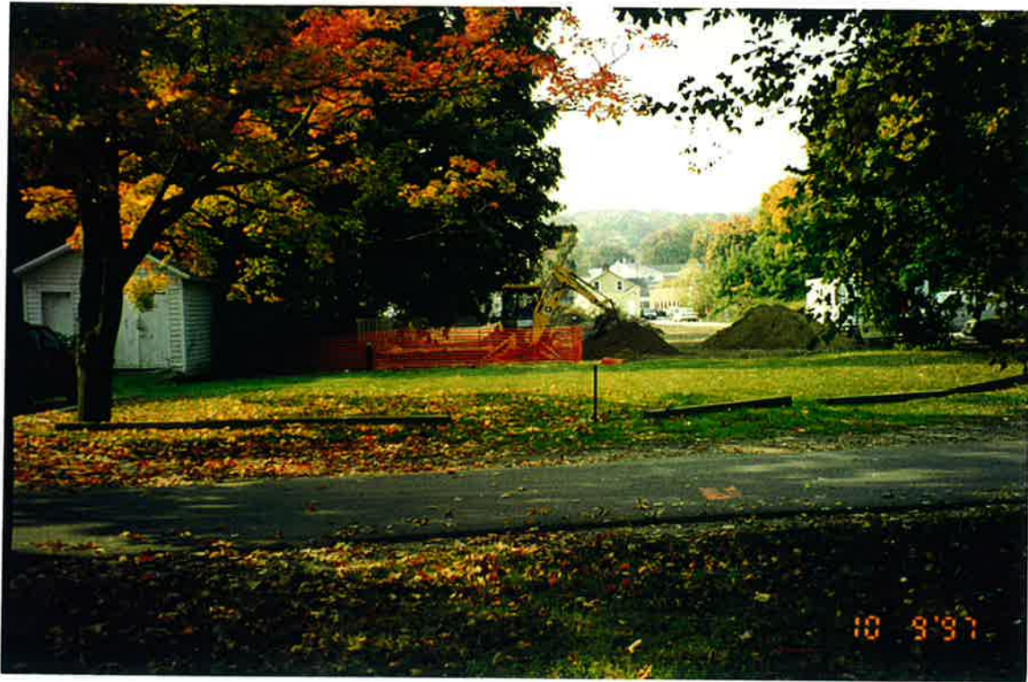
Above: Treatment Building Foundation Excavation.
