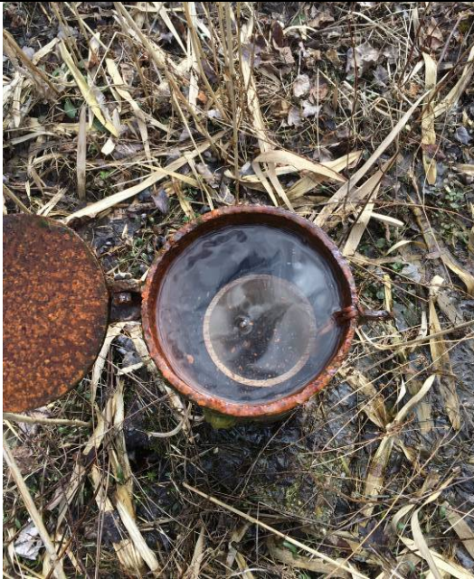
Photo 3: Photo of BVWSA-MW-6B, well overflowing with groundwater
