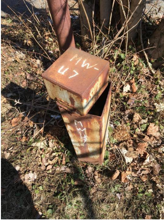
Photo 1: Photo of BVWSA-MW-U7 with damaged casing cap
