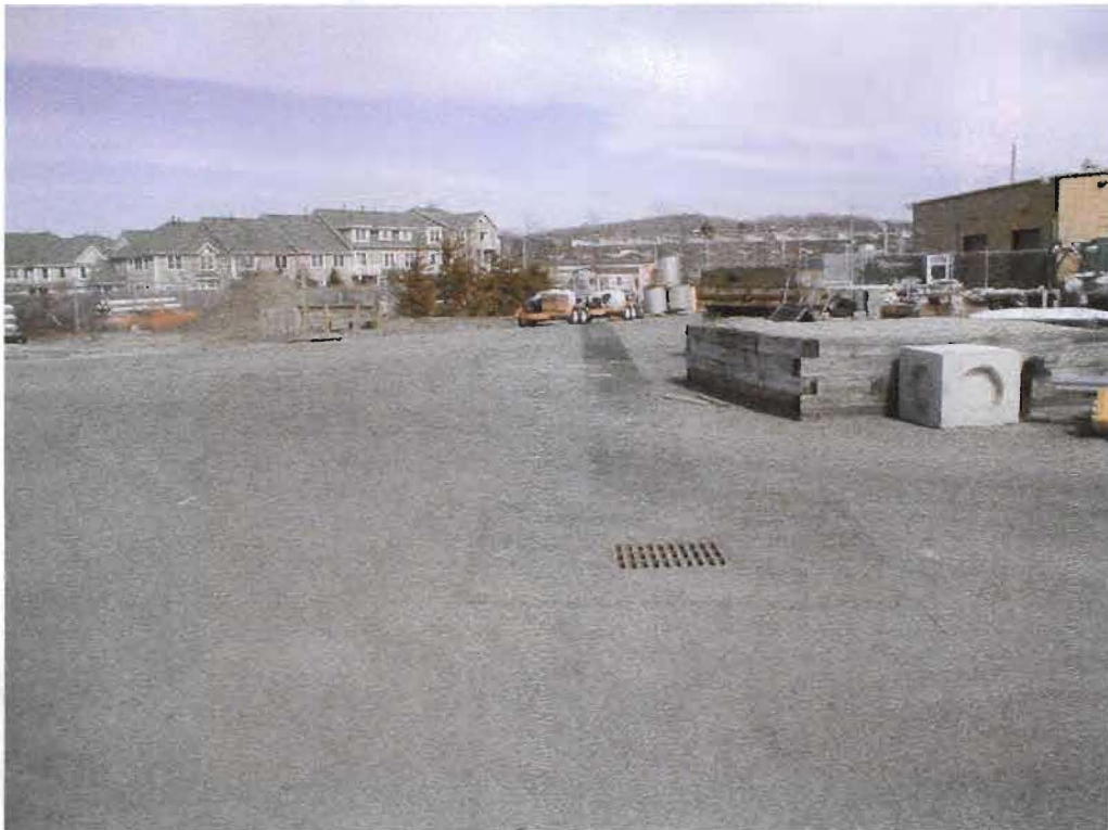
Location 4 View of the sump box installed during drainage modification system.
