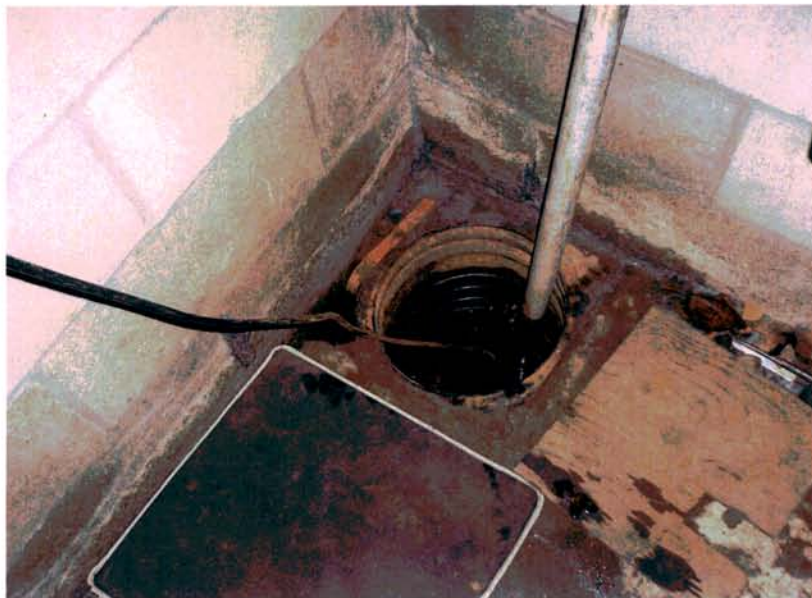
Figure 2. Sample 1 is a liquid sample collected from a sump in the basement of a residence adjacent to the landfill. Sample 2 consisted of solids (iron floc) removed from the sump.
